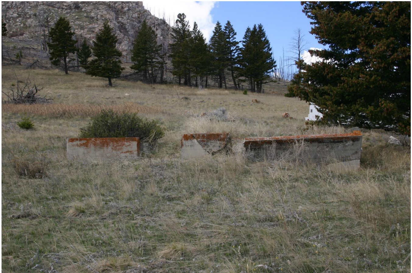
MT_BroadwaterCounty_SpokaneHillAirwayBeacon_#0008: Generator shed foundation. View to the west.
