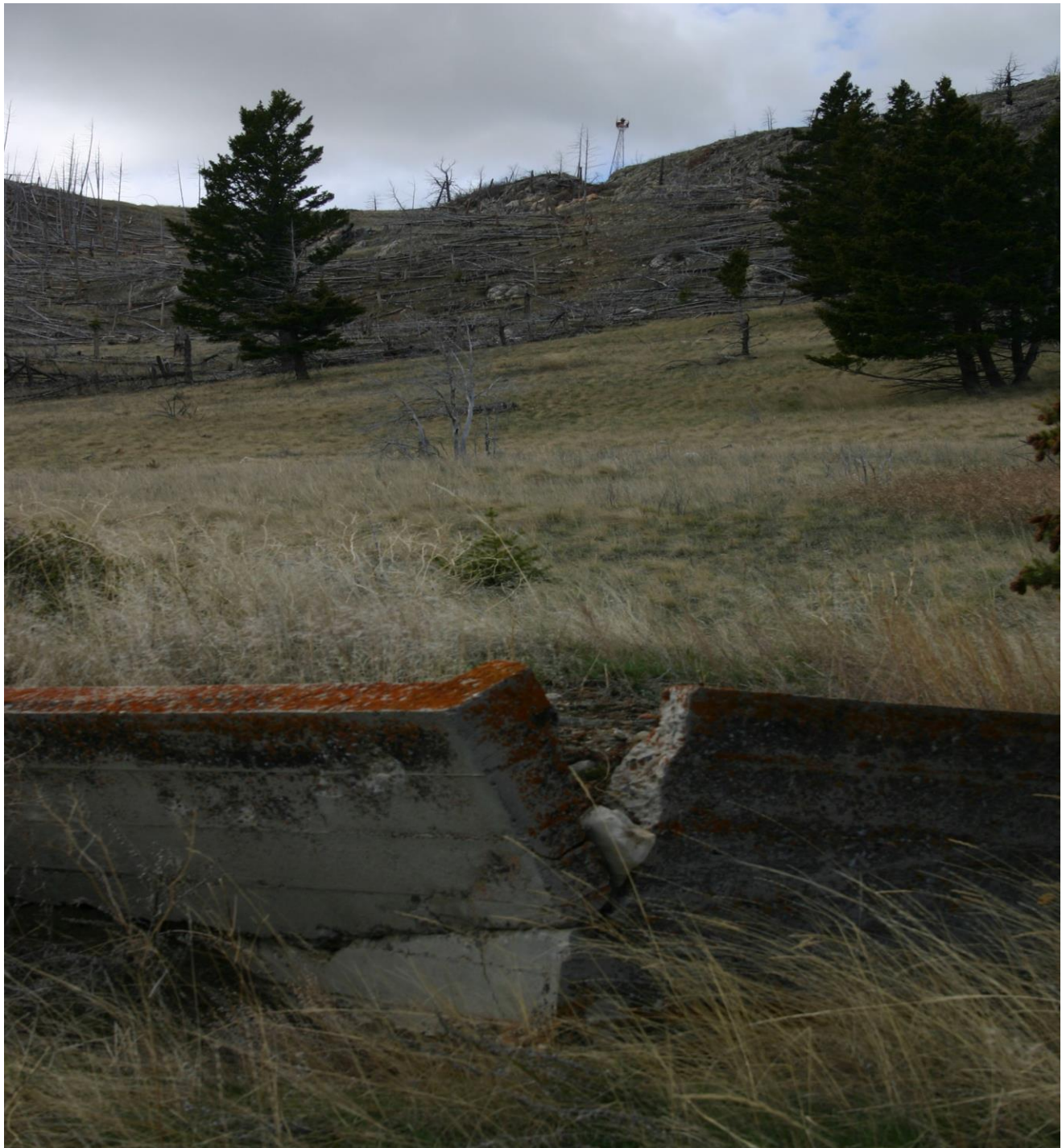
MT_BroadwaterCounty_SpokaneHillAirwayBeacon_#0001: View to the south-southwest.
