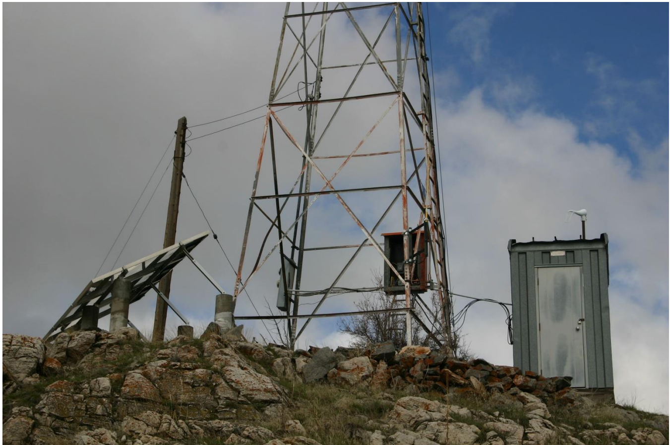
MT_BroadwaterCounty_SpokaneHillAirwayBeacon_#0005: Detail of tower base and shed. View to northwest.
