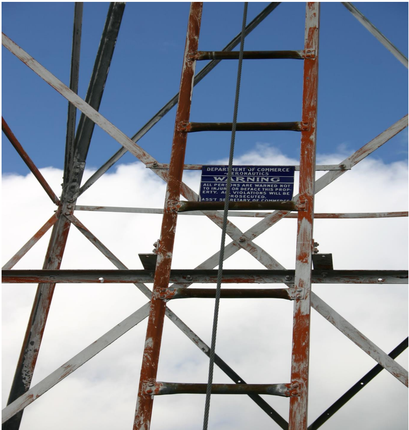
MT_BroadwaterCounty_SpokaneHillAirwayBeacon_#0006: Detail of warning sign. View to the south-southwest.
