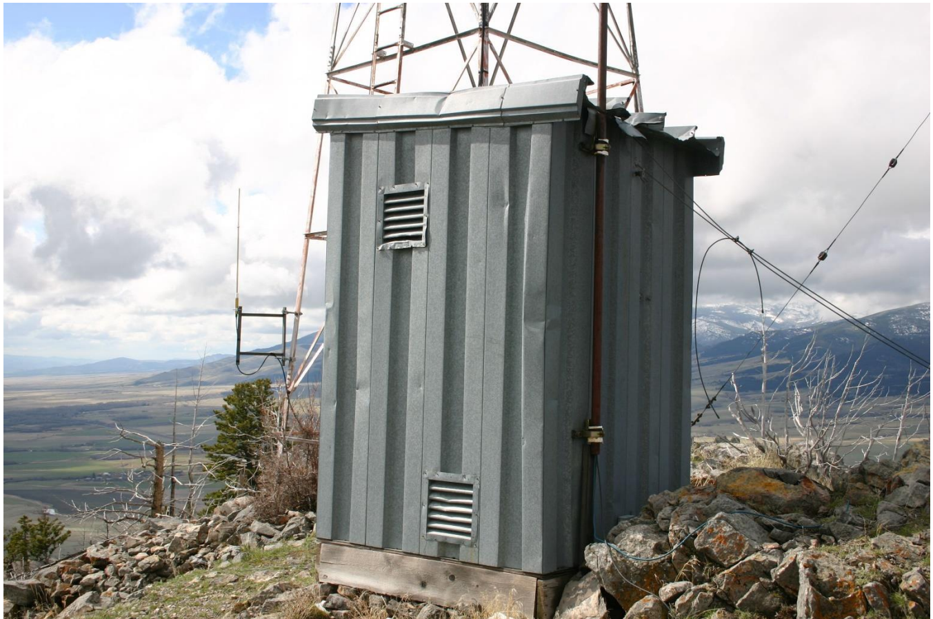
MT_BroadwaterCounty_SpokaneHillBeacon_#0007: Shed. View to the south.
