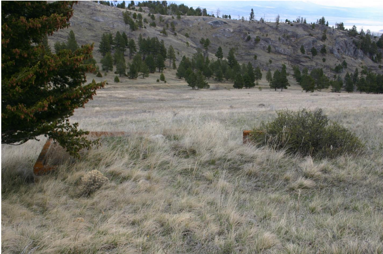
MT_BroadwaterCounty_SpokaneHillAirwayBeacon_#0009: Generator shed foundation. View to the east.
