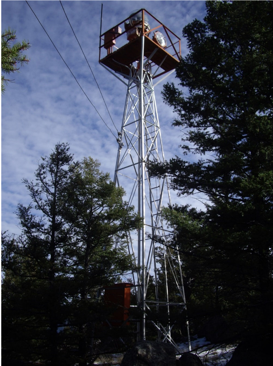
MT_JeffersonCounty_WhitetailAirwayBeacon_#0005: View to Northeast.
