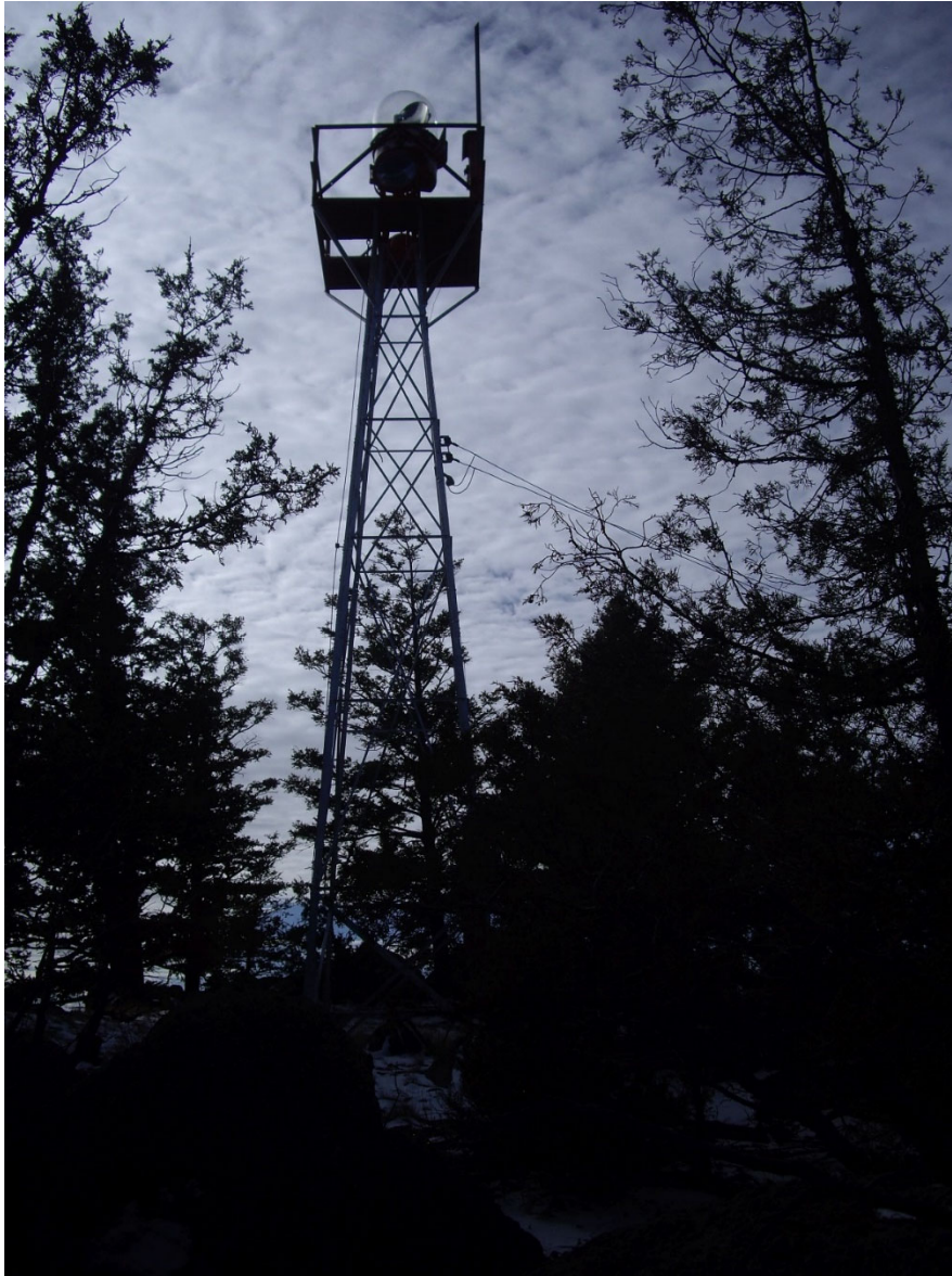
MT_JeffersonCounty_WhitetailAirwayBeacon_#0003: View to the South.
