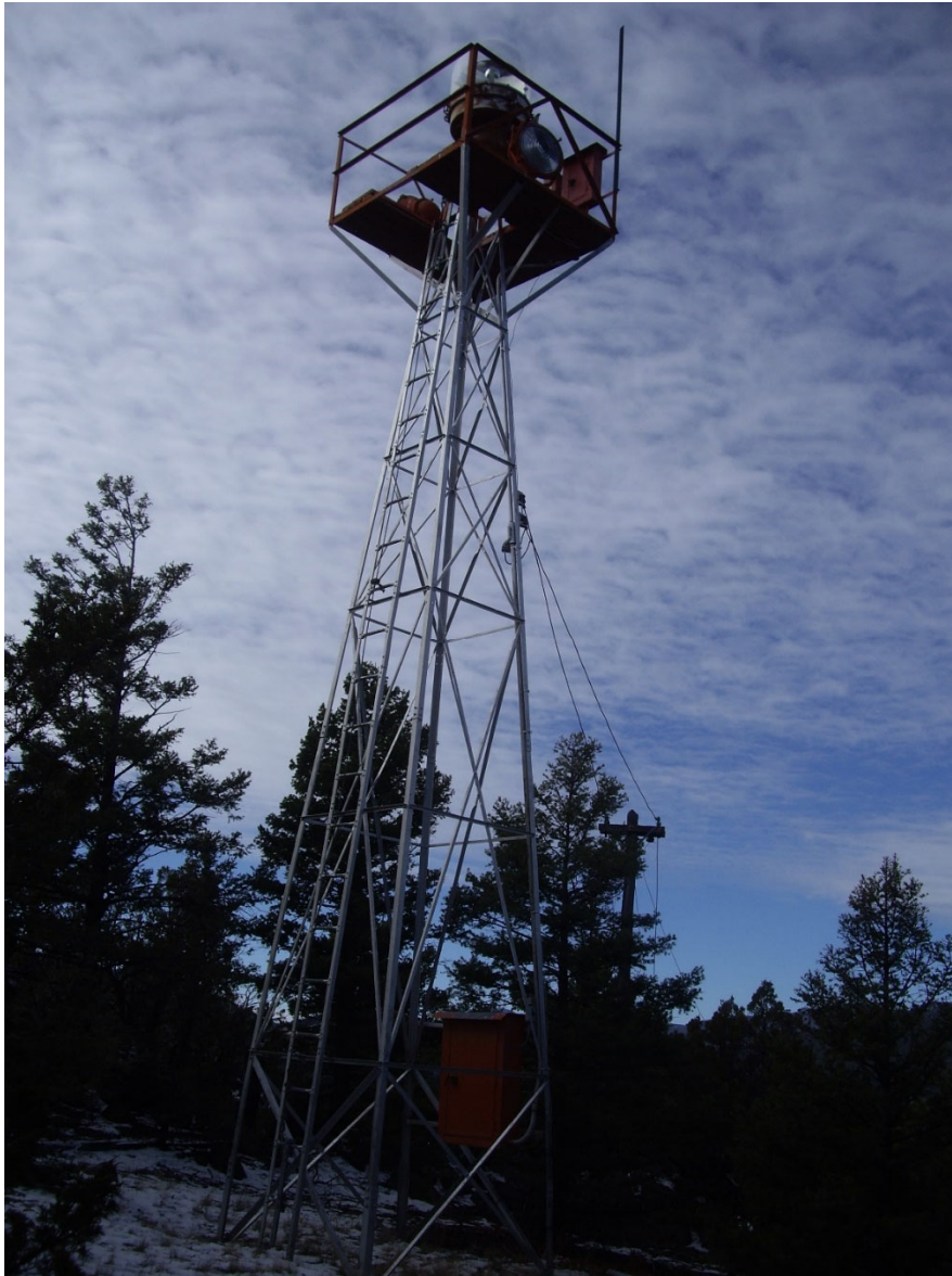
MT_JeffersonCounty_WhitetailAirwayBeacon_#0002: View to the South-southwest.
