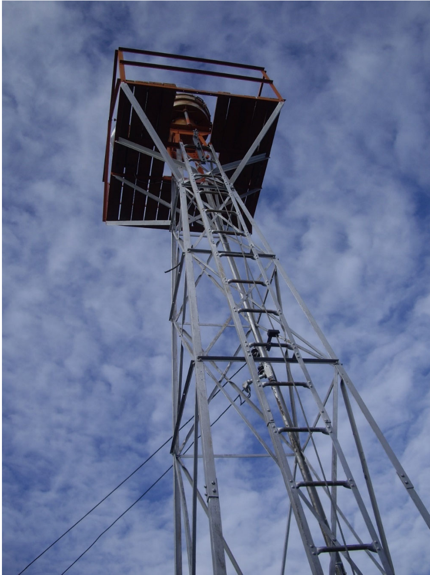
MT_JeffersonCounty_WhitetailAirwayBeacon_#0004: View to the West-southwest.
