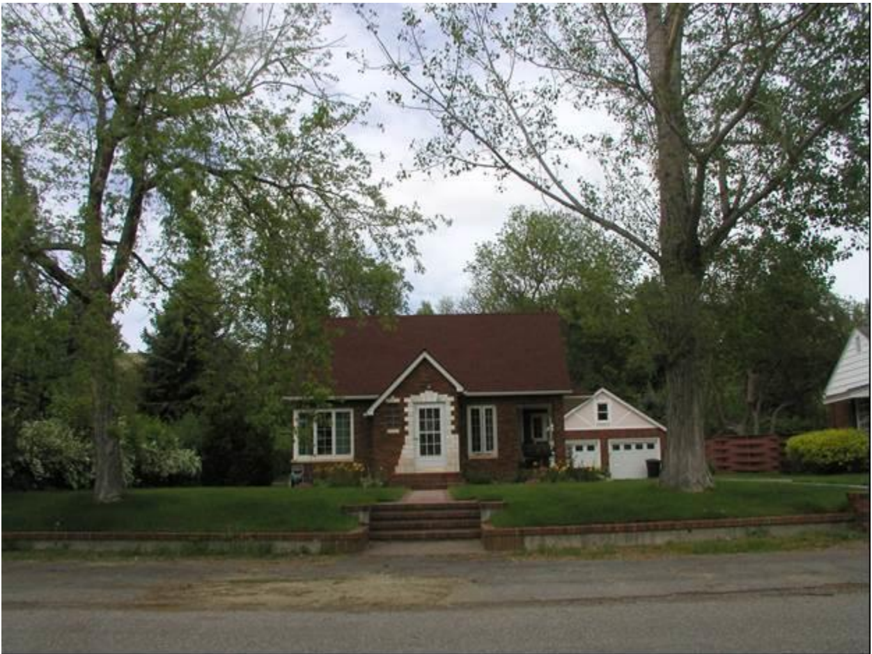
Description and view of camera: South elevation from street, view to north. Photograph: MT_YellowstoneCounty_ArnoldGrafHouse_0001
