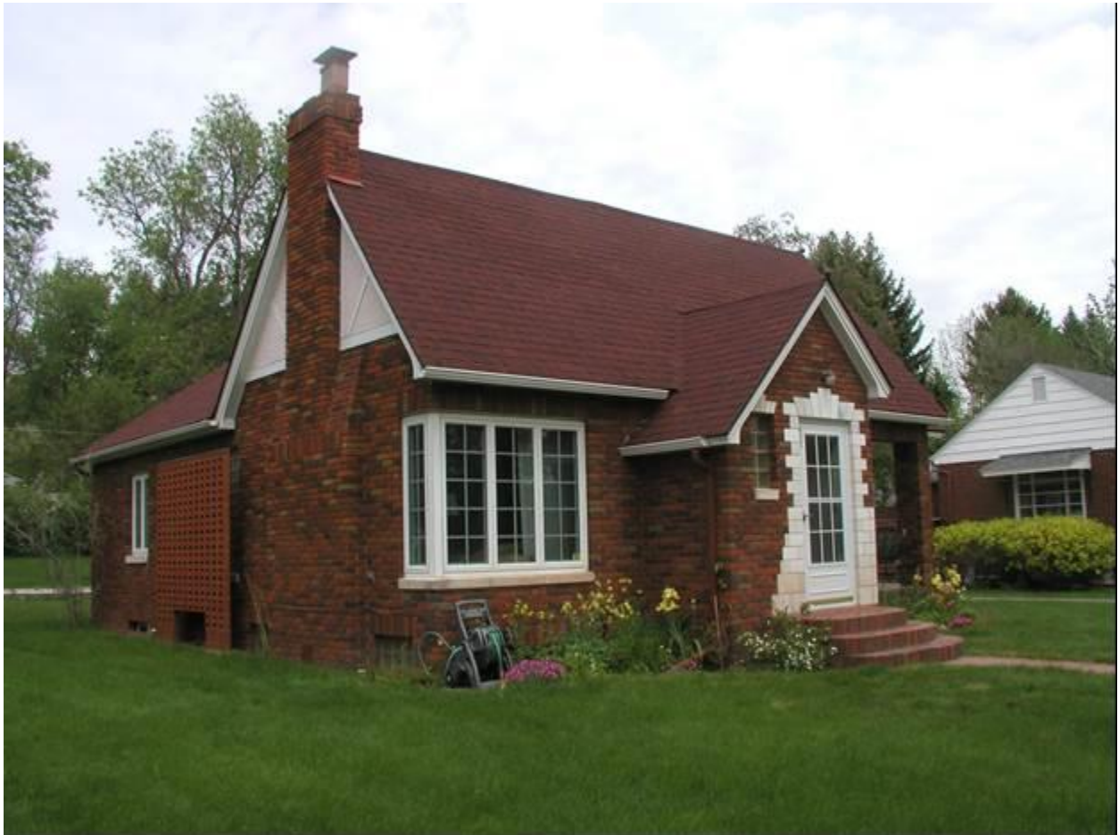
Description and view of camera: South and west elevations, view to northeast. Photograph: MT_YellowstoneCounty_ArnoldGrafHouse_0002
