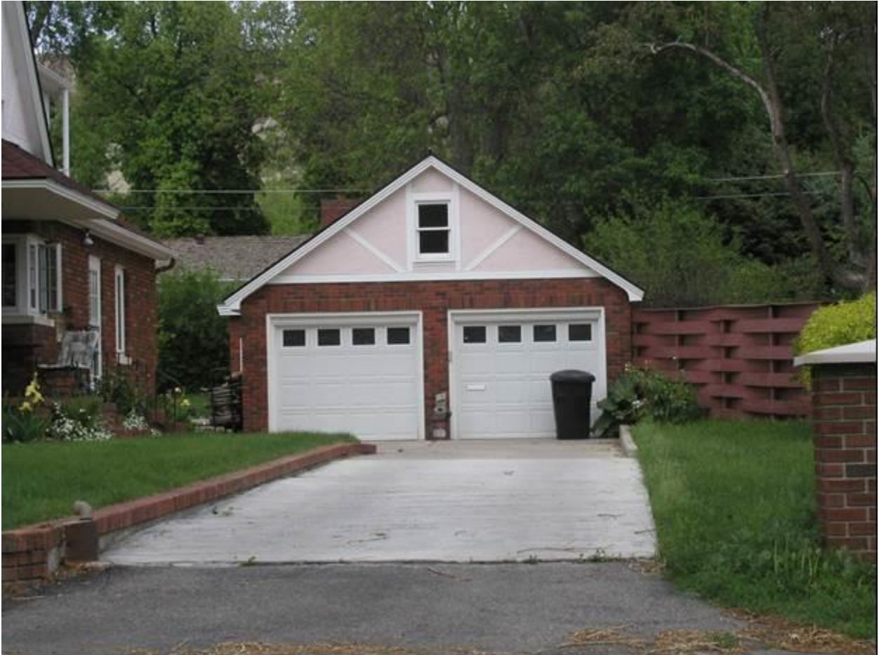
Description and view of camera: South elevation, Garage, view to north Photograph: MT_YellowstoneCounty_ArnoldGrafHouse_0008
