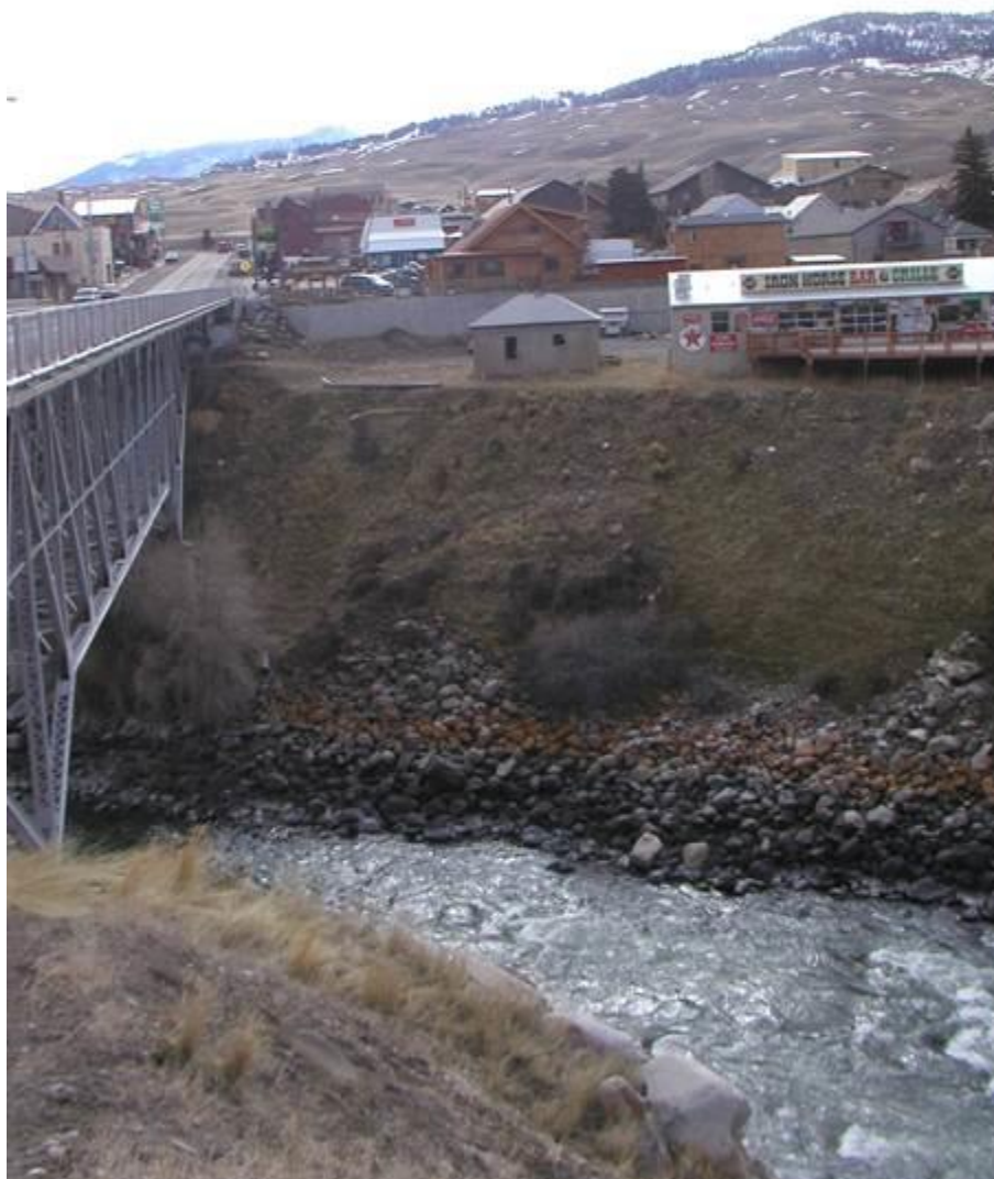
Description and view of camera: North elevation, view to south across Yellowstone River Photograph: MT_ParkCounty_GardinerJail_0005
