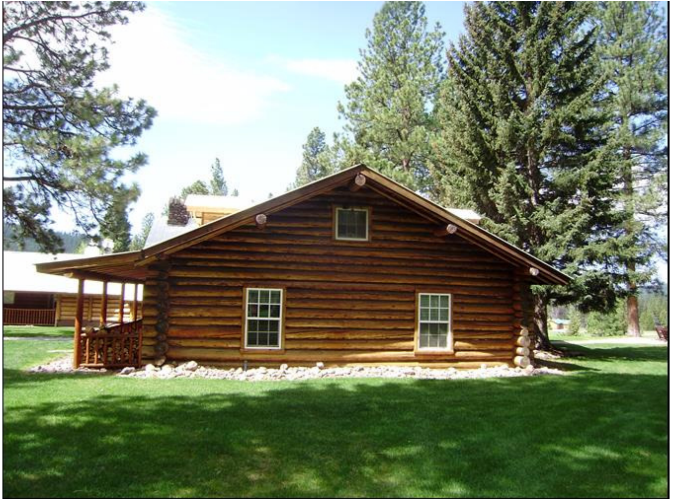
Photo 0006. East elevation of lodge. View to west.
