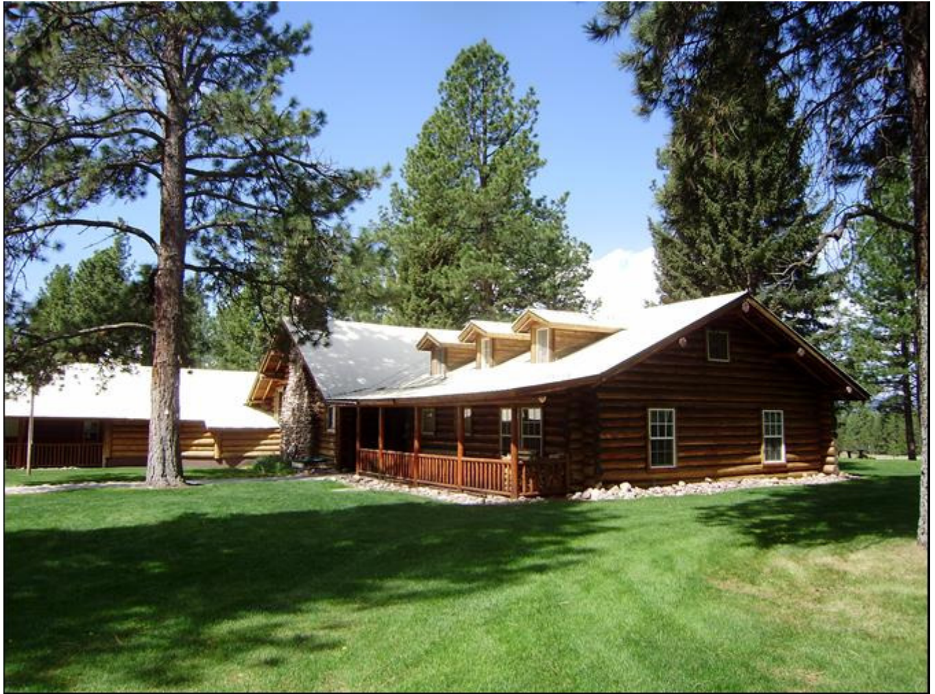
Photo 0003. Façade and east elevation. View to the west.
