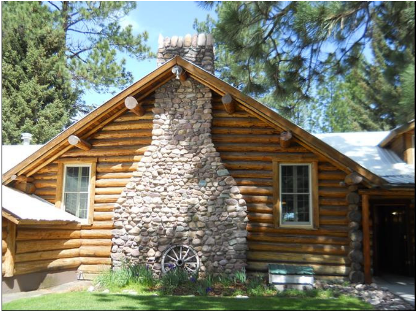
Photo 0004. Detail of cobblestone chimney. View to north.
