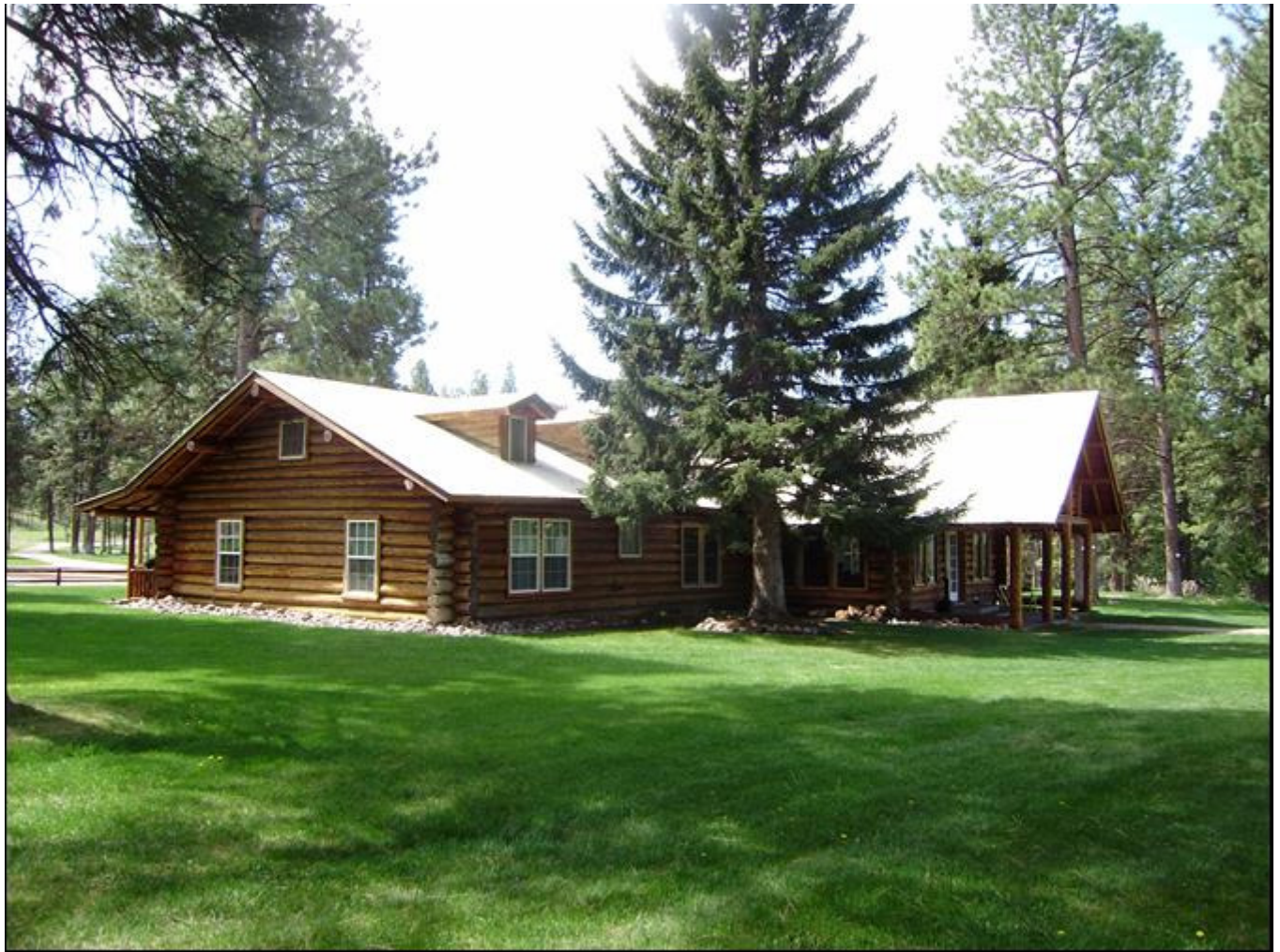
Photo 0007. East elevation and north side of lodge. View to southwest.
