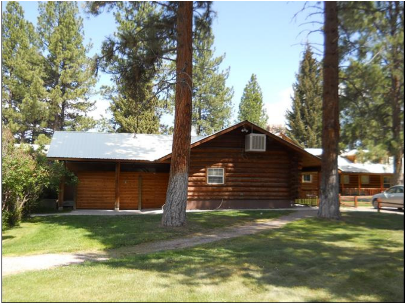
Photo 0014. South side of 2002 addition. View to north.
