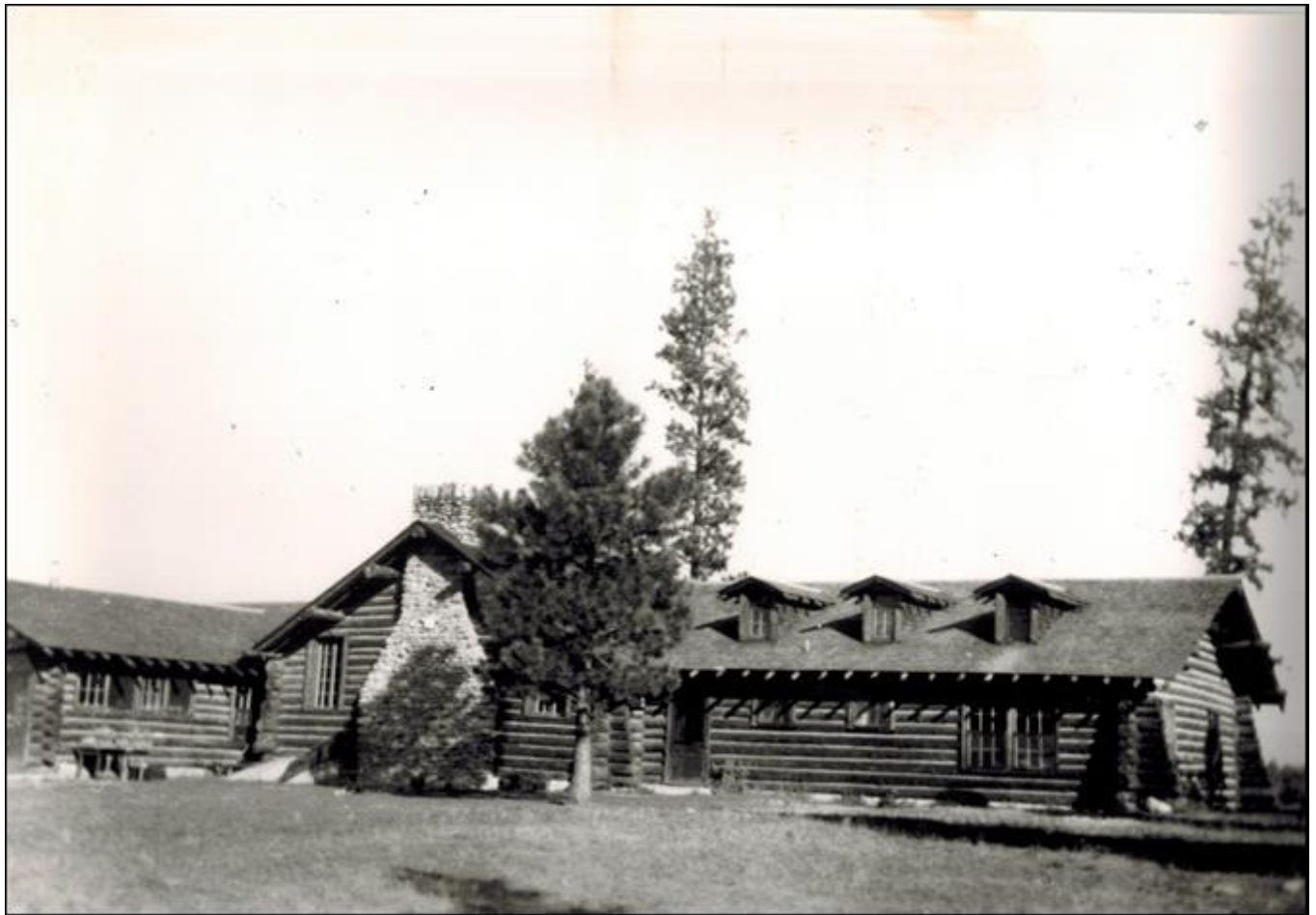
Double Arrow Lodge, circa 1930. View to northwest.
