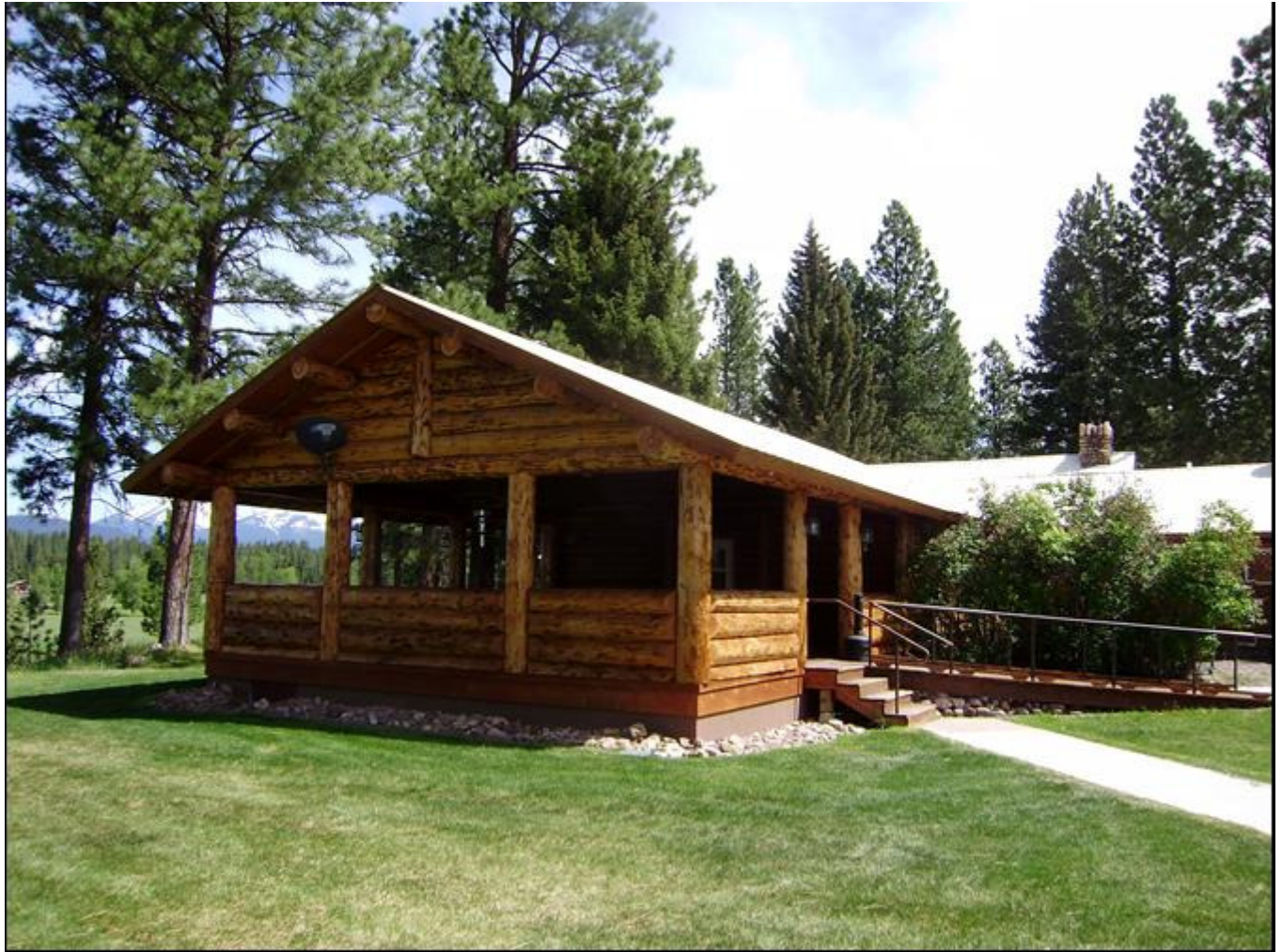
Photo 0013. Patio on west wing. View to northeast.
