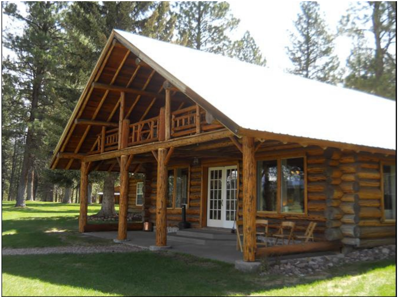
Photo 0011. North patio and balcony. View to the southeast.
