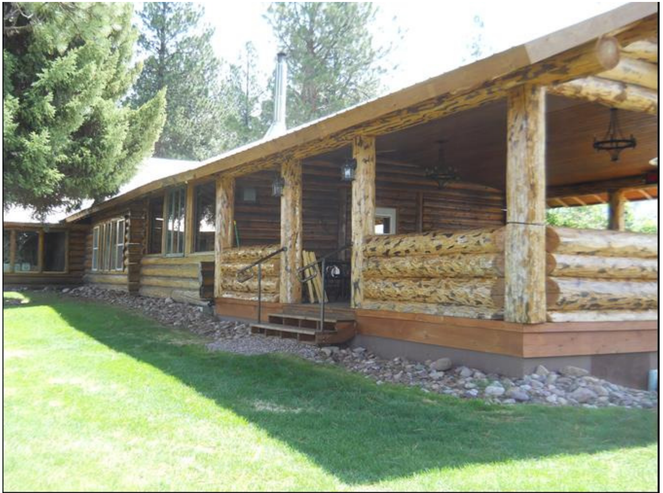
Photo 0012. North side of west wing. View to east.
