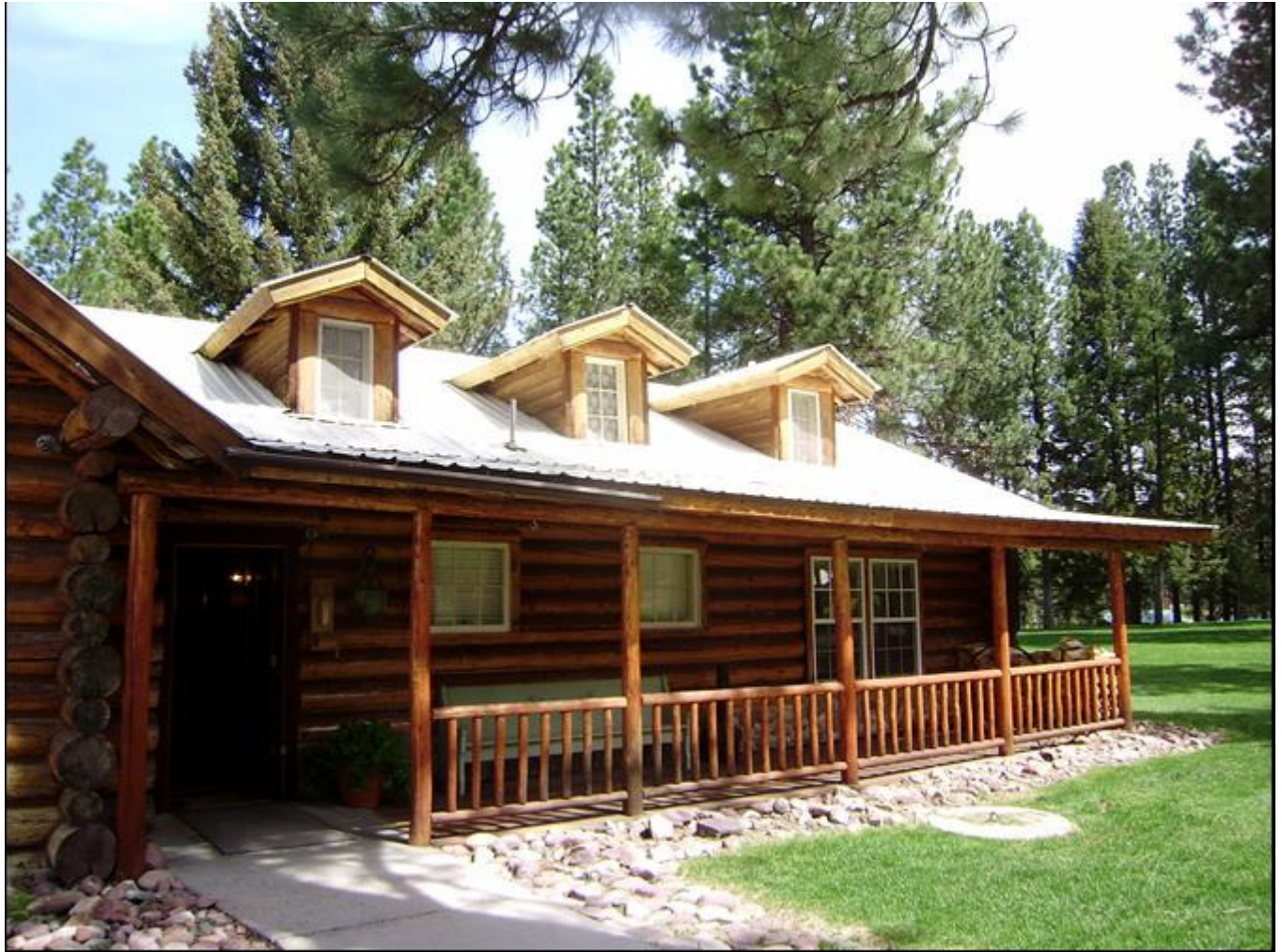
Photo 0005. Façade of lodge's east wing. View to northeast.
