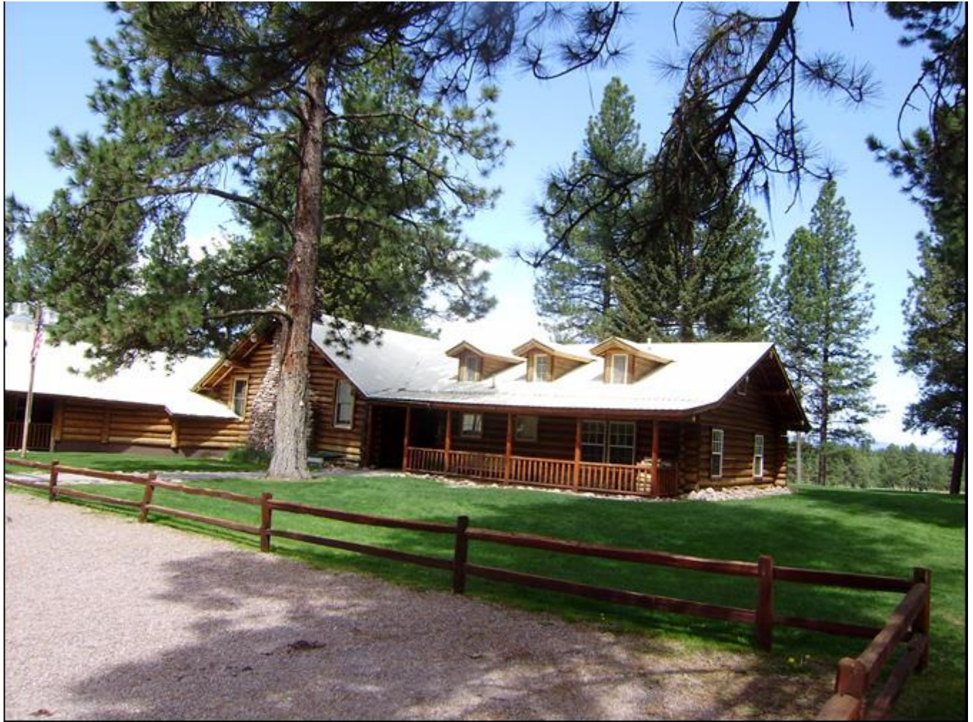
Photo 0001. Overview of façade of Double Arrow Lodge. View to northwest.
