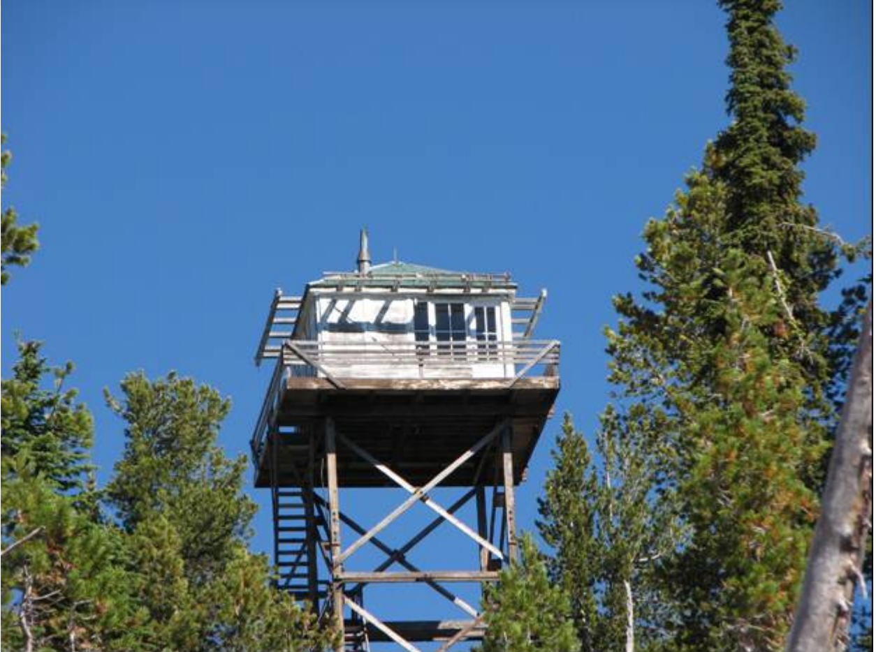
MT_MissoulaCounty_MineralPeakLookout_0001. Looking north to the south side of Mineral Peak Lookout.
