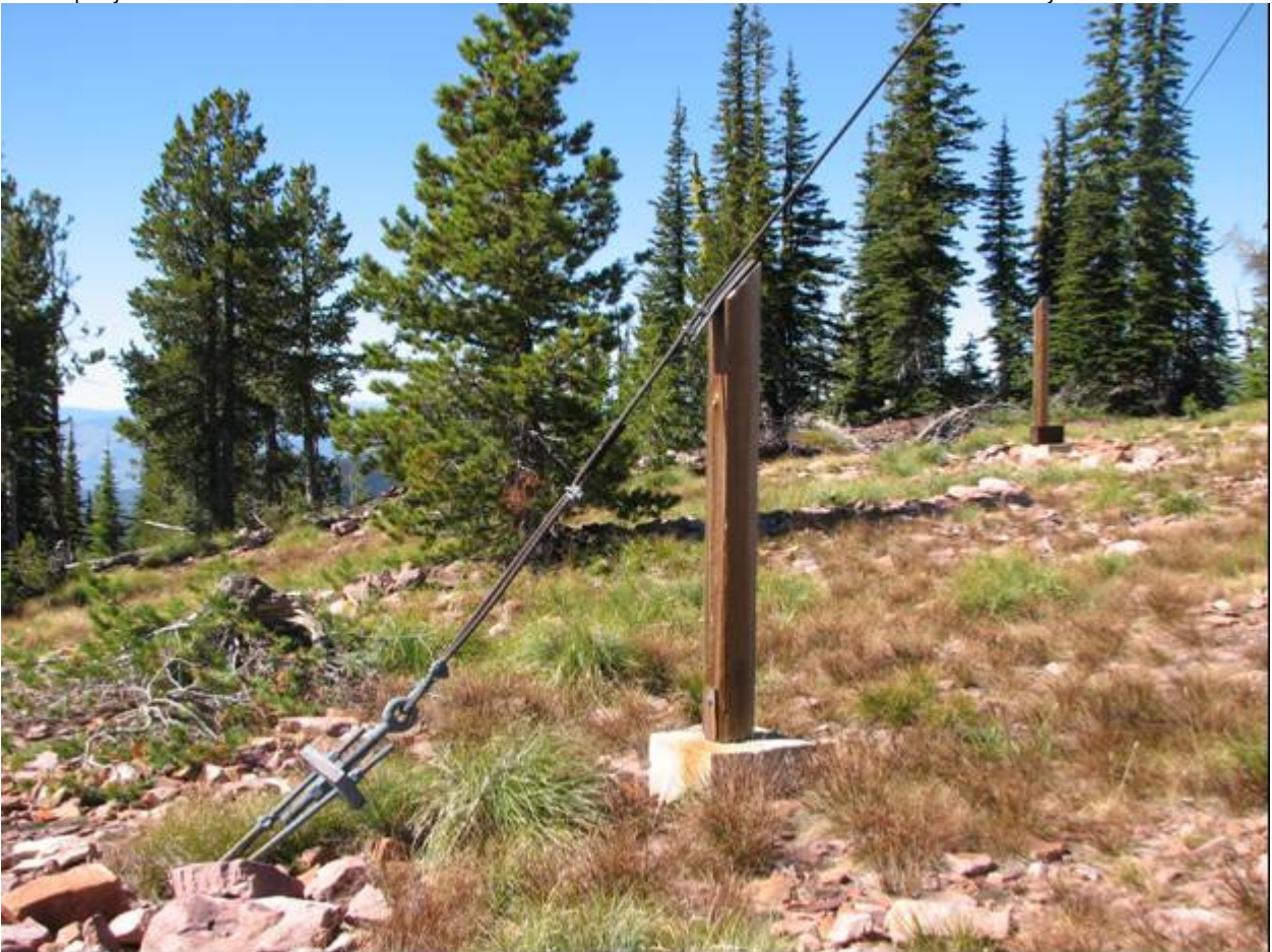
MT_MissoulaCounty_MineralPeakLookout_0007. Detail of guy wire anchors.
