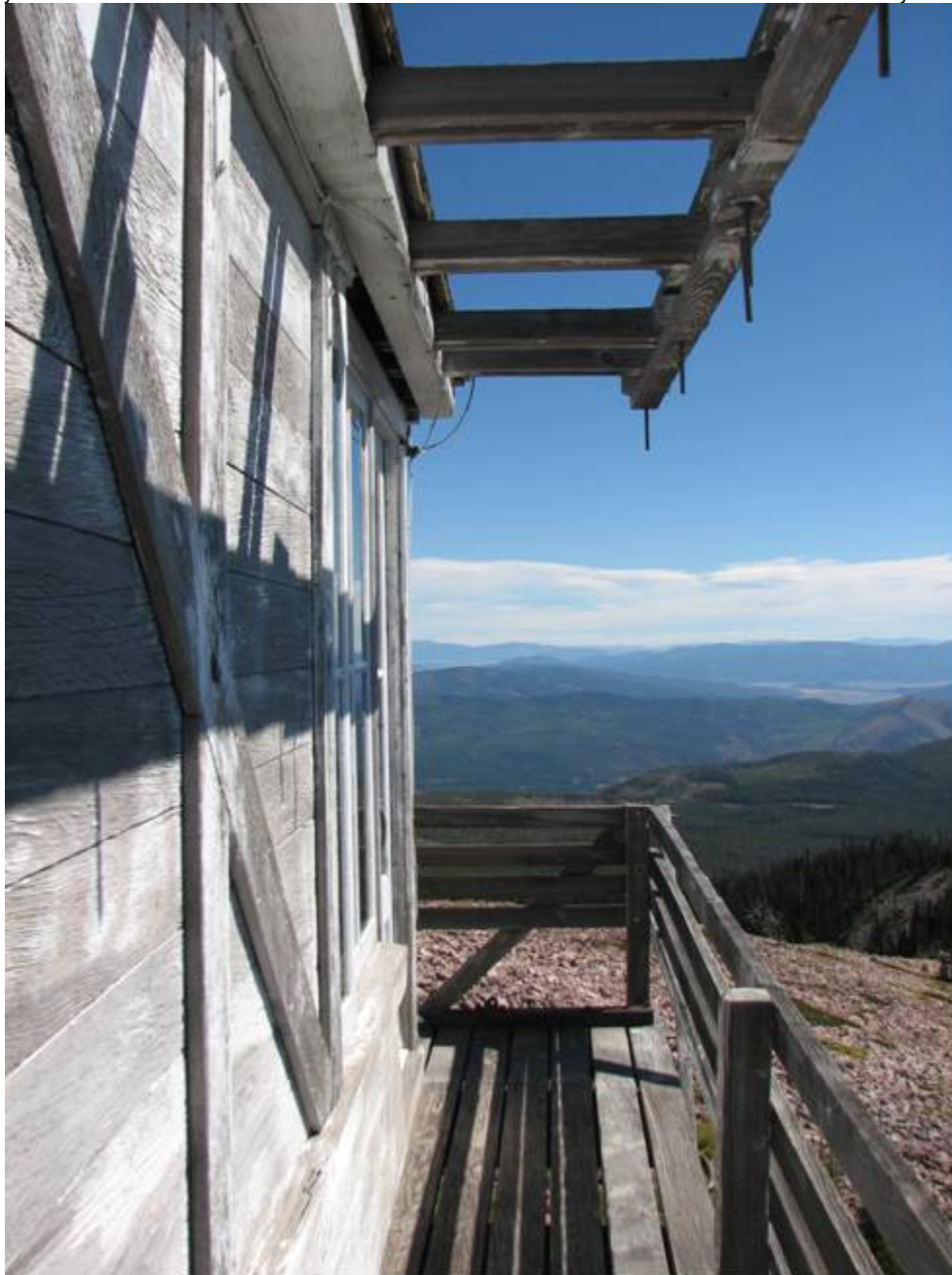
MT_MissoulaCounty_MineralPeakLookout_0004. Looking east along the front (south) wall of the lookout.
