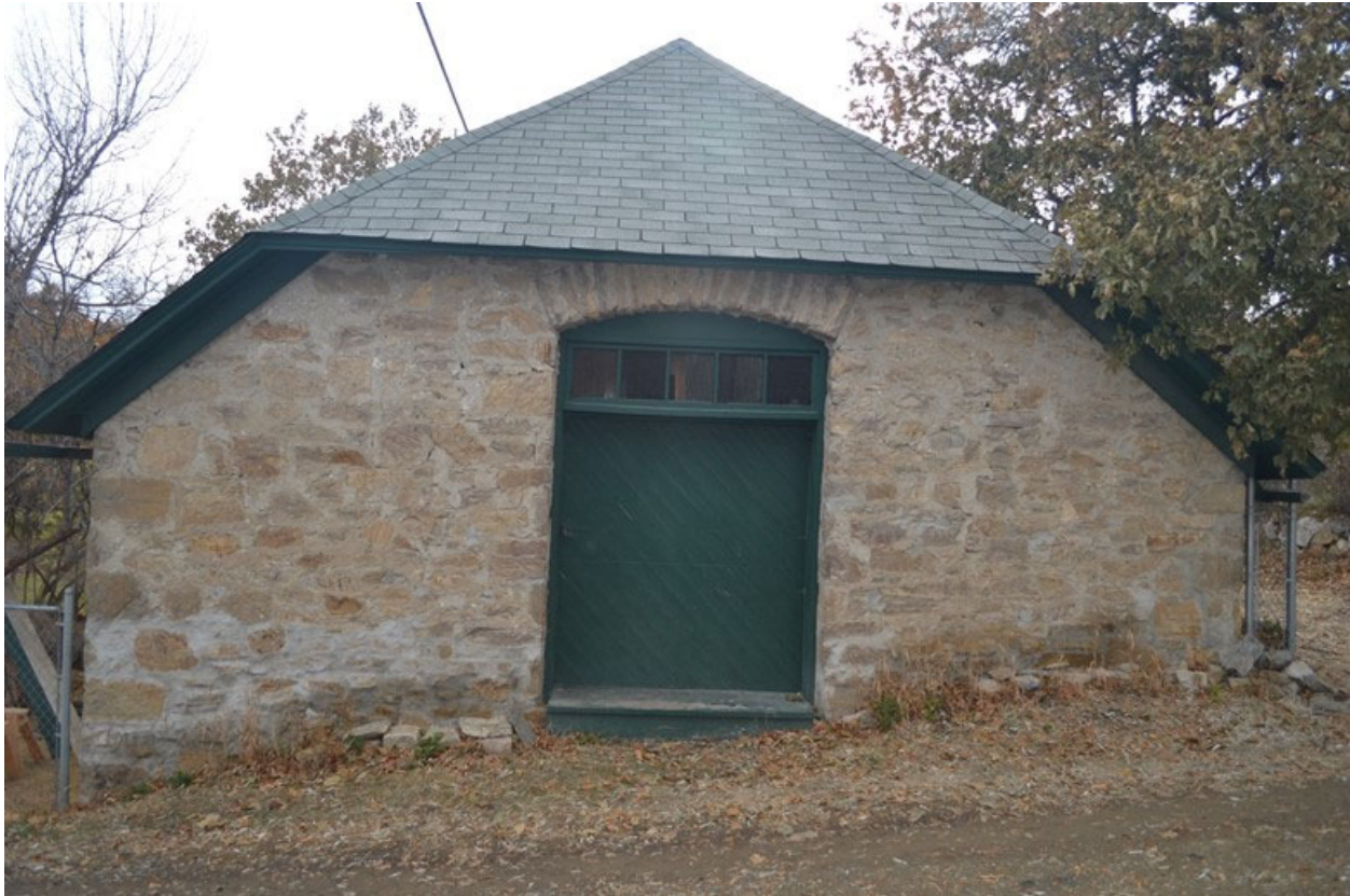
MT_LewisAndClarkCounty_Shaw'sBestFactory_0004 of 0020: Shaw's Best Factory. North Elevation looking south.
