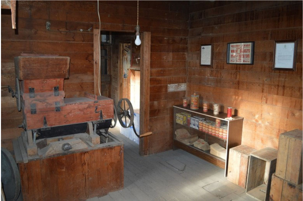
MT_LewisAndClarkCounty_Shaw'sBestFactory_0008 of 0020: Shaw's Best Factory. Second floor interior, east residential/production room, looking northwest.
