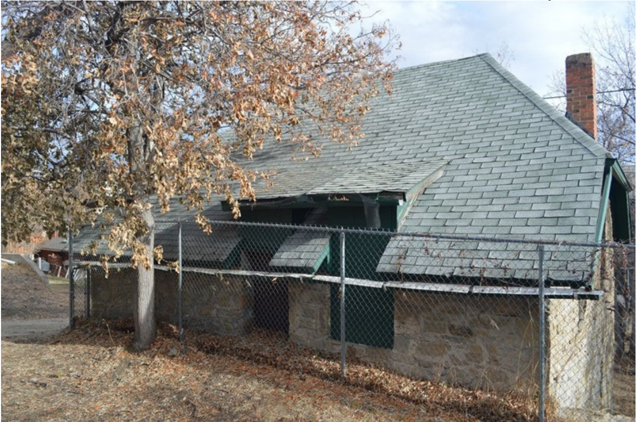
MT_LewisAndClarkCounty_Shaw'sBestFactory_0002 of 0020: Shaw's Best Factory. West Elevation looking northeast.
