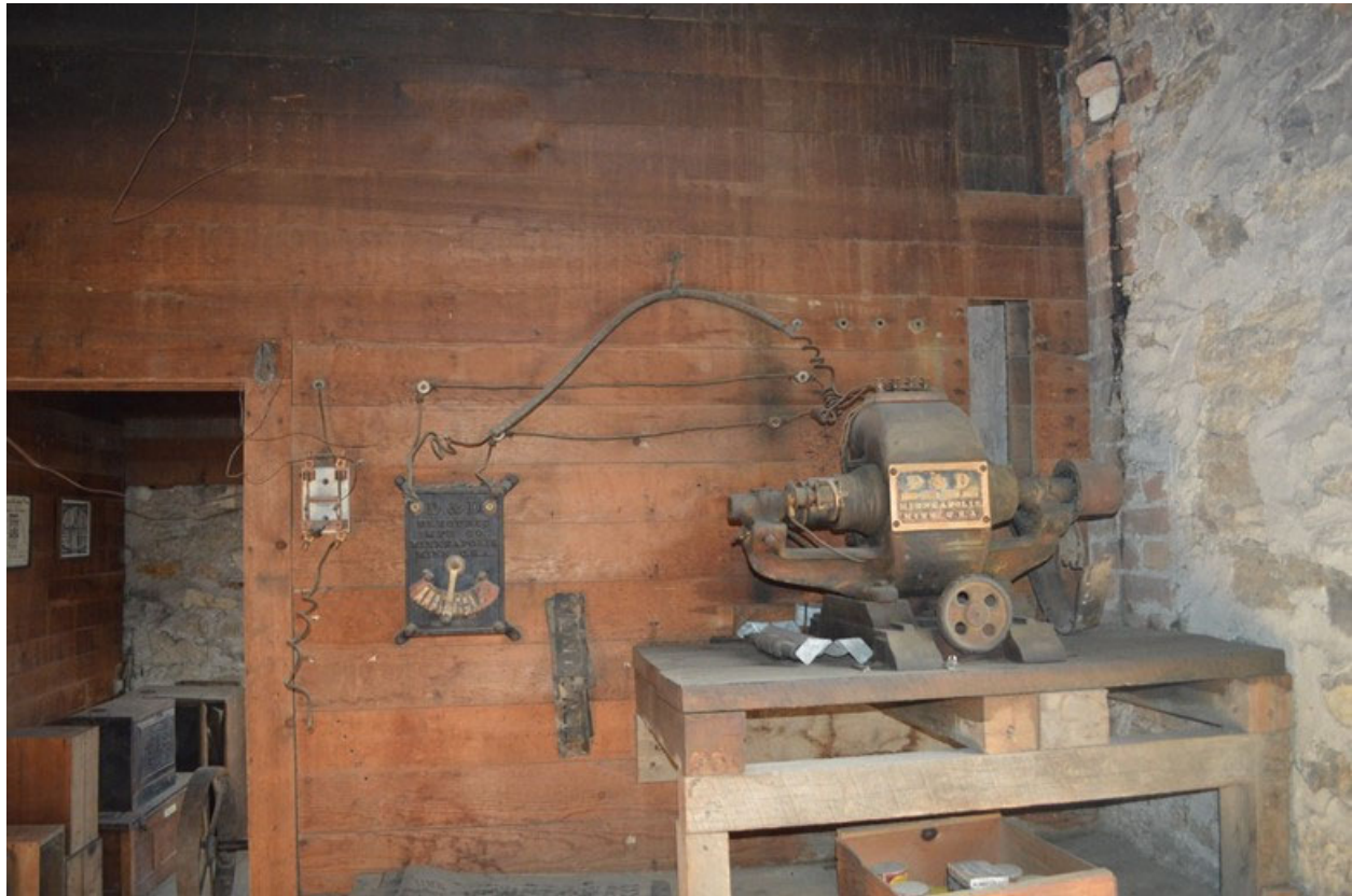
MT_LewisAndClarkCounty_Shaw'sBestFactory_0011 of 0020: Shaw's Best Factory. Second floor interior, west residential/production room, east wall, D & D motor.
