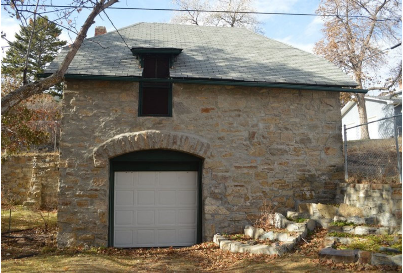
MT_LewisAndClarkCounty_Shaw'sBestFactory_0001 of 0020: Shaw's Best Factory. East Elevation looking west.
