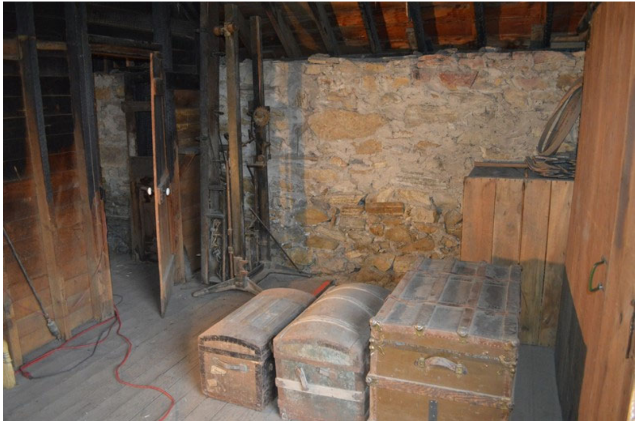
MT_LewisAndClarkCounty_Shaw'sBestFactory_0016 of 0020: Shaw's Best Factory. Second floor interior, storage room with entry into residential/production rooms, west wall, Packing and Weighing Apparatus.
