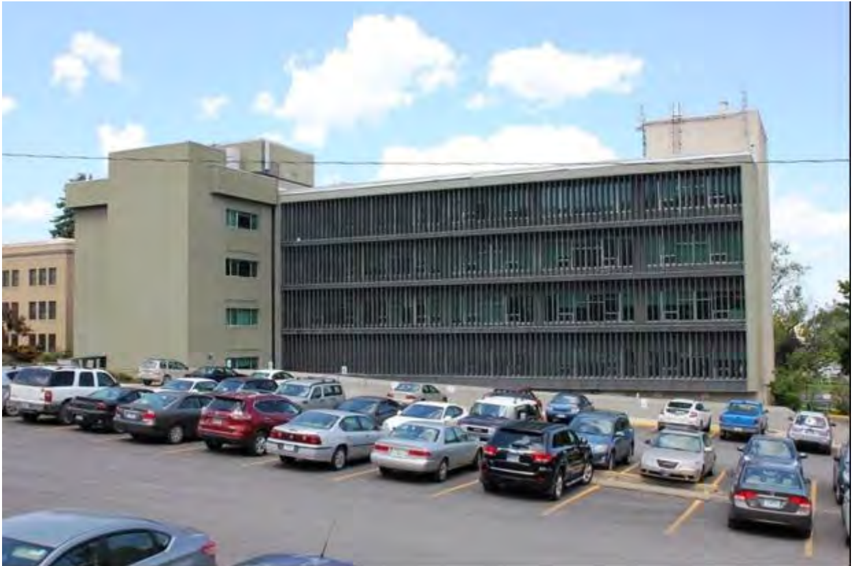
Unemployment Compensation Commission Building / Walt Sullivan Building South Elevation, Facing: NW Montana State Capitol Campus Historic District Helena, Lewis & Clark County, Montana Kate Hampton, June 22, 2015 MT_MontanaStateCapitolCampusHD_0023
