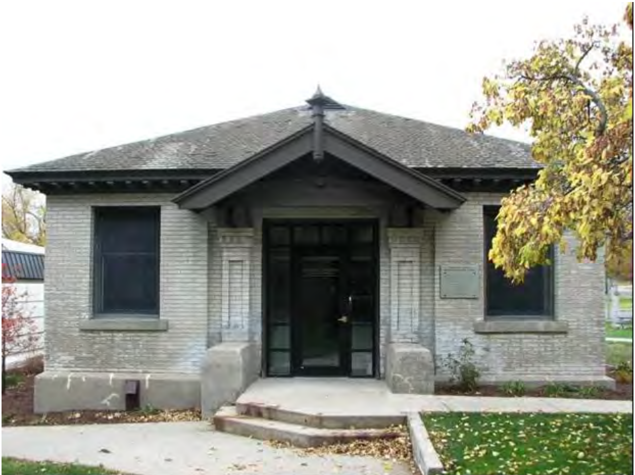
Legislative Restaurant / Capitol Annex West Façade, Facing: E Montana State Capitol Campus Historic District Helena, Lewis & Clark County, Montana Jessie Nunn, October 11, 2014 MT_MontanaStateCapitolCampusHD_0004
