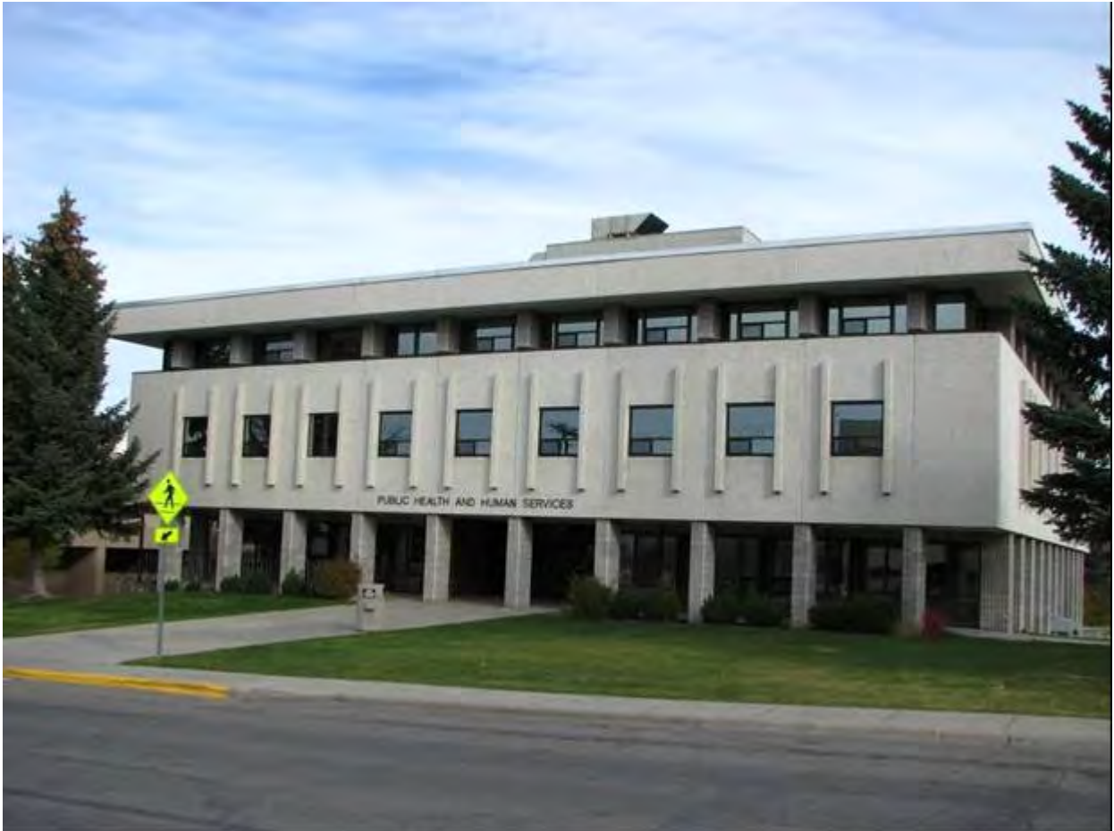
Social & Rehabilitation Services Building (DPHHS Building) West Façade, Facing: SE Montana State Capitol Campus Historic District Helena, Lewis & Clark County, Montana Jessie Nunn, October 25, 2014 MT_MontanaStateCapitolCampusHD_0027
