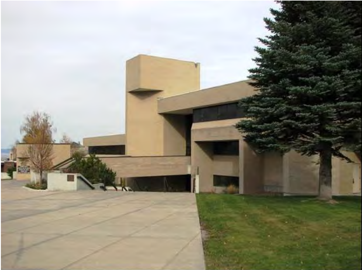
Justice Building & Montana State Library (Joseph P. Mazurek Building) West Façade with Main Entrance, Facing: SE Montana State Capitol Campus Historic District Helena, Lewis & Clark County, Montana Jessie Nunn, October 25, 2014 MT_MontanaStateCapitolCampusHD_0028
