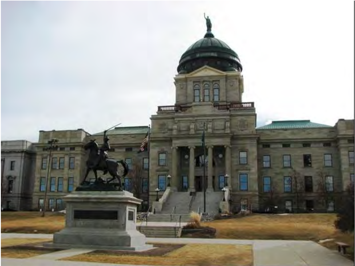
Montana State Capitol Main Entrance and Thomas Francis Meagher Statue, Facing: SE Montana State Capitol Camus Historic District Helena, Lewis & Clark County, Montana Jessie Nunn, October 11, 2014 MT_MontanaStateCapitolCampusHD_0002
