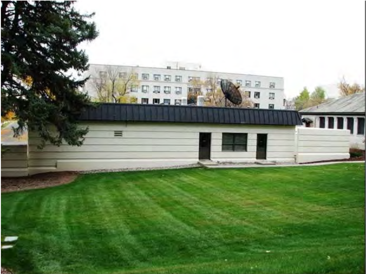
Boiler Plant West Elevation, Facing: SE Montana State Capitol Campus Historic District Helena, Lewis & Clark County, Montana Jessie Nunn, October 11, 2014 MT_MontanaStateCapitolCampusHD_0006
