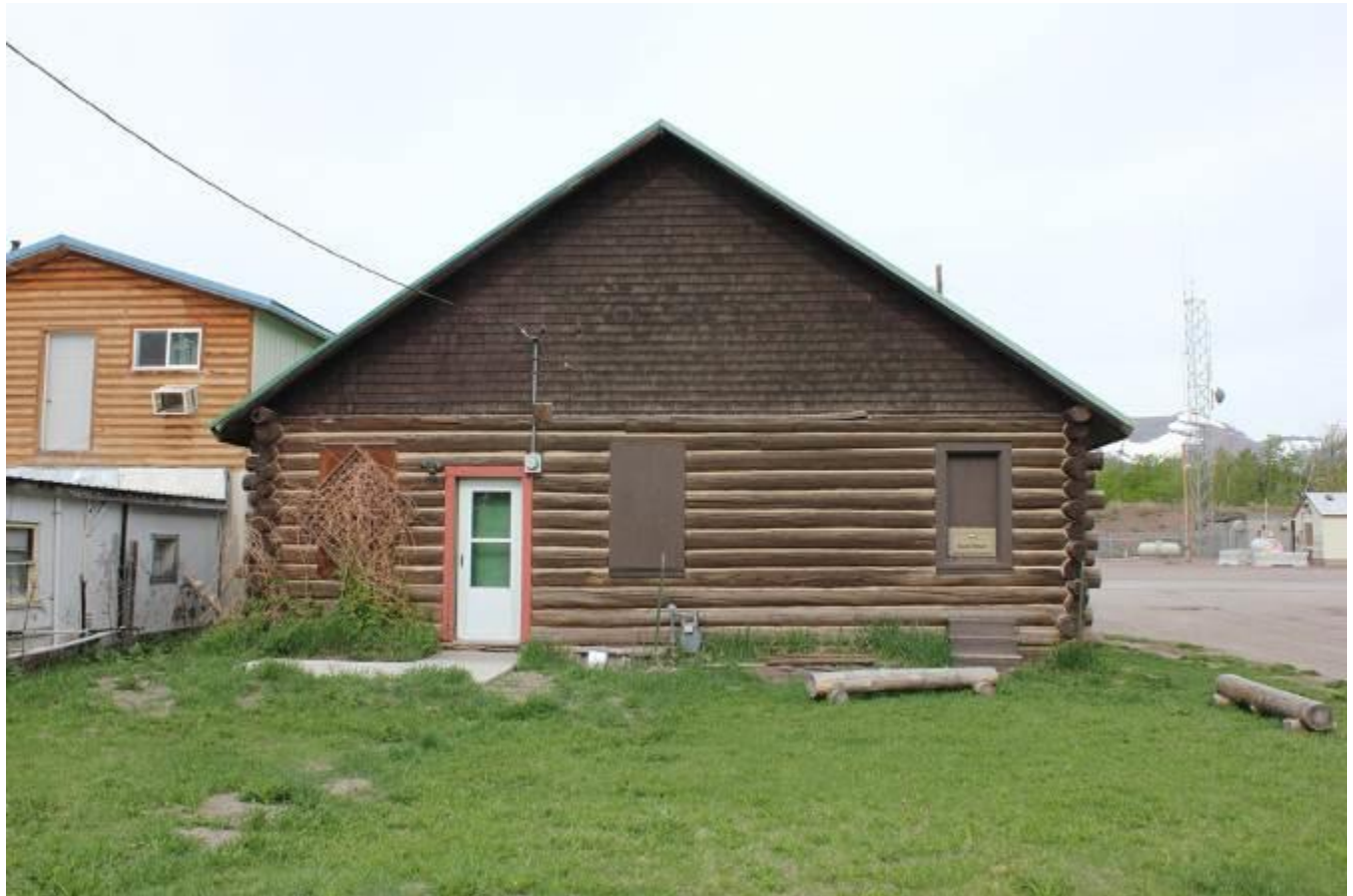
Description of Photograph(s) and number: West (rear) elevation. MT_GlacierCounty_GlacierParkWomen'sClub_0004 of 0011.
