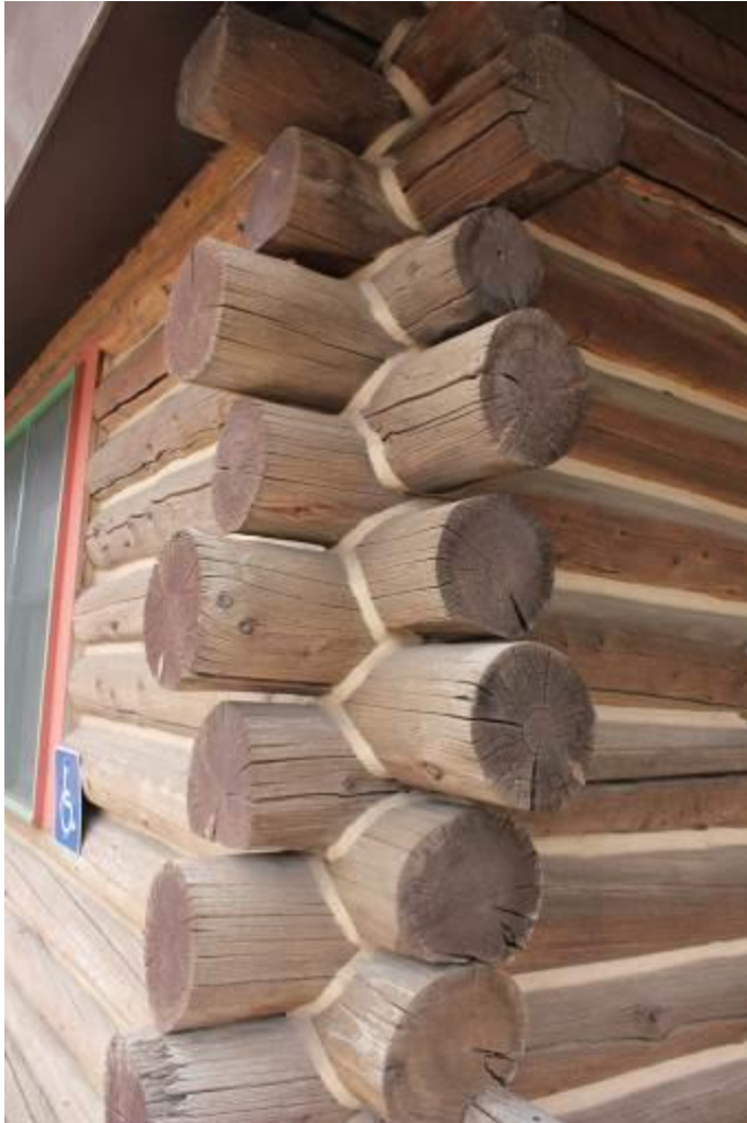
Description of Photograph(s) and number: detail of saddle notching at southwest corner. MT_GlacierCounty_GlacierParkWomen'sClub_0006 of 0011.
