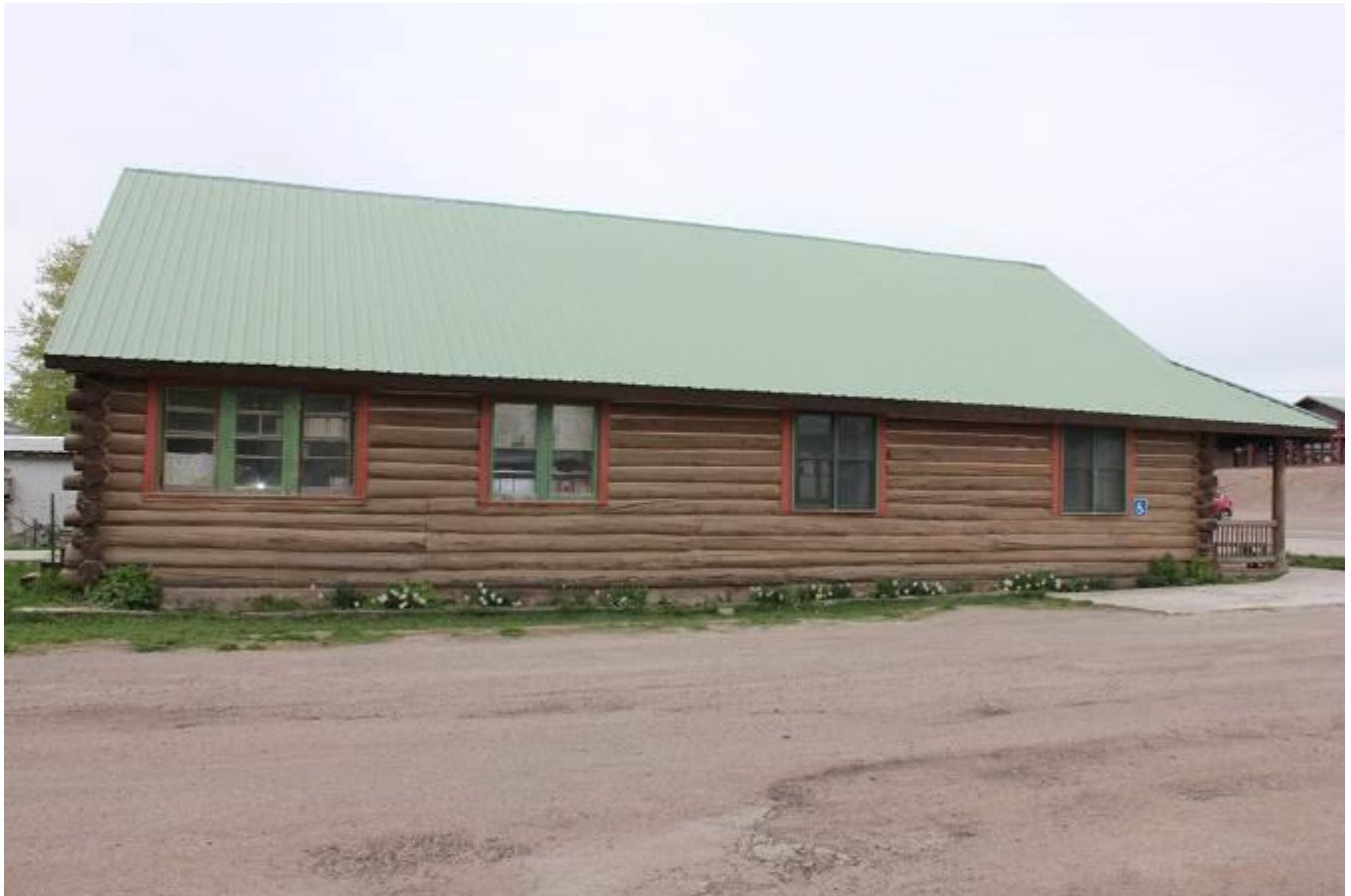
Description of Photograph(s) and number: North (side) elevation. MT_GlacierCounty_GlacierParkWomen'sClub_0002 of 0011.
