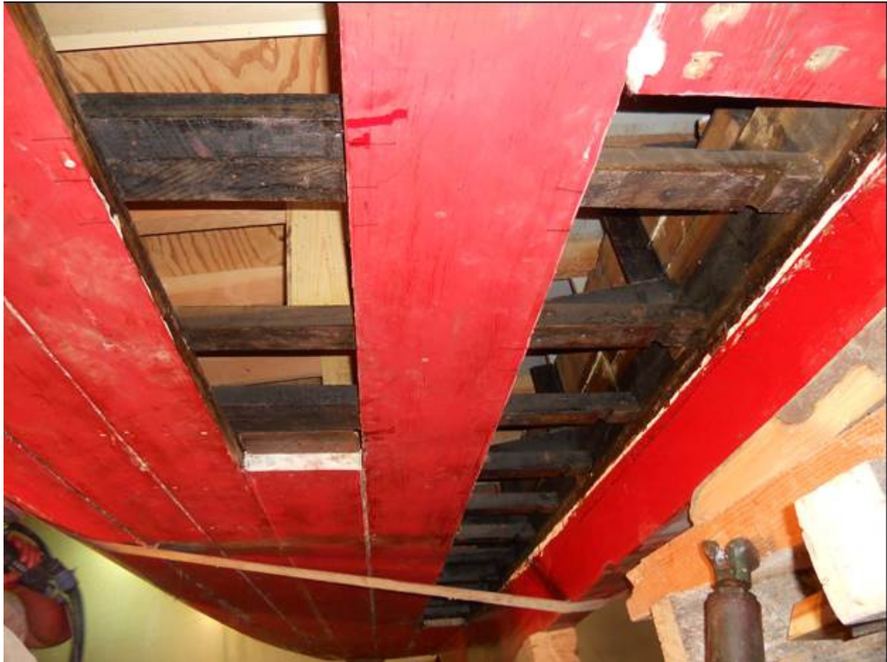
MT_GlacierCounty_Rising Wolf_0010, bottom garboard plank frames keel.
