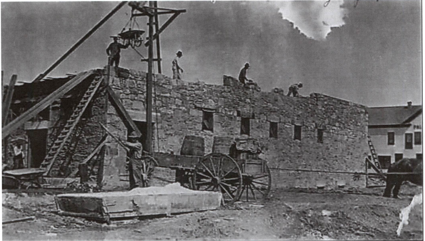
Construction of Stafford's Grocery Store, circa 1914.
