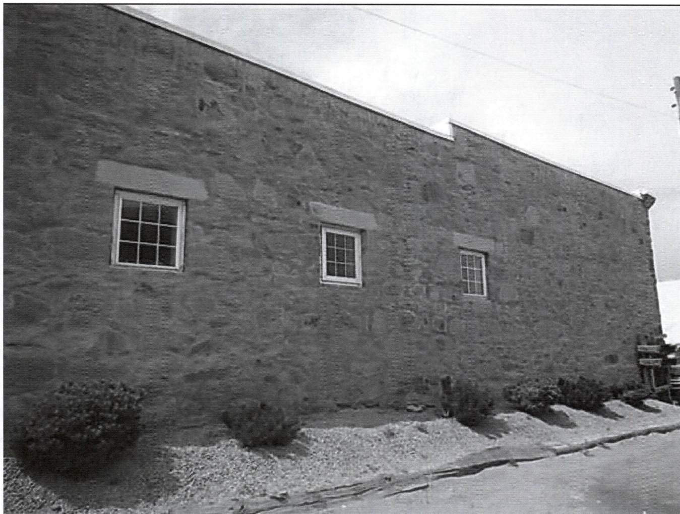
MT_FergusCounty_Stafford'sGrocery_0010. East wall. View looking northwest.
