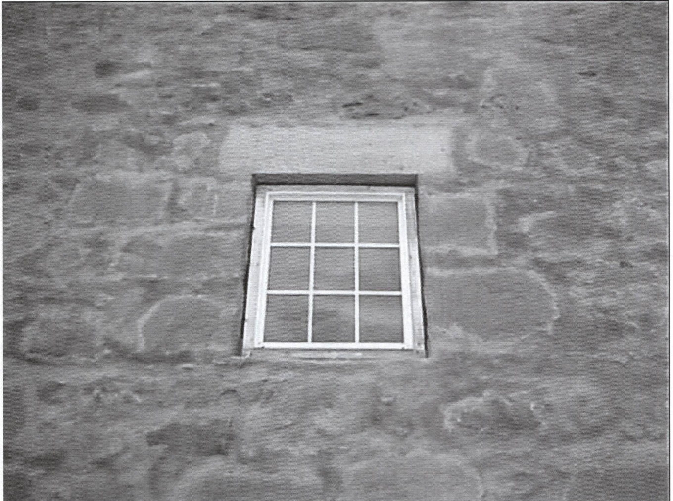
MT_FergusCounty_Stafford'sGrocery_0009. Detail of window on east wall. View looking west.
