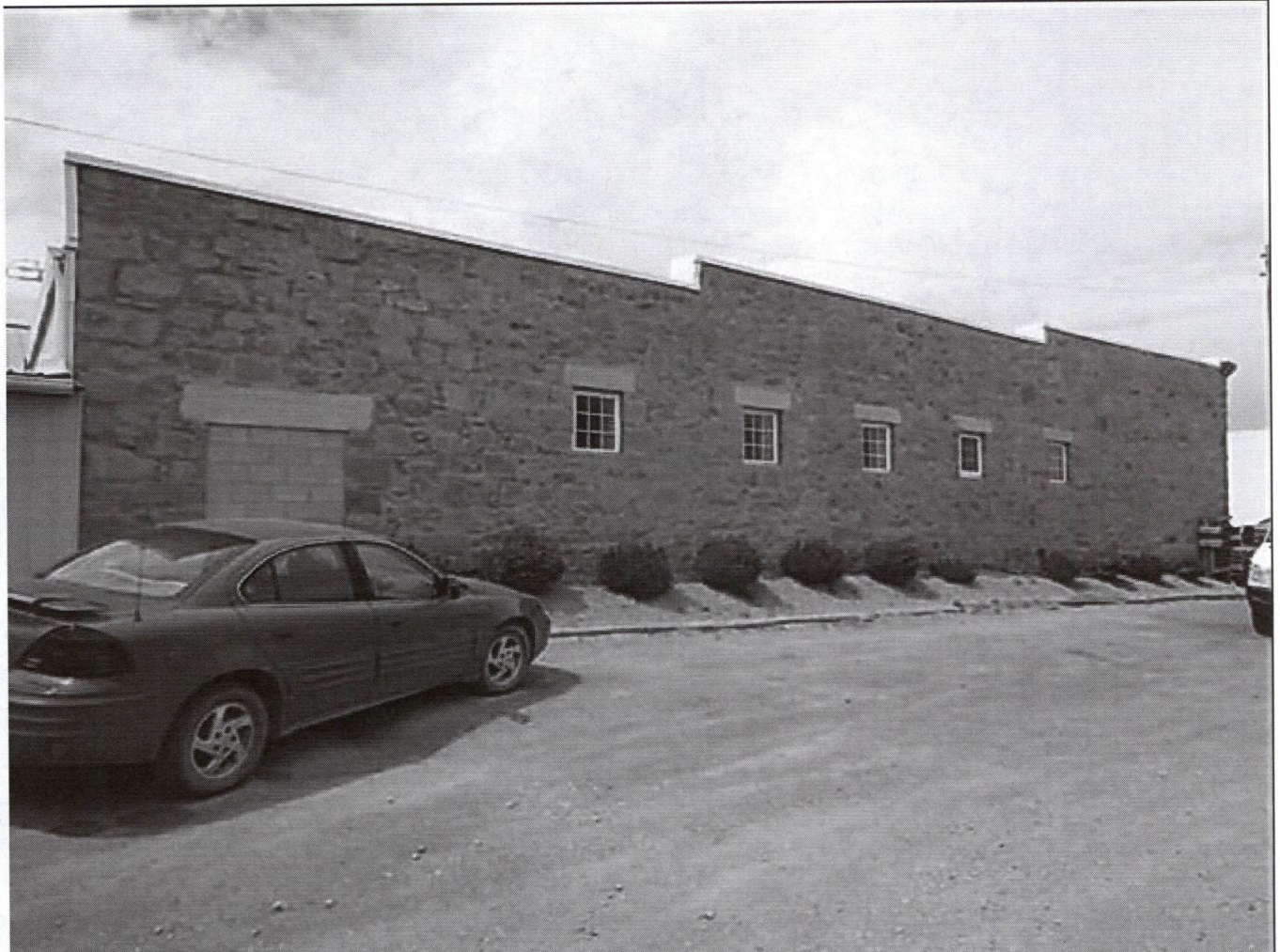
MT_FergusCounty_Stafford'sGrocery_0005. East wall. View looking north-northwest
