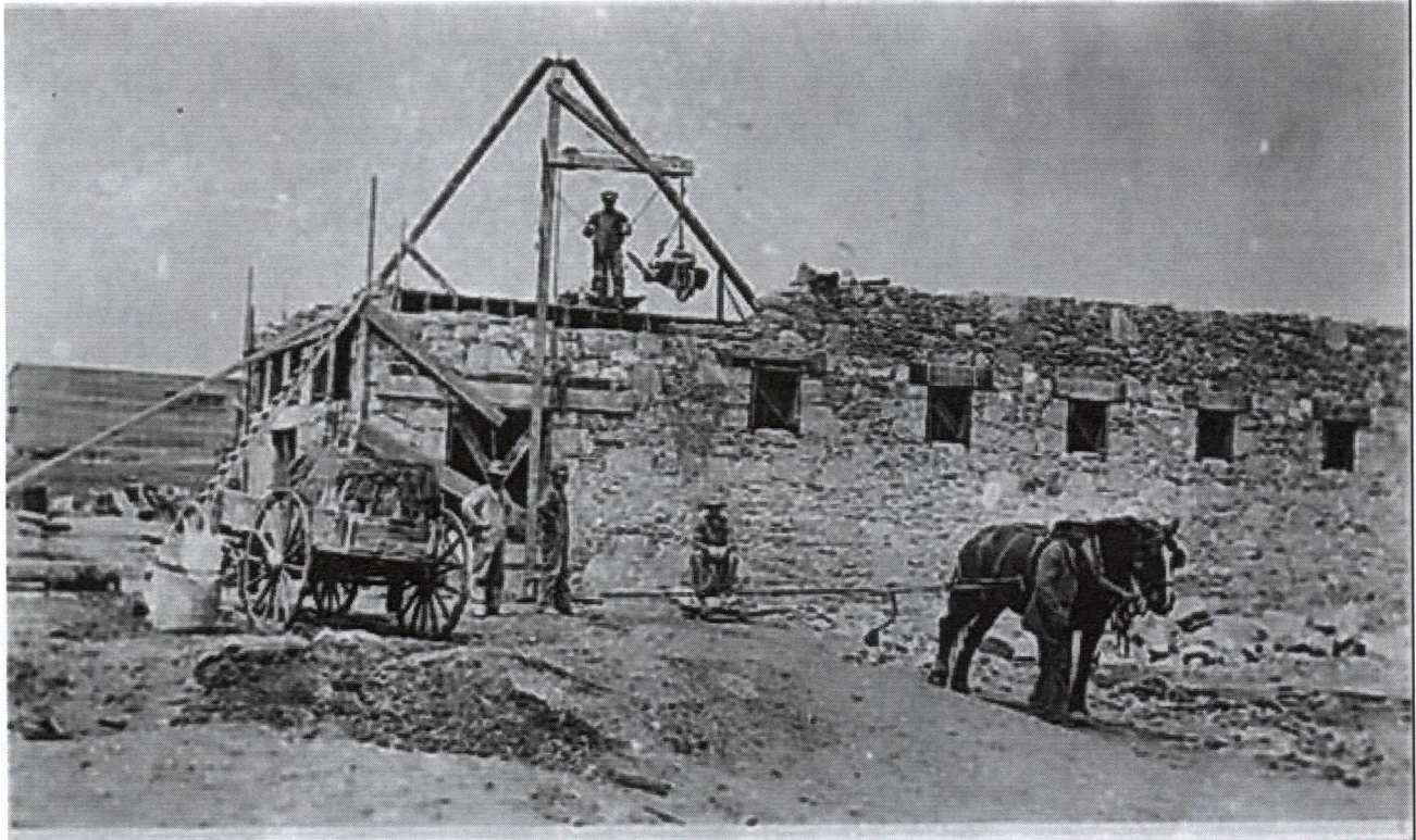
Construction of Stafford's Grocery Store, circa 1914.
