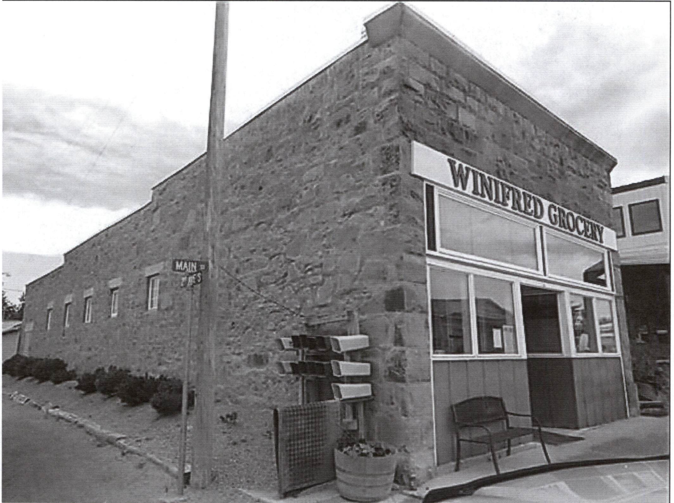
MT_FergusCounty_Stafford'sGrocery_0011. Façade (north) and east wall. View looking southwest.
