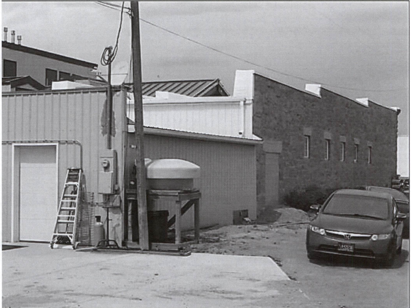
MT_FergusCounty_Stafford'sGrocery_0007. Rear (south) façade and east wall. View looking north-northwest
