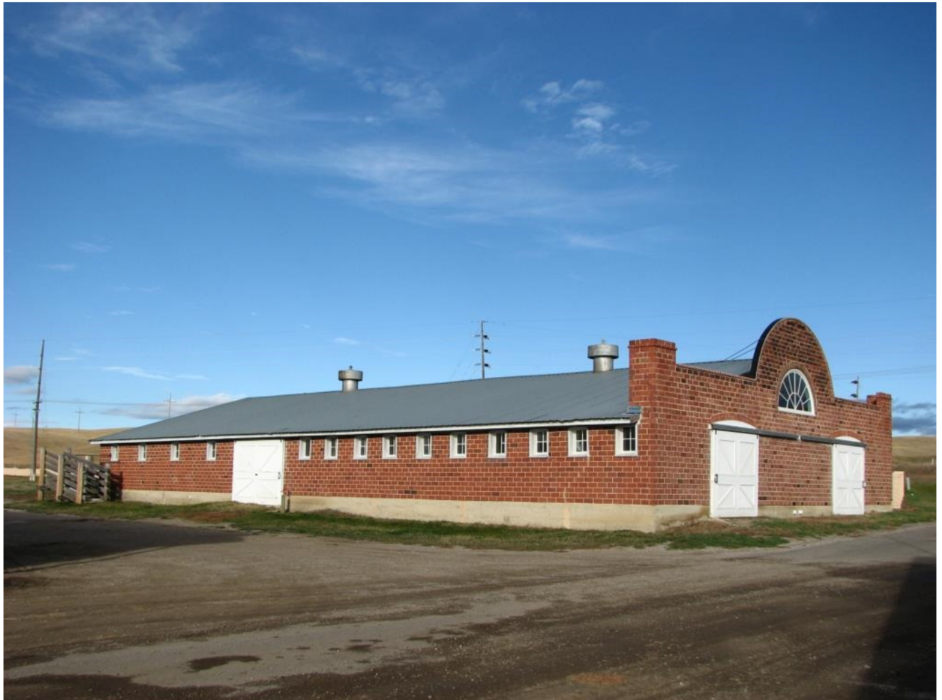
Photo 0002. South Façade and West Elevation, Facing: NE
