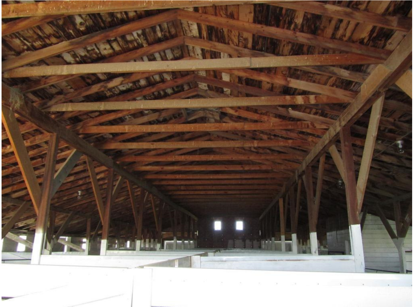
Photo 0008. Interior, Detail of Roof Structure, Facing: N
