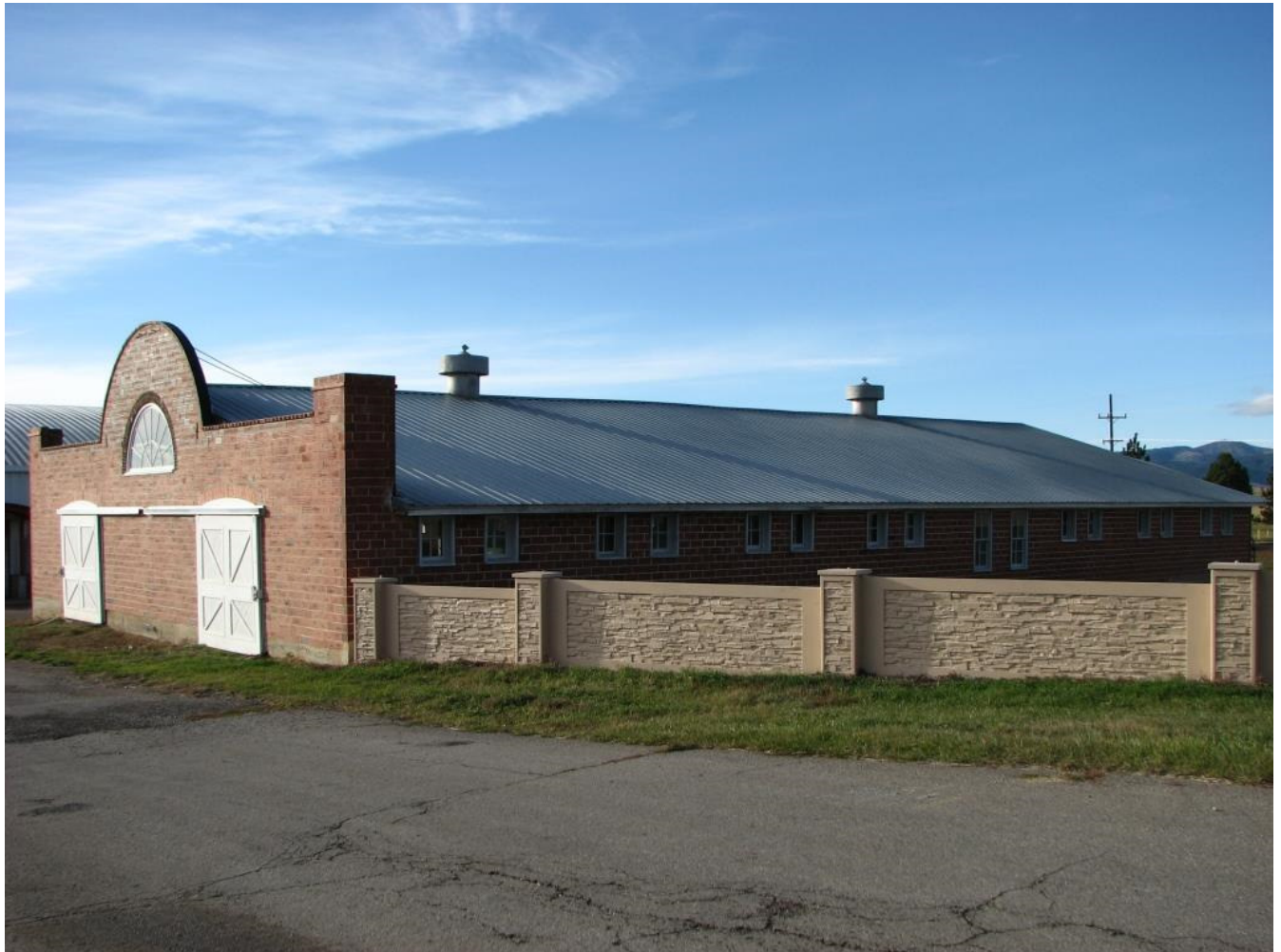
Photo 0004. South Façade and East Elevation, Facing: NW
