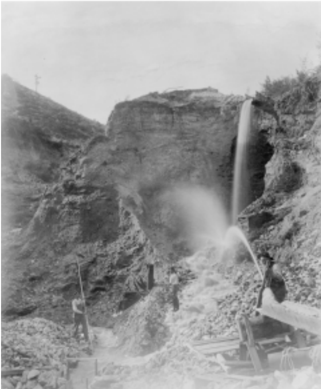
Hydraulic mining on Nelson Gulch near Helena, Montana, about 1905.
