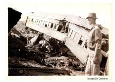
The Custer Creek train wreck (sometimes called the Saugus train wreck) is the worst rail disaster in Montana history. It occurred on June 19, 1938, when a bridge collapsed beneath the Milwaukee Road's "Olympian" as it crossed Custer Creek, southwest of Terry, Montana. Caused by a flash flood that washed away the foundations of the bridge, the crash killed 47 people. Join Bill Jones as he recounts his father's story of surviving this horrific incident.
