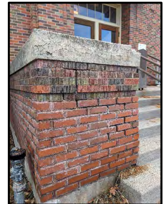
International Center west entrance and brick pier damage, February 2024. Photos: Nikki Manning
