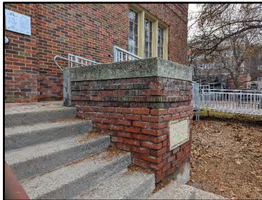
International Center west entrance and brick pier damage, February 2024. Photos: Nikki Manning
