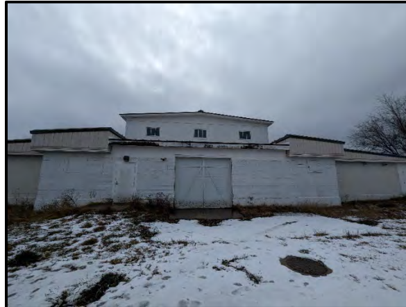
North elevation T-156, February 4, 2024. Photos: Nikki Manning
