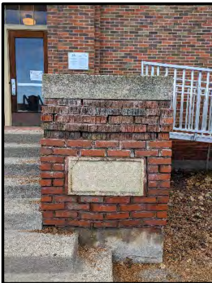
International Center west entrance and brick pier damage, February 2024. Photos: Nikki Manning
