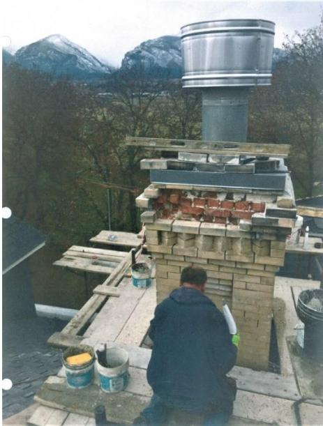
Picture 9: Daly Mansion: brick chimney being repaired
