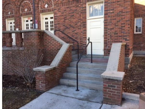
Picture 5: Elrod steps: new concrete steps & handrails
