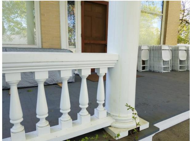
Picture 16: Porch balusters repaired, anchored &
