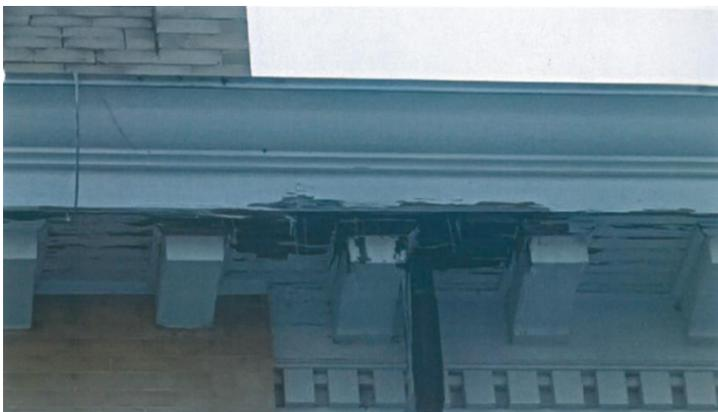
Picture 11: High roof trim & fascia before repair showing damage.
