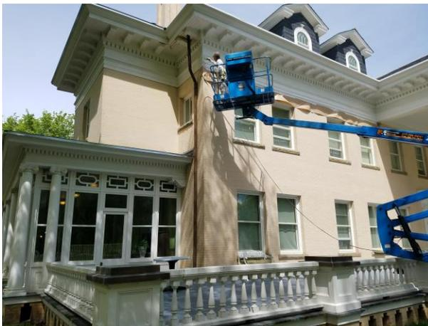
Picture 15: Roof trim being repaired & painted
