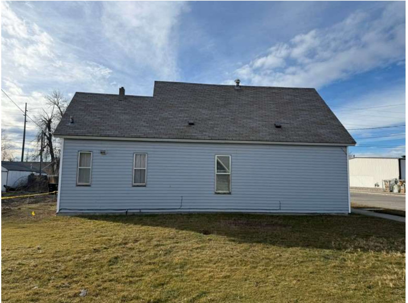
Photo: MT_YellowstoneCounty_WaymanChapelAMEChurchAndParsonage_0014. Parsonage, east elevation, view to the southwest. Kate Hampton, January 2026.
