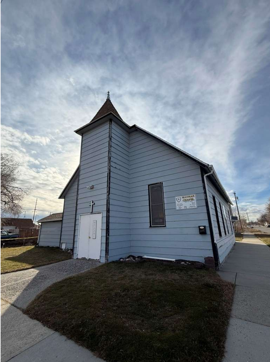
Photo: MT_YellowstoneCounty_WaymanChapelAMEChurchAndParsonage_0002. Wayman Chapel east elevation, view to the south. Photographer Kate Hampton, January 2026.
