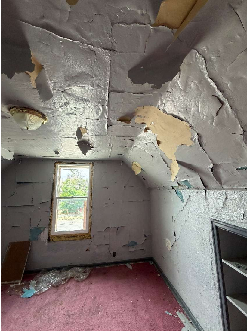
Photo: MT_YellowstoneCounty_WaymanChapelAMEChurchAndParsonage_0018. Parsonage, upstairs front room, view to the northwest. Brennan DeBoer, July 2026.
