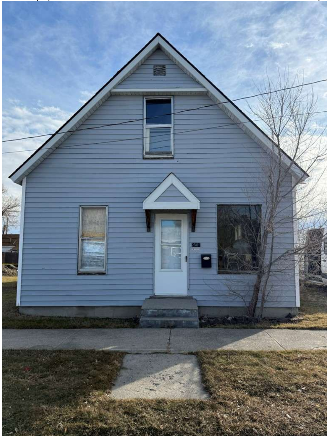
Photo: MT_YellowstoneCounty_WaymanChapelAMEChurchAndParsonage_0013. Parsonage, north elevation, view to the southeast. Kate Hampton, January 2026.
