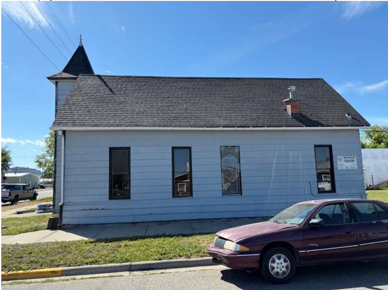
Photo: MT_YellowstoneCounty_WaymanChapelAMEChurchAndParsonage_0006. Wayman Chapel north elevation, view to the south southwest. Brennan DeBoer, July 2026.
