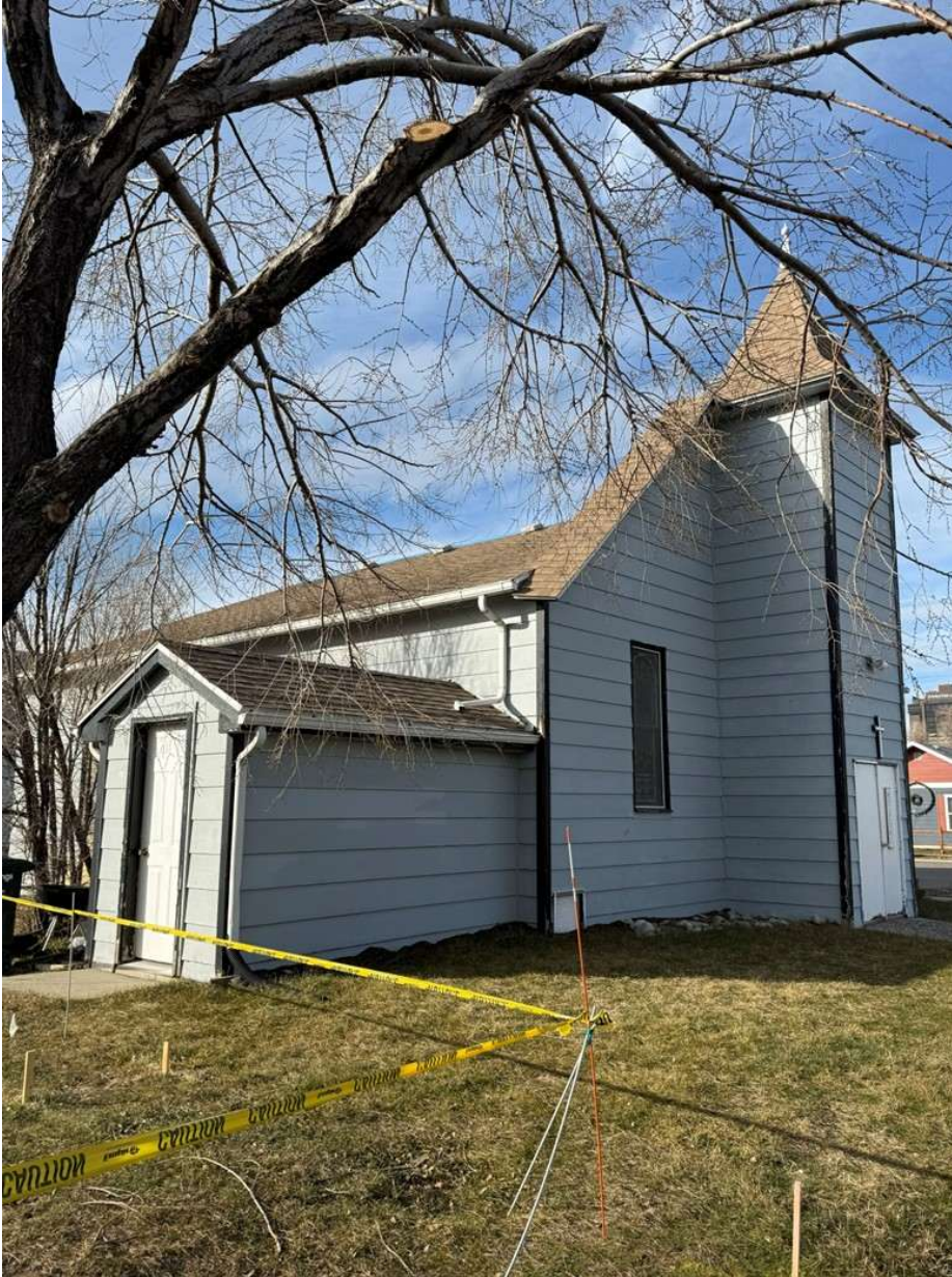
Photo: MT_YellowstoneCounty_WaymanChapelAMEChurchAndParsonage_0003. Wayman Chapel east elevation, view to the north northwest. Kate Hampton January 2026.
