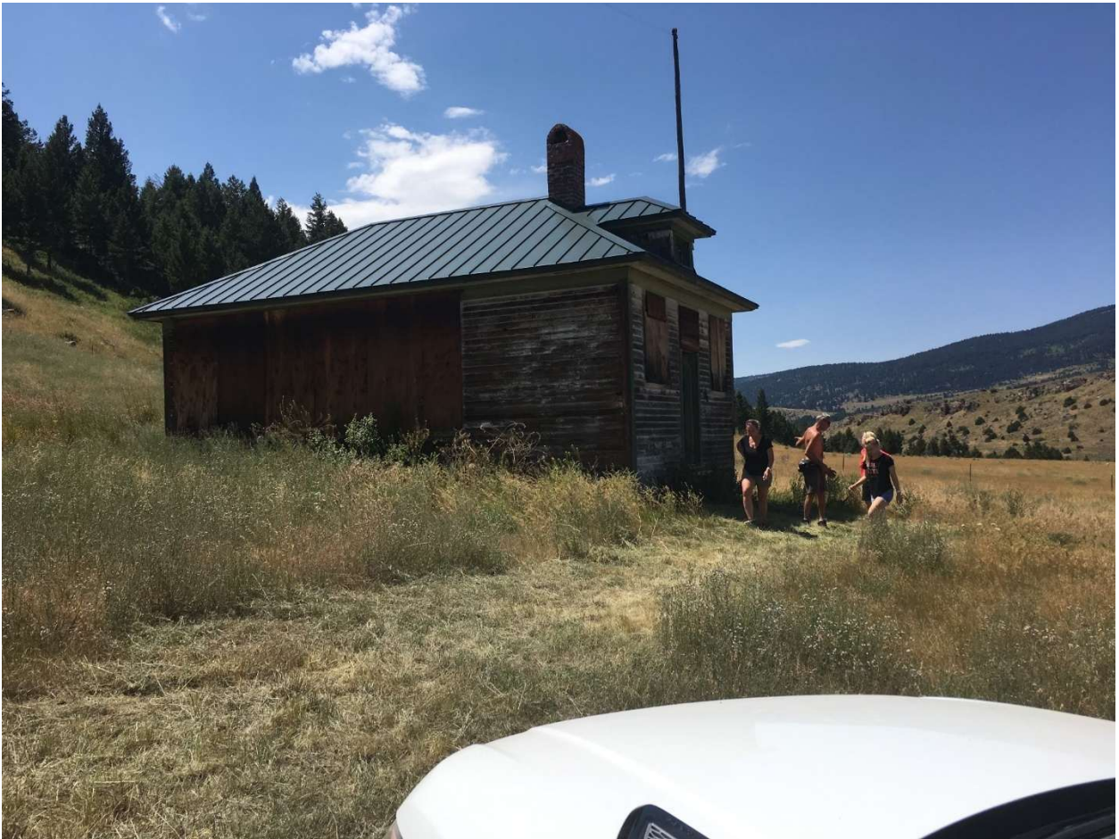
MT_MeagherCounty_SixteenSchool_0002: East and north elevations of Sixteen School, view to the southwest.
