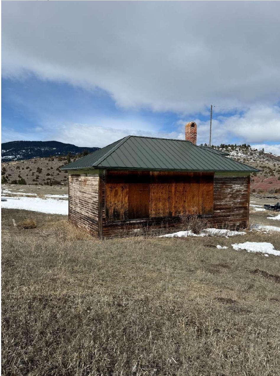
MT_MeagherCounty_SixteenSchool_0003: South and east elevations of Sixteen School, view to the northwest
