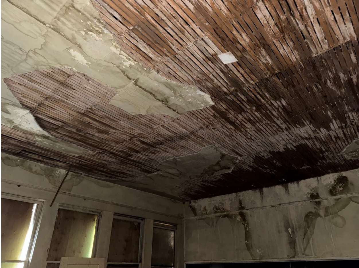
MT_MeagherCounty_SixteenSchool_0009: East and south walls and ceiling of Sixteen School, view to the southeast
