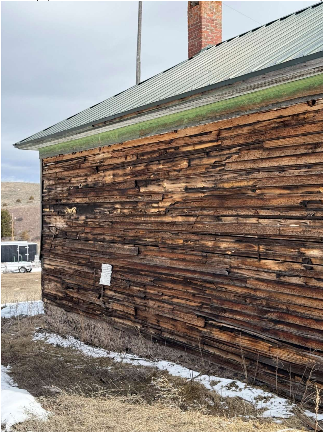
MT_MeagherCounty_SixteenSchool_0004: West elevation of Sixteen School, view to the northeast.
