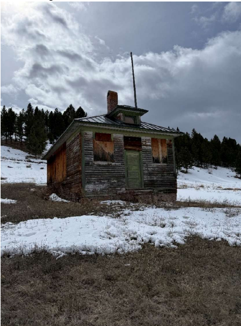
MT_MeagherCounty_SixteenSchool_0001: Front façade/north elevation of Sixteen School, view to the south.
