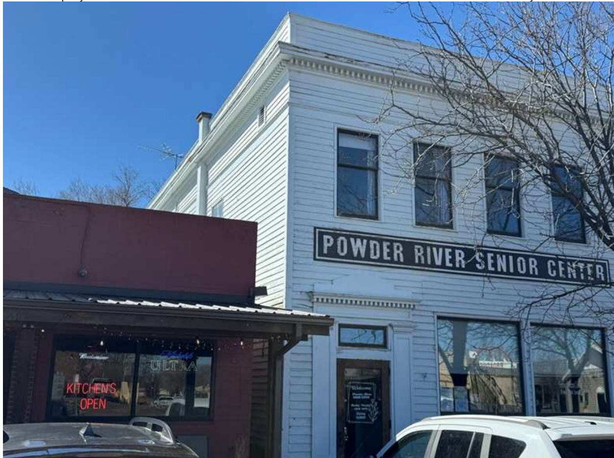
MT_PowderRiverCounty_0004: Powder River County Bank, east and south elevations, view to the northwest
