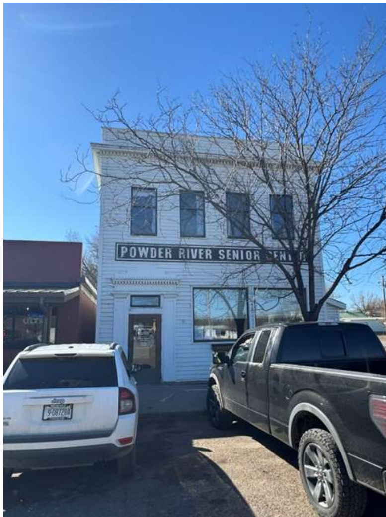
MT_PowderRiverCounty_0001: Powder River County Bank, east elevation, view to the west
