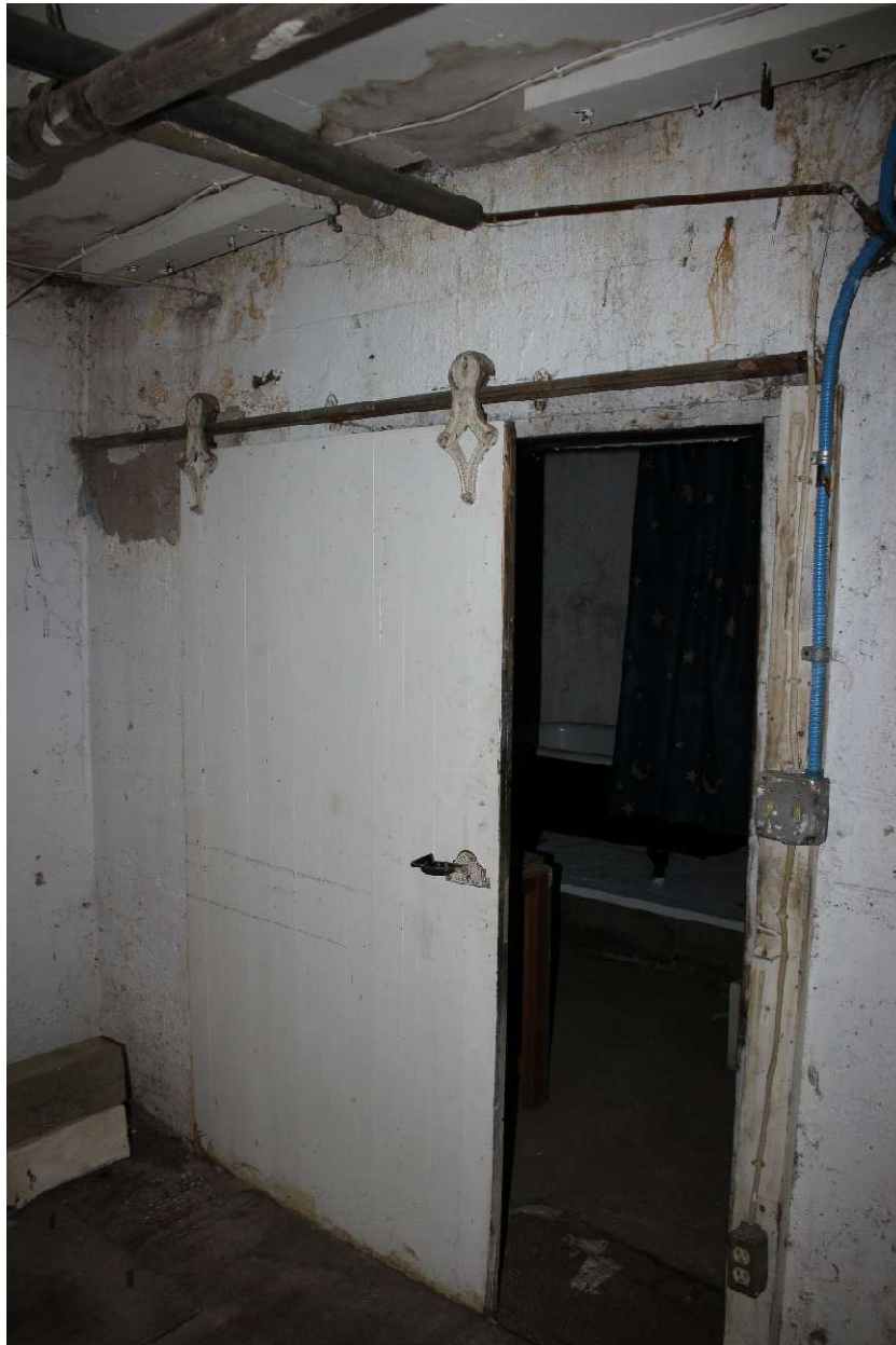
MT_PowderRiverCounty_0017: Powder River County Bank, basement interior, what exactly is this??? view to the southwest ???
