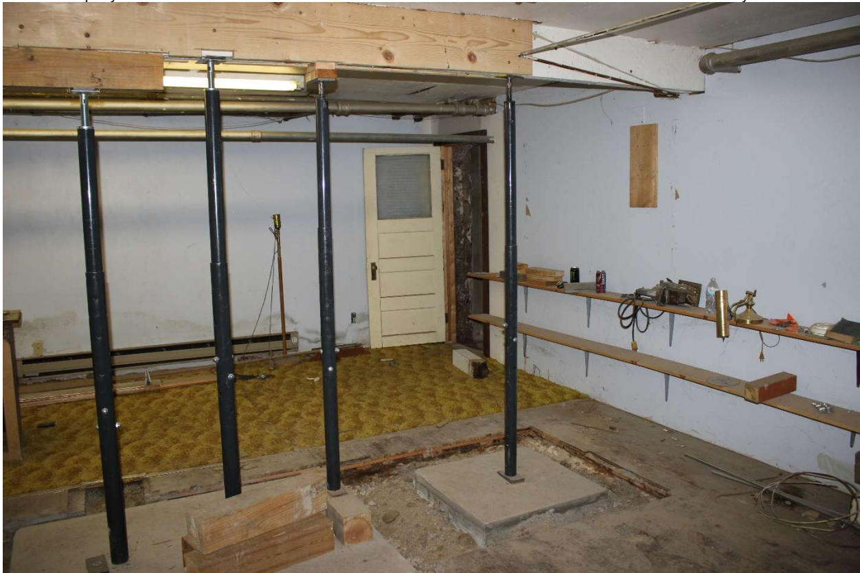
MT_PowderRiverCounty_0016: Powder River County Bank, basement interior, view to the southwest ???
