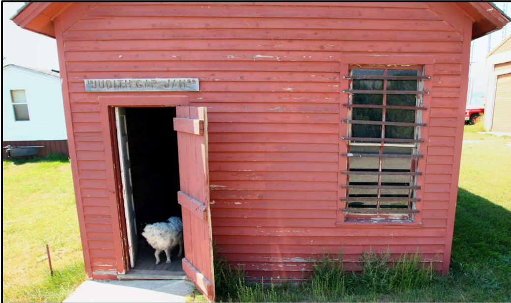
Photo 4: MT_WheatlandCounty_JudithGapJail_0004. Judith Gap Jail in 2025, east elevation details of door and window, view direction west. This is a stitched image as evidenced by paint variance. (Photographer: James Busse)
