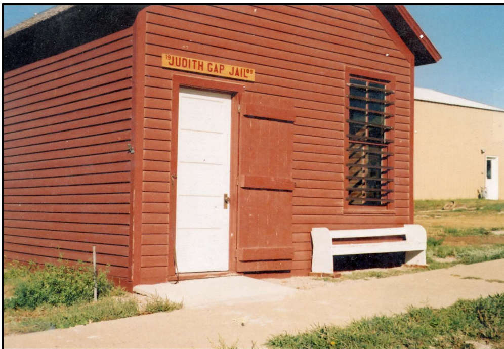
Photo 17: MT_WheatlandCounty_JudithGapJail_0017. Finished exterior following renovation in 2002. View direction northwest. (Photographer: Alice Bair)
