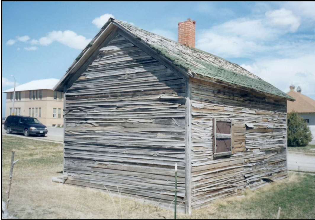
Photo 14: MT_WheatlandCounty_JudithGapJail_0014. Building exterior prior to renovation in 2002. View direction northeast. (Photographer: Alice Bair)
