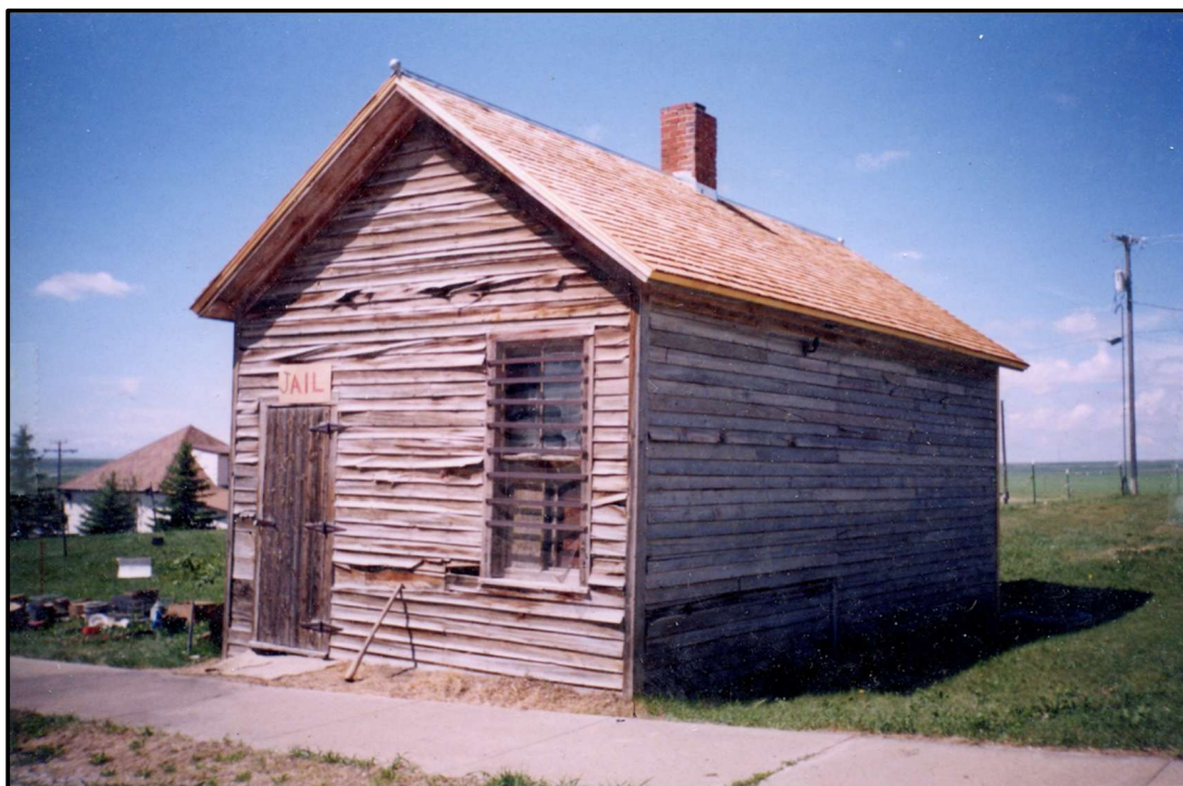
Photo 15: MT_WheatlandCounty_JudithGapJail_0015. Building with a new roof during renovation in 2002. View direction southwest. (Photographer: Alice Bair)
