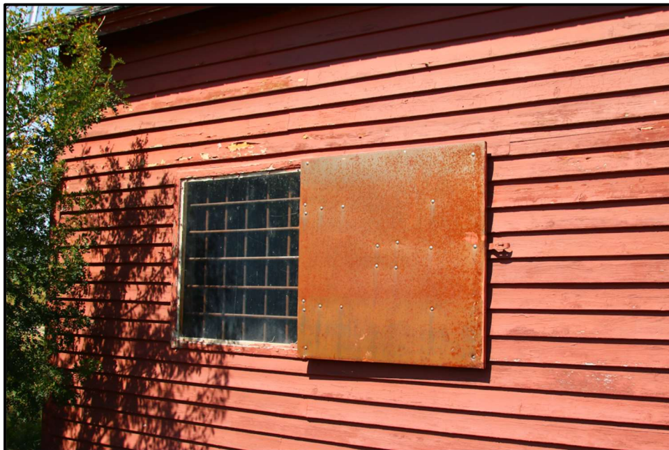
Photo 5: MT_WheatlandCounty_JudithGapJail_0005. Judith Gap Jail in 2025, south elevation detail of holding cell window and cover, view direction northwest. (Photographer: James Busse)
