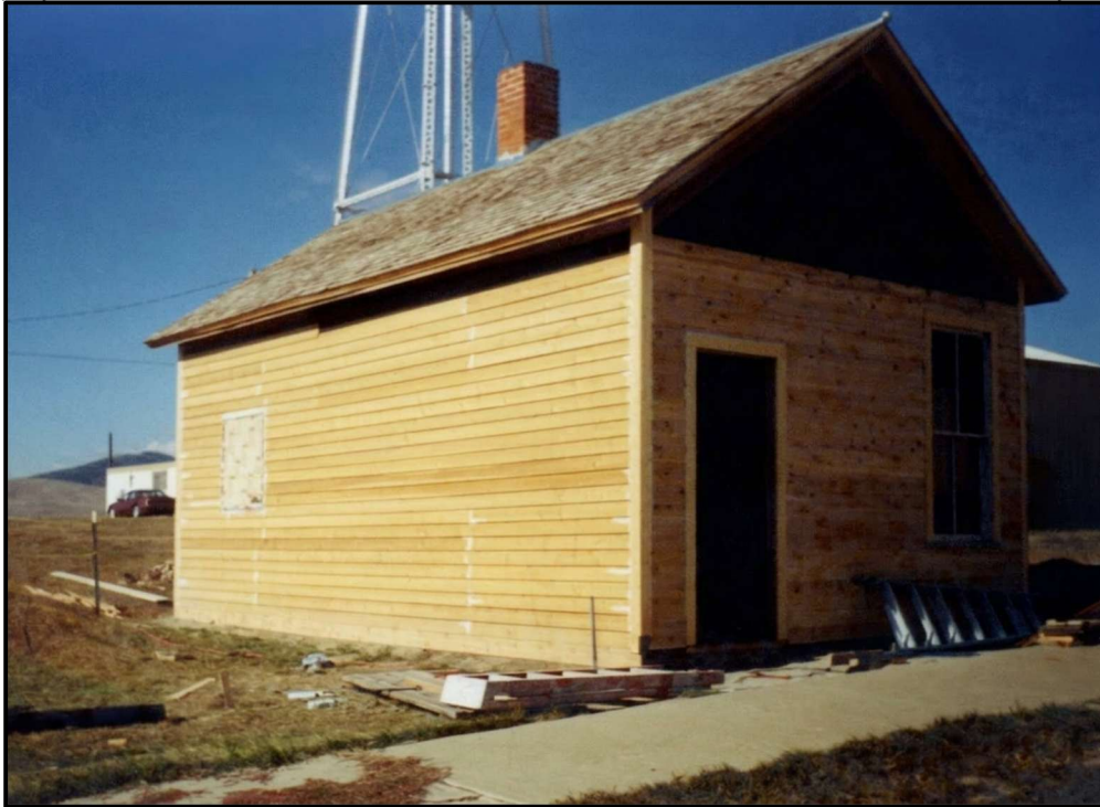
Photo 16: MT_WheatlandCounty_JudithGapJail_0016. Building with tarpaper underlayment and new siding during renovation in 2002. View direction northwest. (Photographer: Alice Bair)
