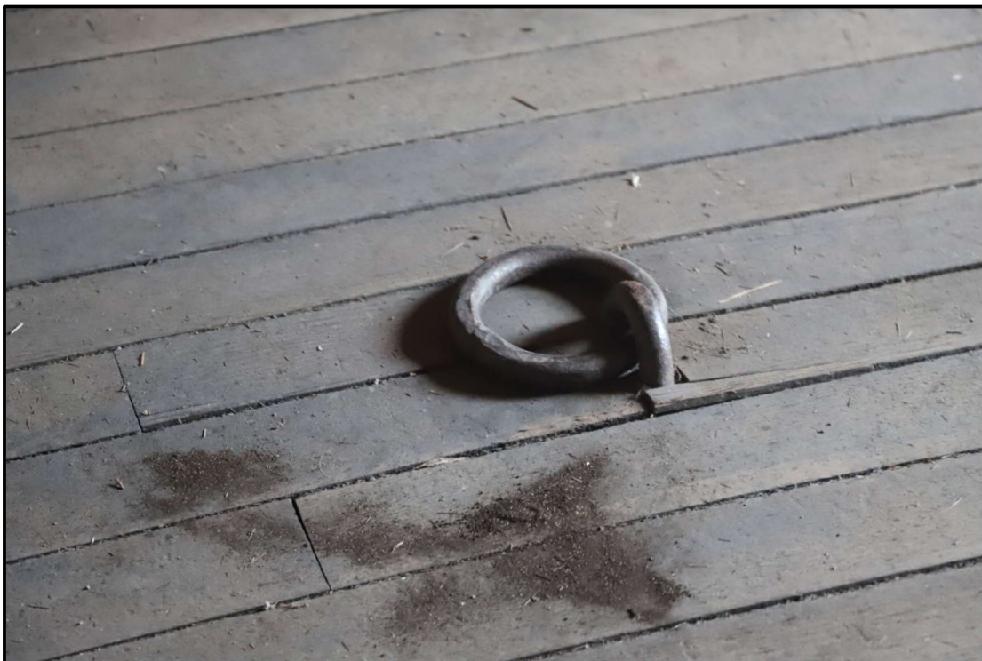
Photo 12: MT_WheatlandCounty_JudithGapJail_0012. Forged steel floor ring in 2025. View direction east. (Photographer: Tim Urbaniak)
