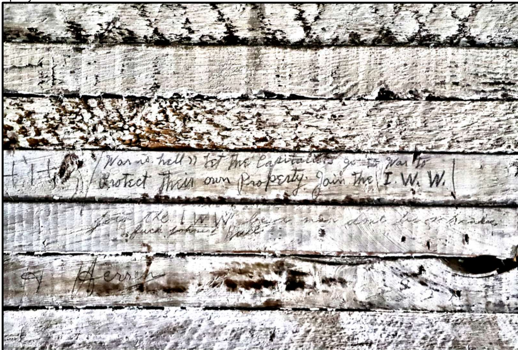
Photo 20: MT_WheatlandCounty_JudithGapJail_0020. View of IWW inscription on cell wall B4 that reads "War is hell. Let the capitalists go to war to protect their own property. Join the I.W.W." View direction east in 2025. (Photographer: Tim Urbaniak)
