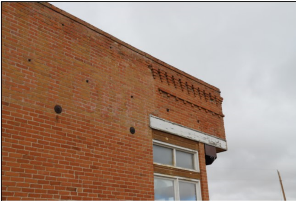
MT_FergusCounty_GarneillCommunityCenter_0006. View of the east wall showing the bracing anchor plates and bolts. View direction northwest. (Photographer: Tim Urbaniak)
