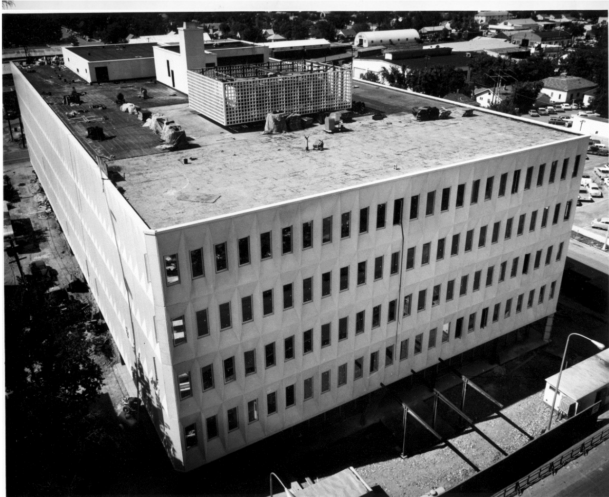
MT_YellowstoneCounty_JamesFBattin Federal Building_0031, Feature #H-2 Description: Battin Federal Building. Photograph courtesy of the Western Heritage Center, accession #2006.06.829. Facing: Northeast at the roof during construction, c. 1965. Note the tighter grid of precast panels screening the cooling tower. The current panels are similar to the scale of the building's window panels.
