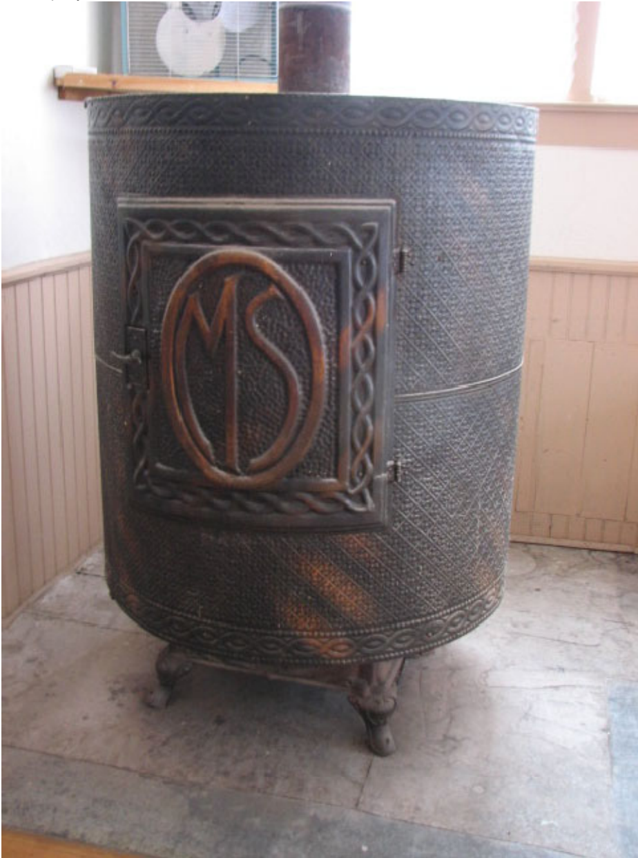
MT_RavalliCounty_ComoSchool_0006: Detail of the Manuel-Smith heating system, southwest corner of the classroom.
