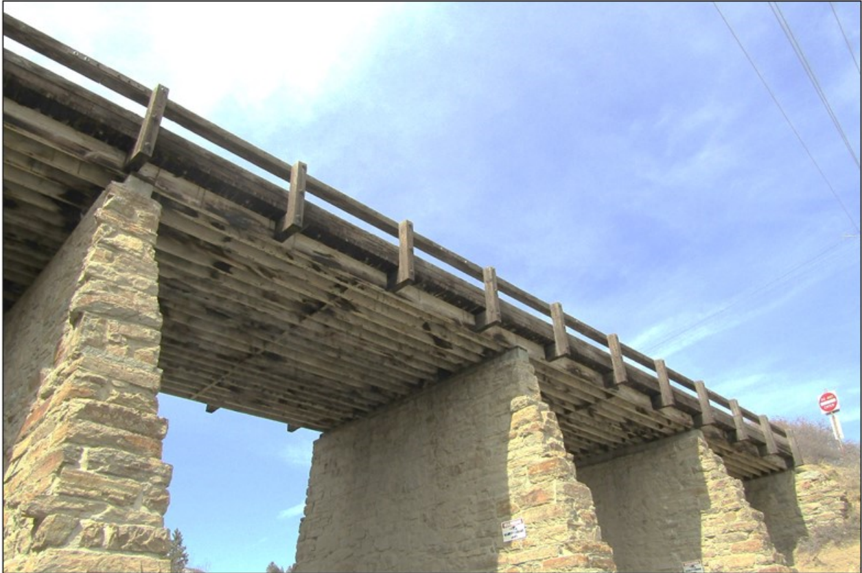
Morelli Bridge. Detail of bents, underside of deck, and guardrails. View to northwest. MT_LewisandClarkCounty_MorelliBridge_0012.
