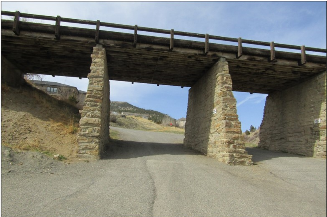
Morelli Bridge. Detail of rubblestone bents. View to west. MT_LewisandClarkCounty_MorelliBridge_0009.
