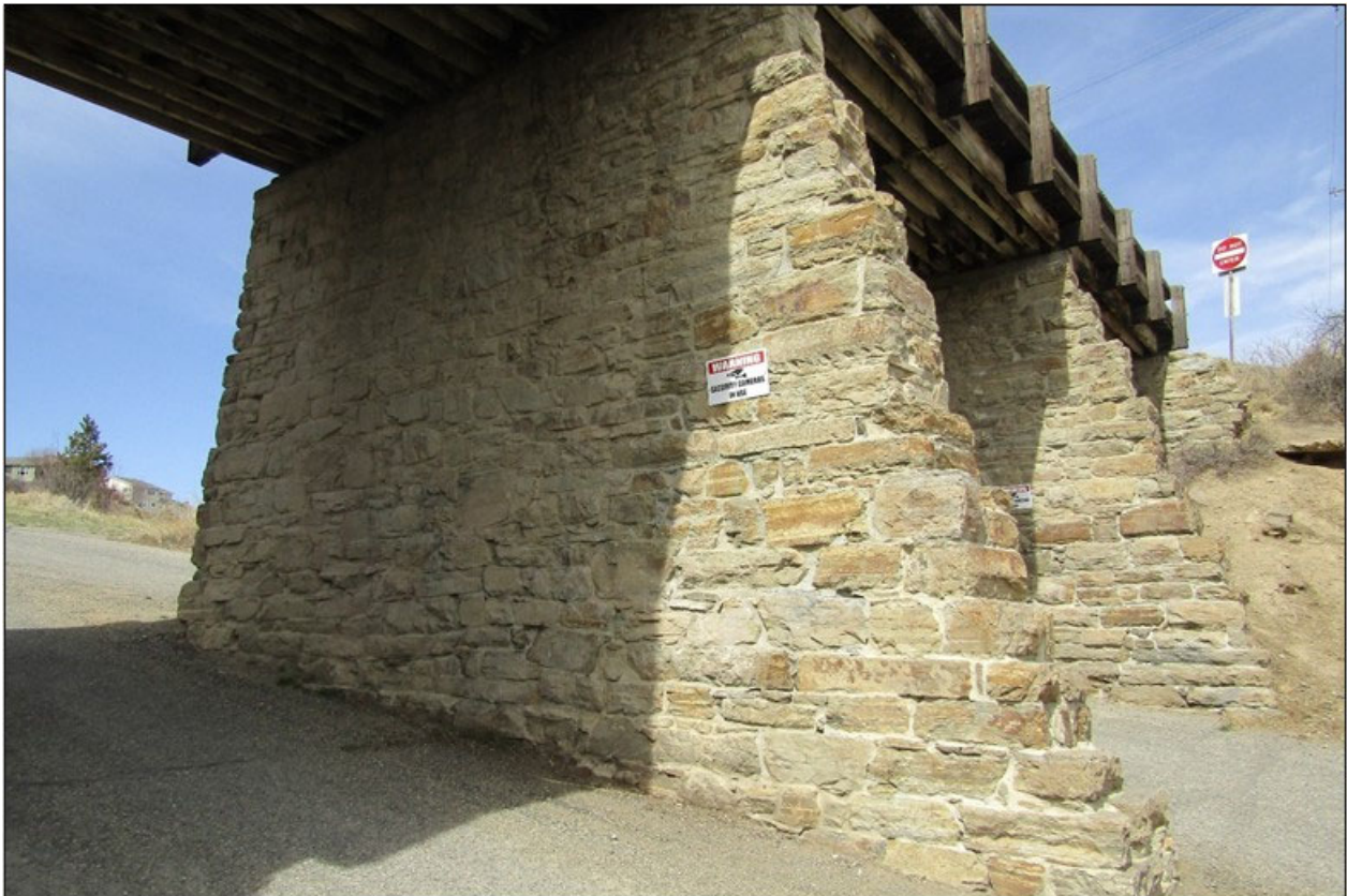
Morelli Bridge. Detail of rubblestone bents. View to the northwest. MT_LewisandClarkCounty_MorelliBridge_0010.
