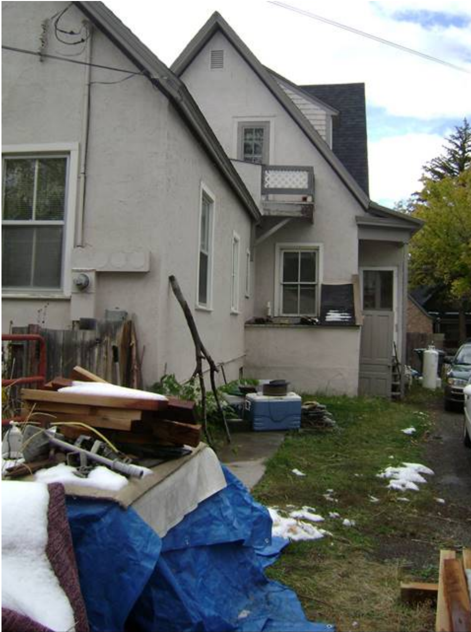
MT_LewisAndClark_Lyman-NeelResidence_0009: Lyman-Neel Residence. Two-Story Portion, East Elevation looking west.
