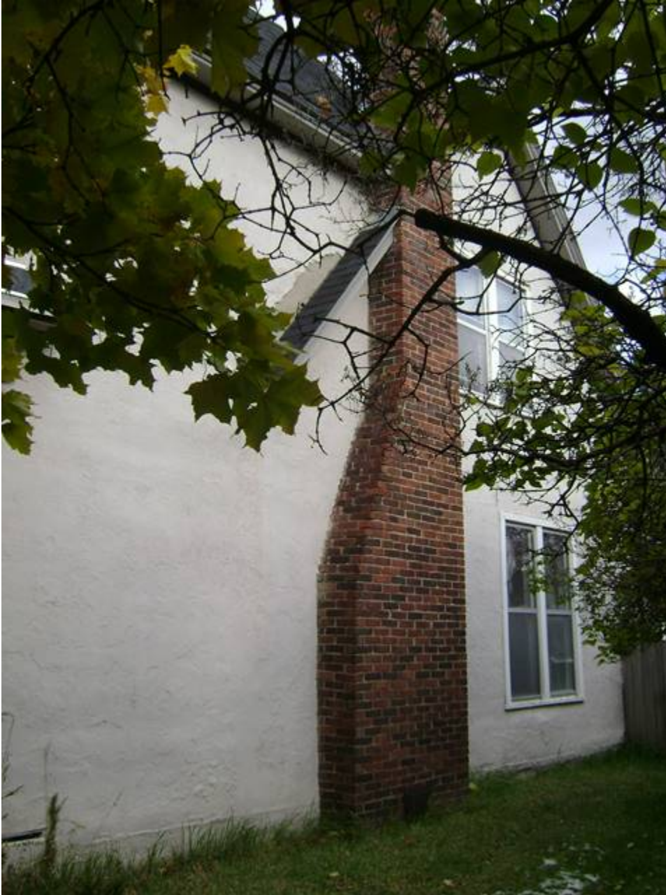
MT_LewisAndClark_Lyman-NeelResidence_0006: Lyman-Neel Residence. Two-Story South Elevation, looking northeast.
