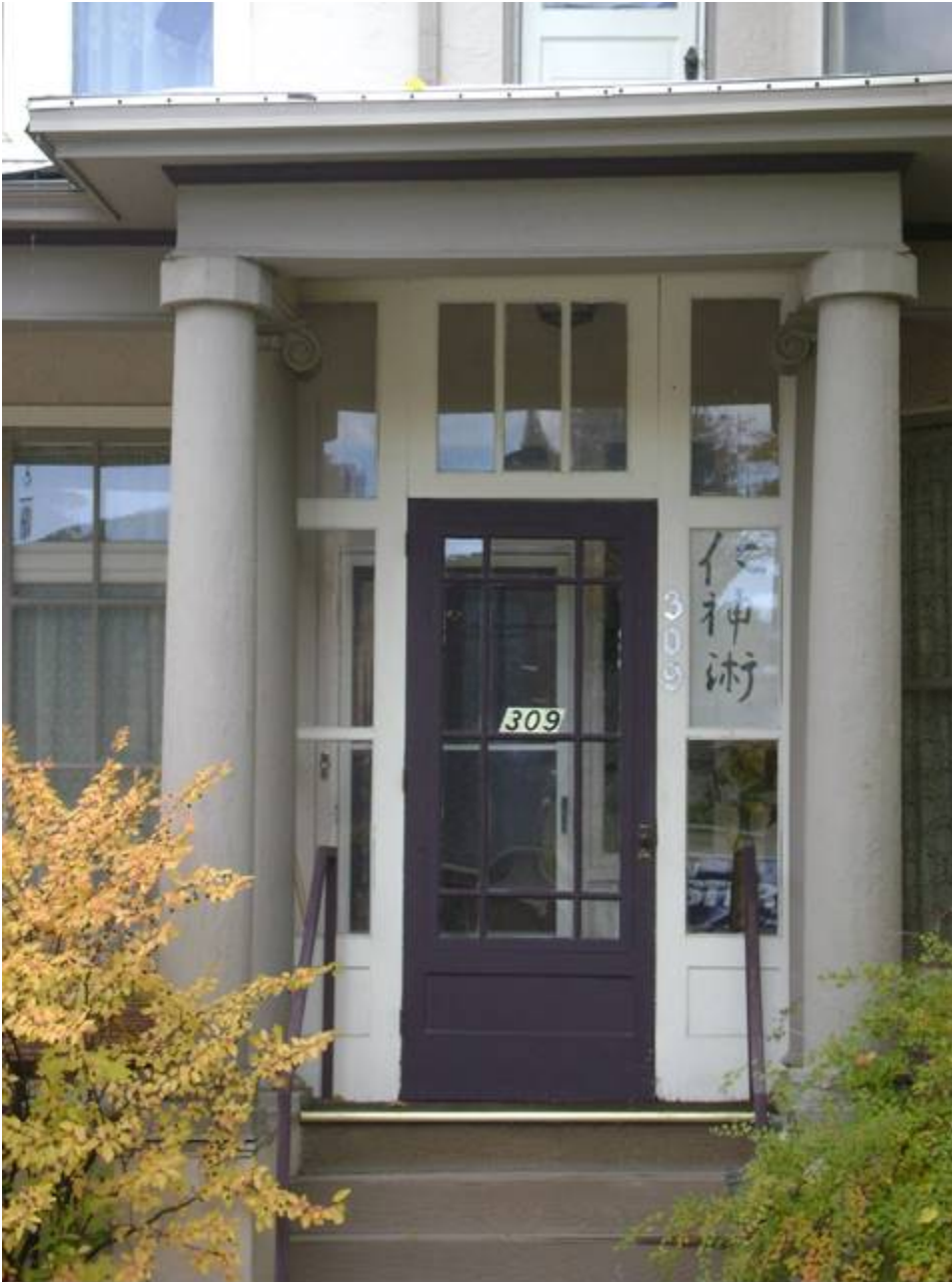
MT_LewisAndClark_Lyman-NeelResidence_0002: Lyman-Neel Residence. West Elevation looking east. Main entry
