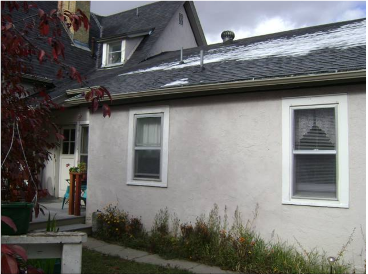
MT_LewisAndClark_Lyman-NeelResidence_0012: Lyman-Neel Residence. One-Story Addition, South Elevation, looking NW
