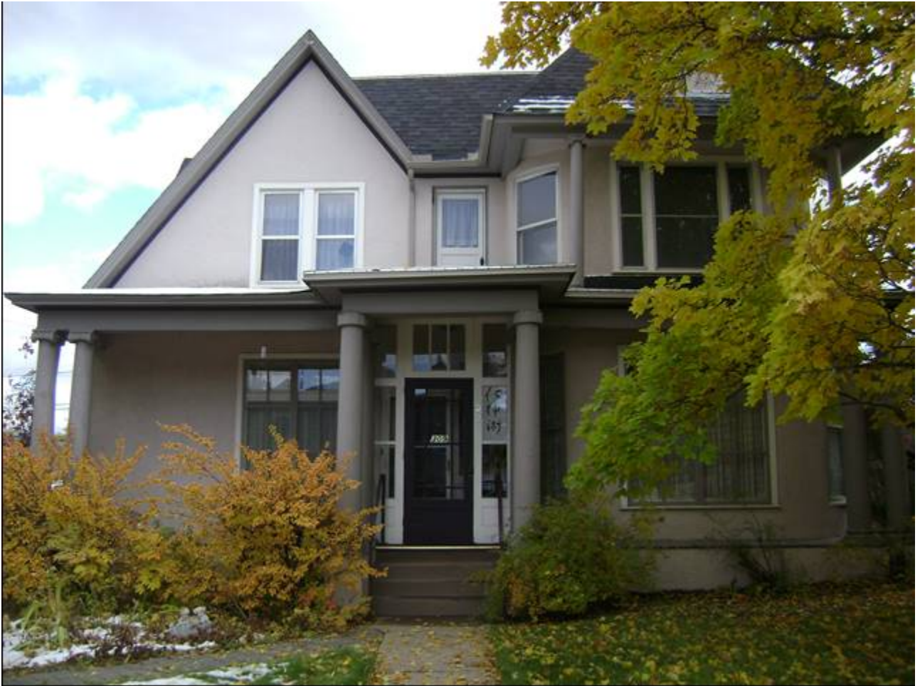
MT_LewisAndClark_Lyman-NeelResidence_0001: Lyman-Neel Residence. West Elevation looking east
