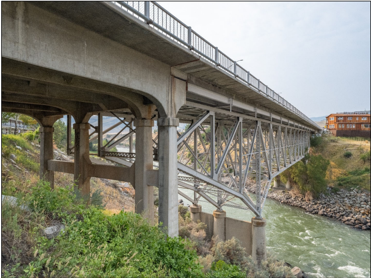
Gardiner Bridge. Detail of bridge. View to the south. MT_ParkCounty_GardinerBridge_0016.
