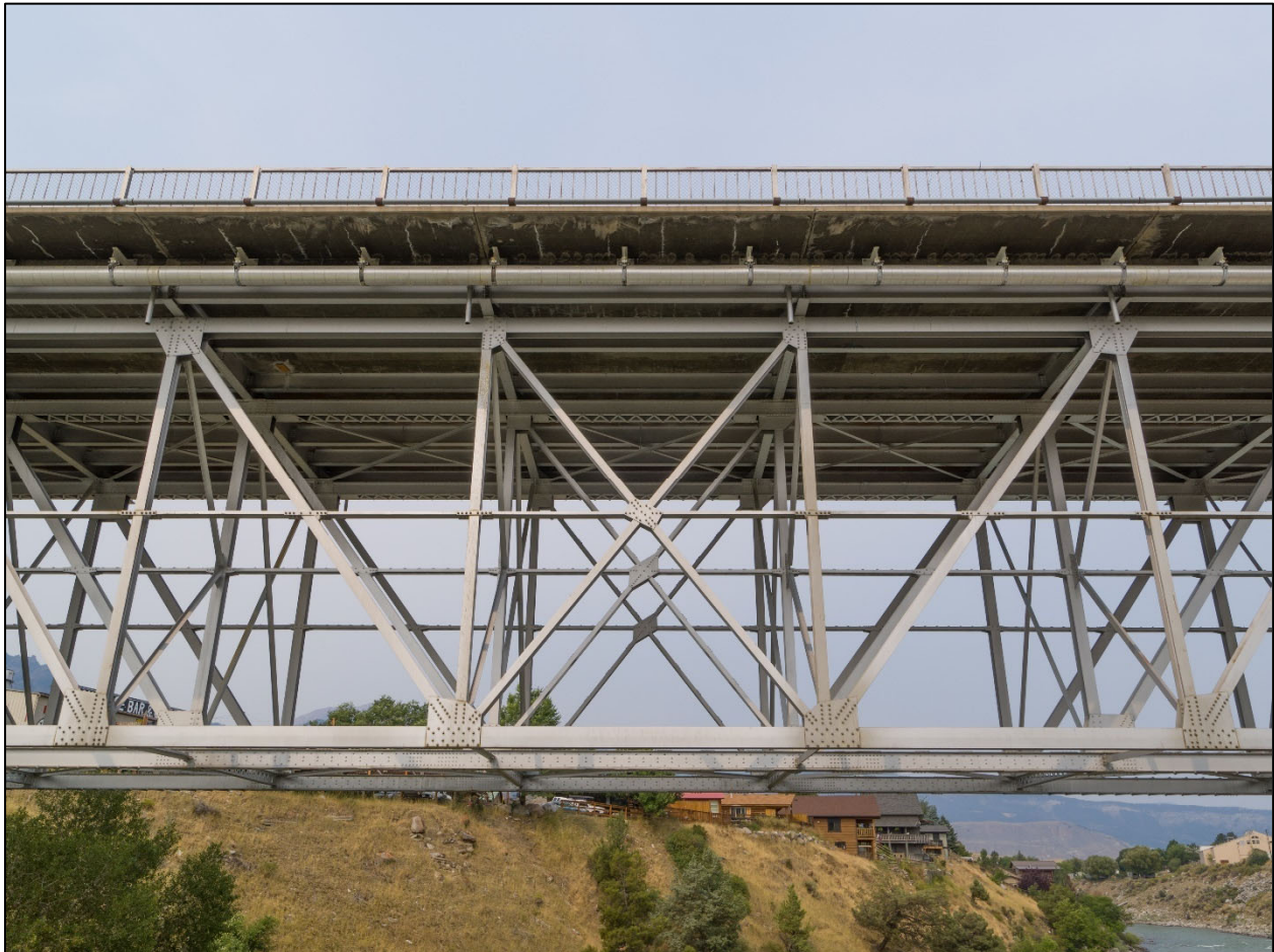
Gardiner Bridge. Detail of truss. View to the east. MT_ParkCounty_GardinerBridge_0017.
