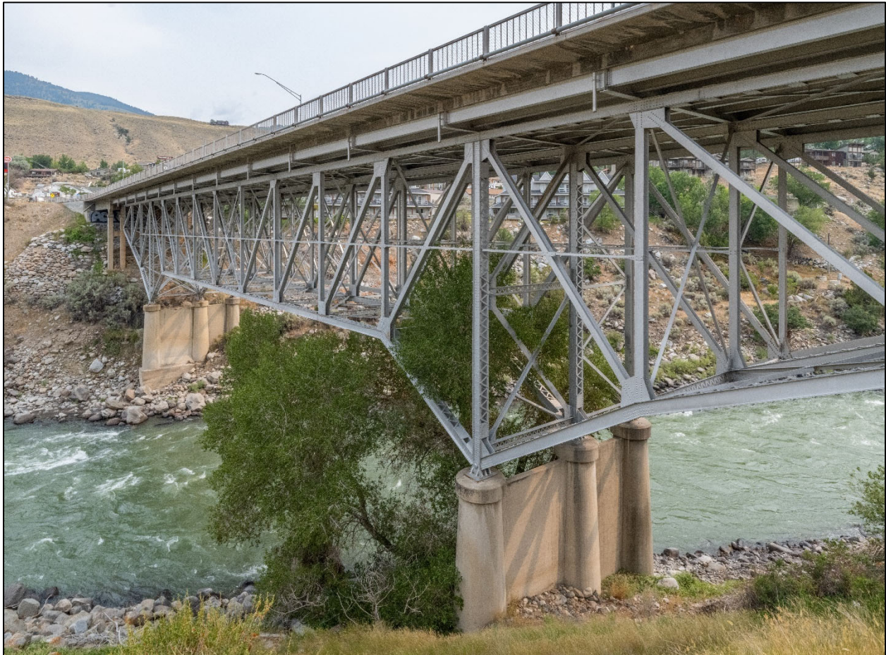
Gardiner Bridge. West side. View to north-northeast. MT_ParkCounty_GardinerBridge_0008.
