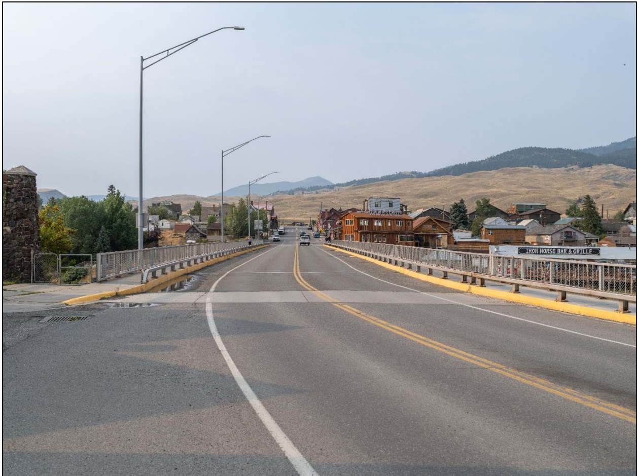
Gardiner Bridge. North approach. View to the south. MT_ParkCounty_GardinerBridge_0018.
