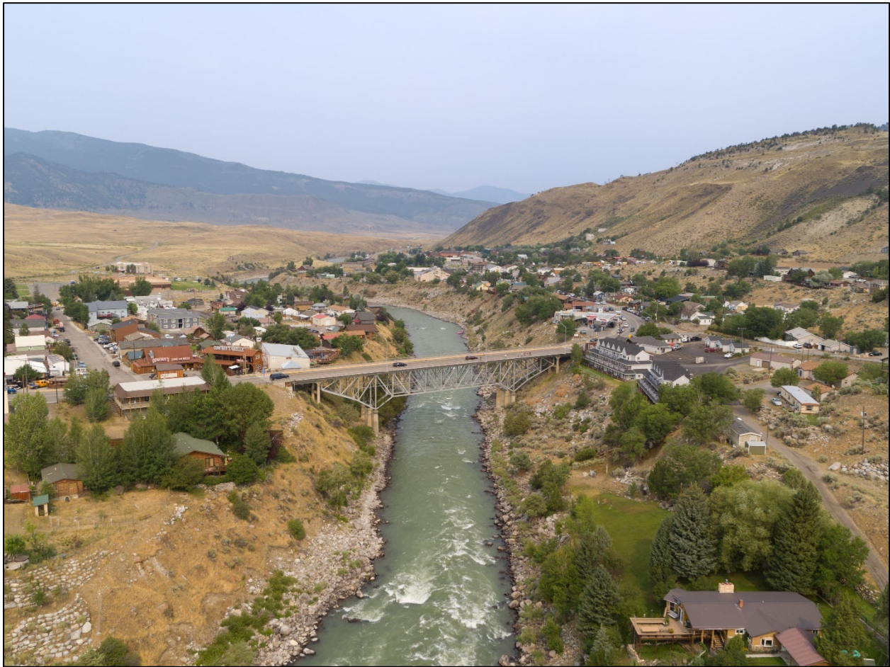
Gardiner Bridge. East side. View to the west. MT_ParkCounty_GardinerBridge_0005.
