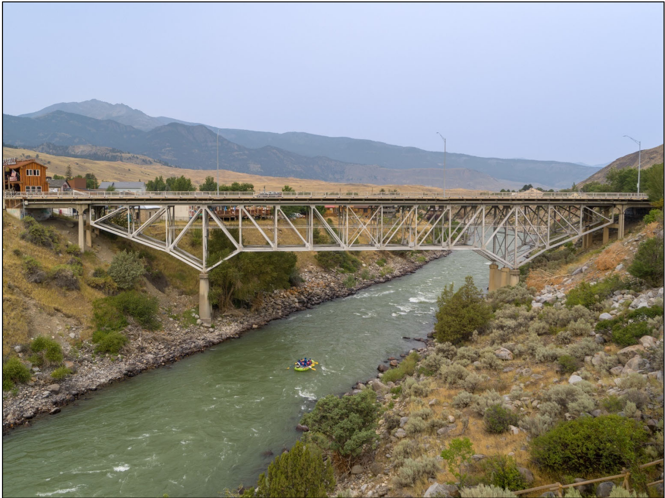
Gardiner Bridge. East side. View to west. MT_ParkCounty_GardinerBridge_0006.
