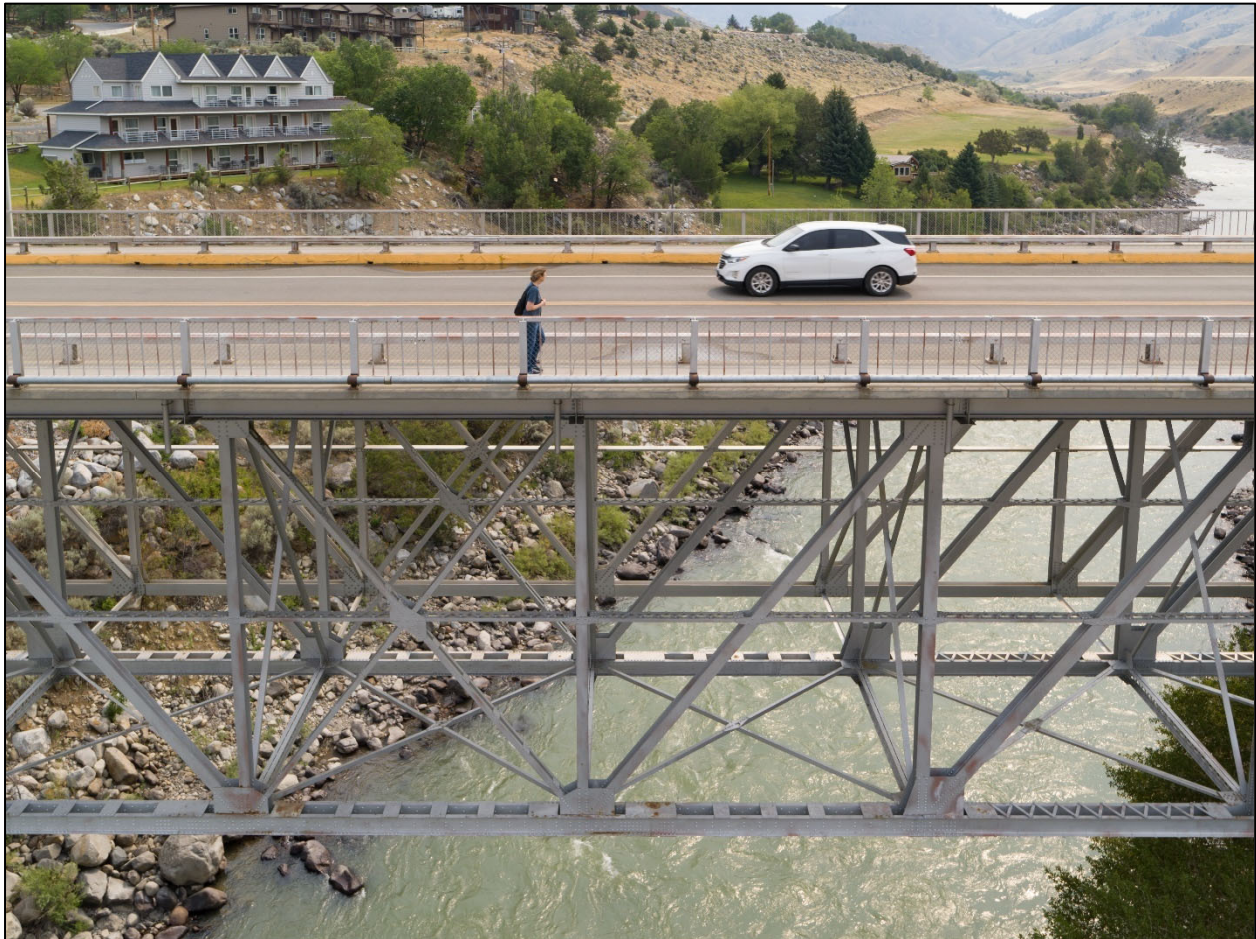
Gardiner Bridge. Detail of truss. View to the east. MT_ParkCounty_GardinerBridge_0012.
