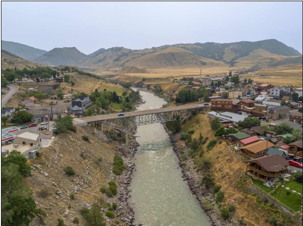
Gardiner Bridge. West side. View to east. MT_ParkCounty_GardinerBridge_0001
