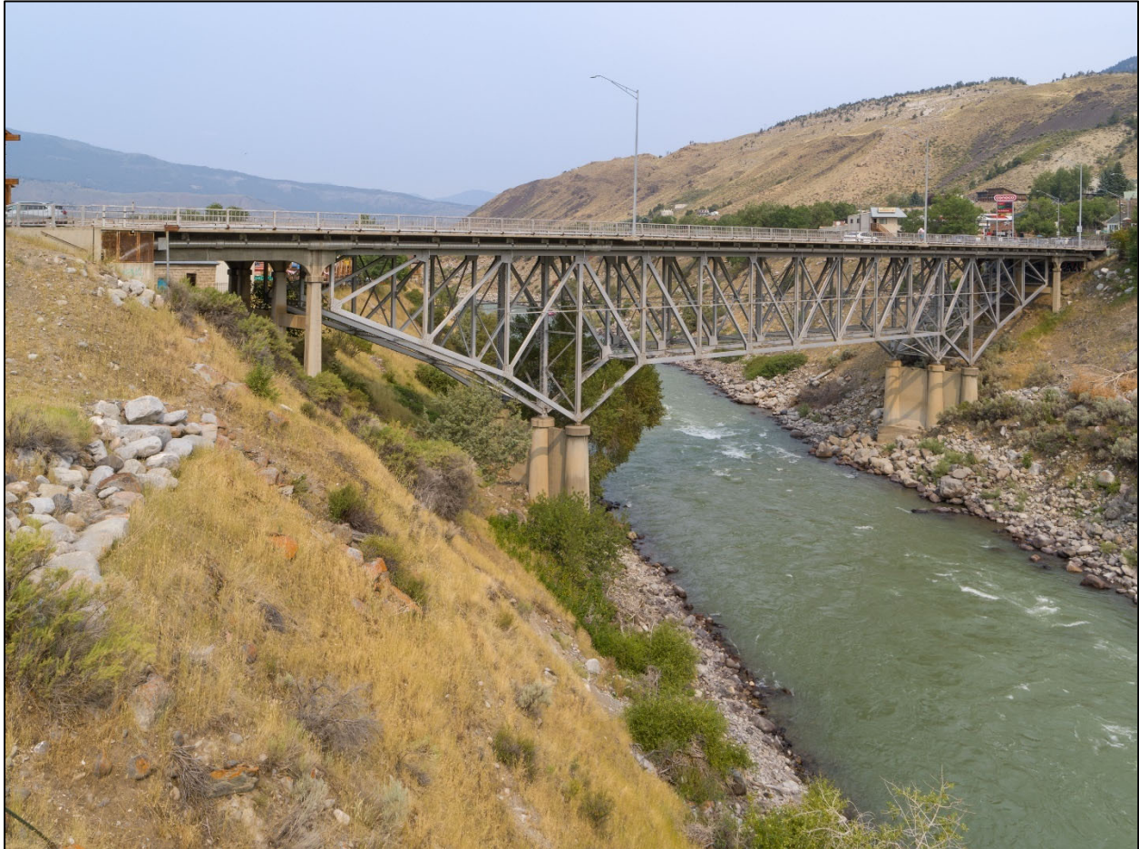
Gardiner Bridge. East side. View to west-northwest. MT_ParkCounty_GardinerBridge_0009.
