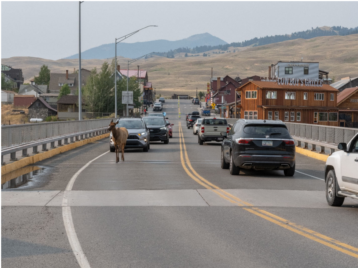
Gardiner Bridge. South approach with elk on bridge. View to the south. MT_ParkCounty_GardinerBridge_0019.
