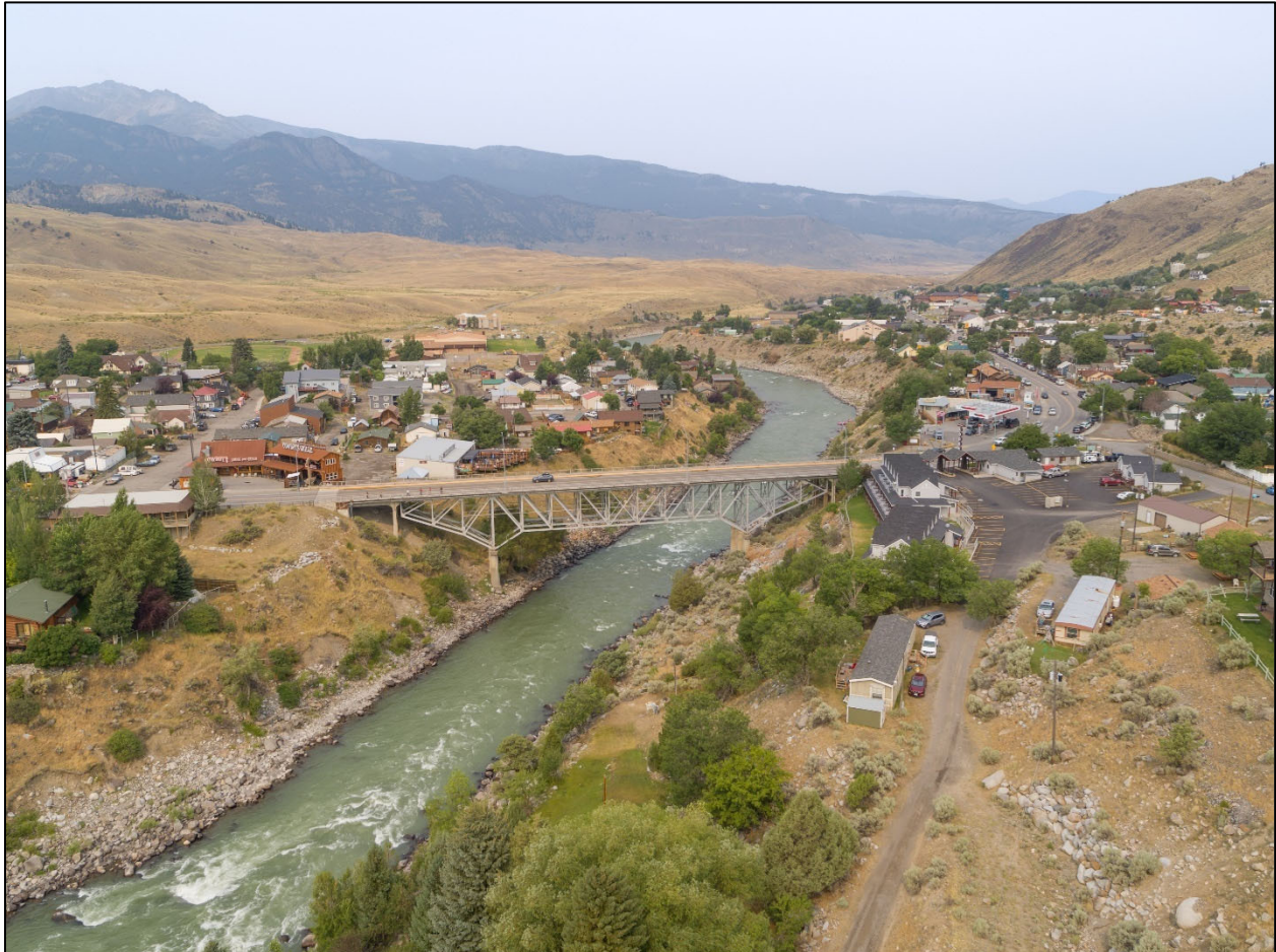
Gardiner Bridge. East side. View to west. MT_ParkCounty_GardinerBridge_0004.
