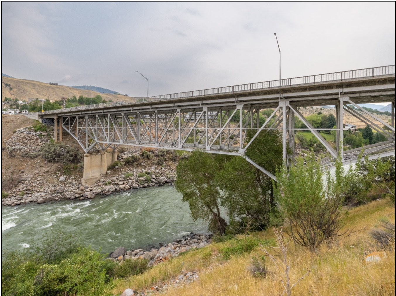
Gardiner Bridge. West side. View to the northeast. MT_ParkCounty_GardinerBridge_0007.
