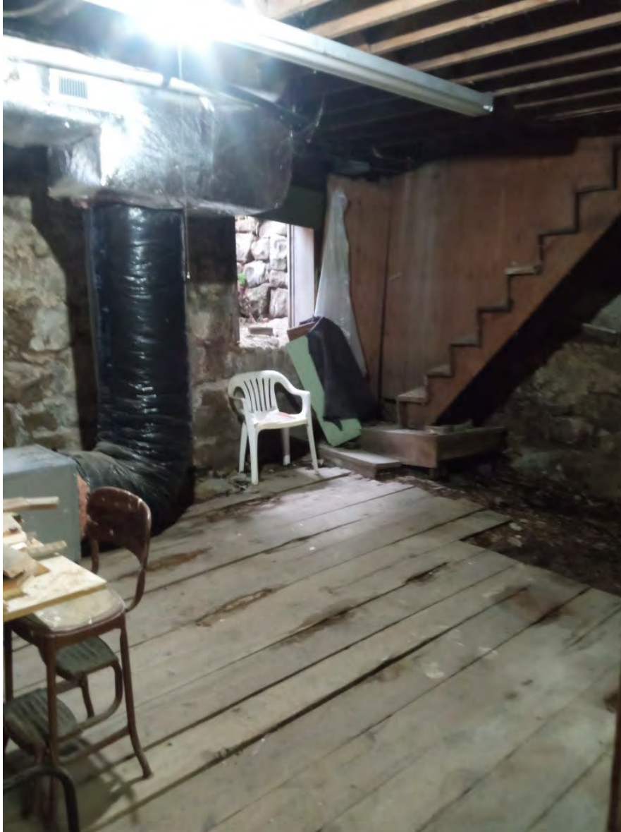
Basement of Farmers Trading Company showing staircase, view to Northwest
