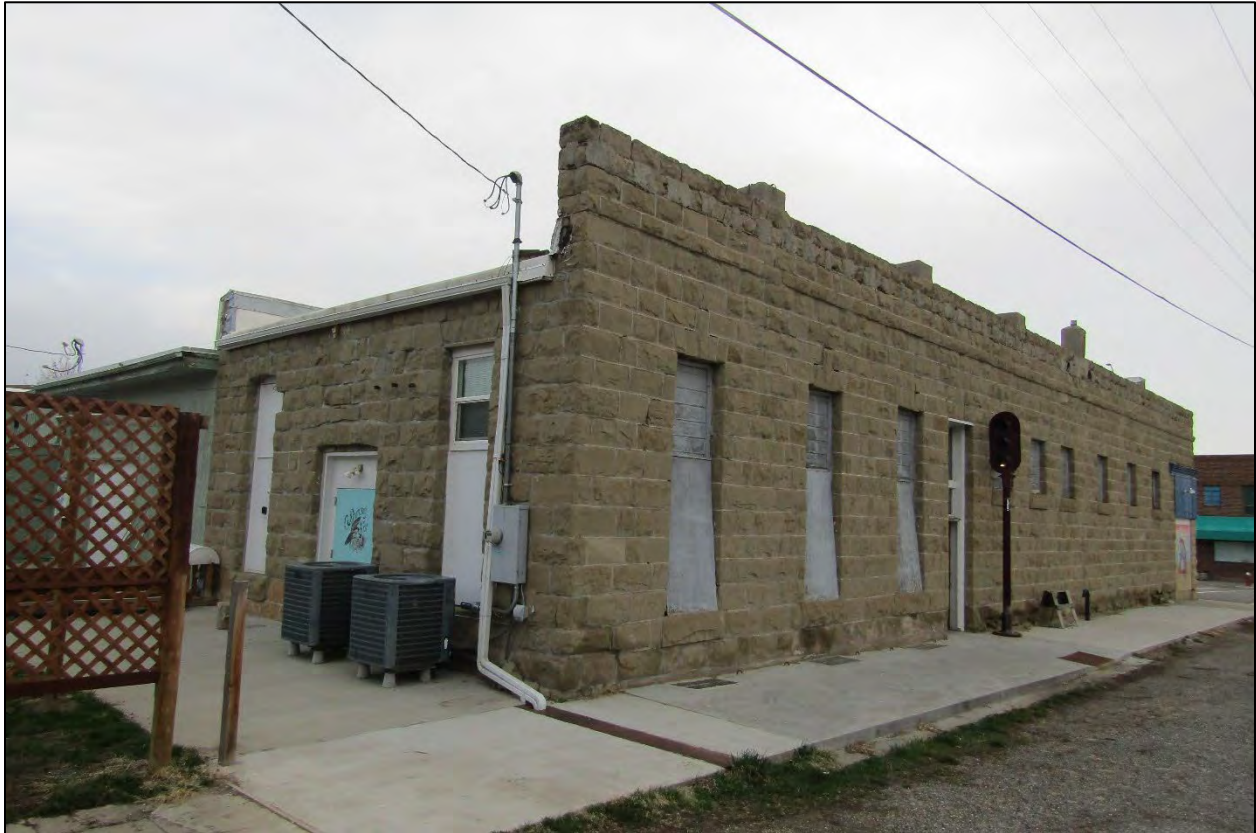
Farmers Trading Company. South side and rear facade. View to northeast. MT_CarbonCounty_FarmersTradingCompany_0004.
