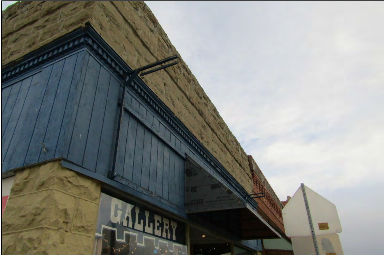
Farmers Trading Company. Detail of facade. View to north-northwest. MT_CarbonCounty_FarmersTradingCompany_0009.
