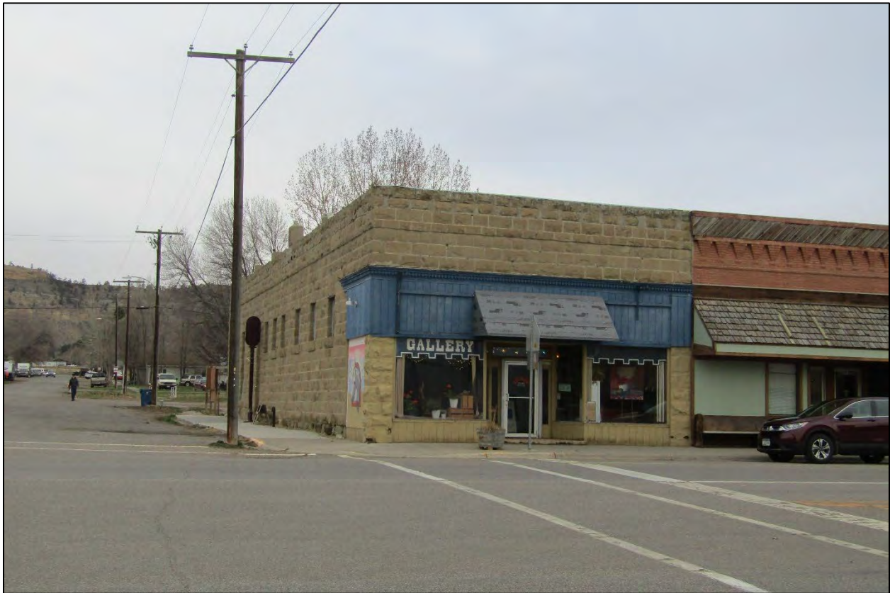
Farmers Trading Company. Façade and south side. View to west. MT_CarbonCounty_FarmersTradingCompany_0001
