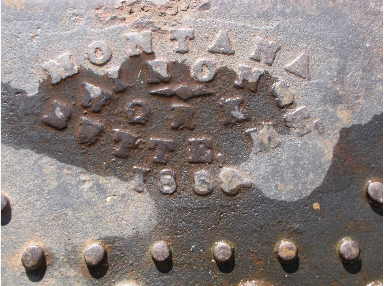
MT_DeerLodge_DriversSaloonCafe_004. Detail of the iron storefront with maker's mark "Montana / Iron Works / Butte, MT. / 1888"
