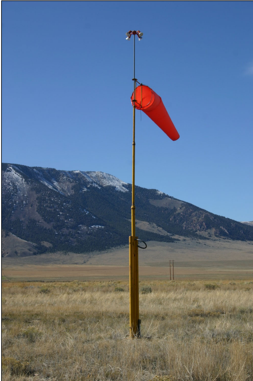
MT_BeaverheadCounty_DellFlightStrip_0018. Lighted wind cone, view to northwest.
