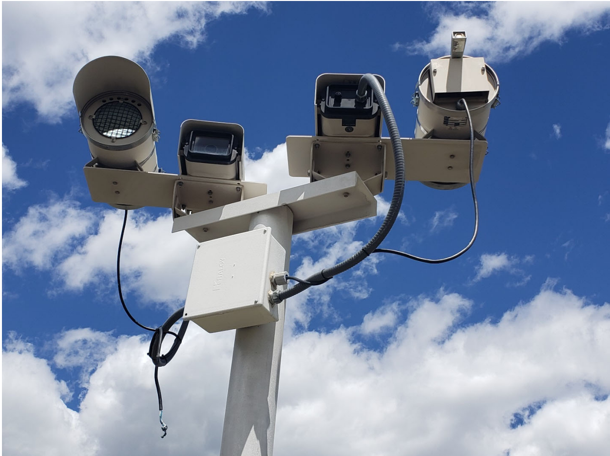
MT_BeaverheadCounty_DellFlightStrip_0025. Close up of Modern PAPI.
