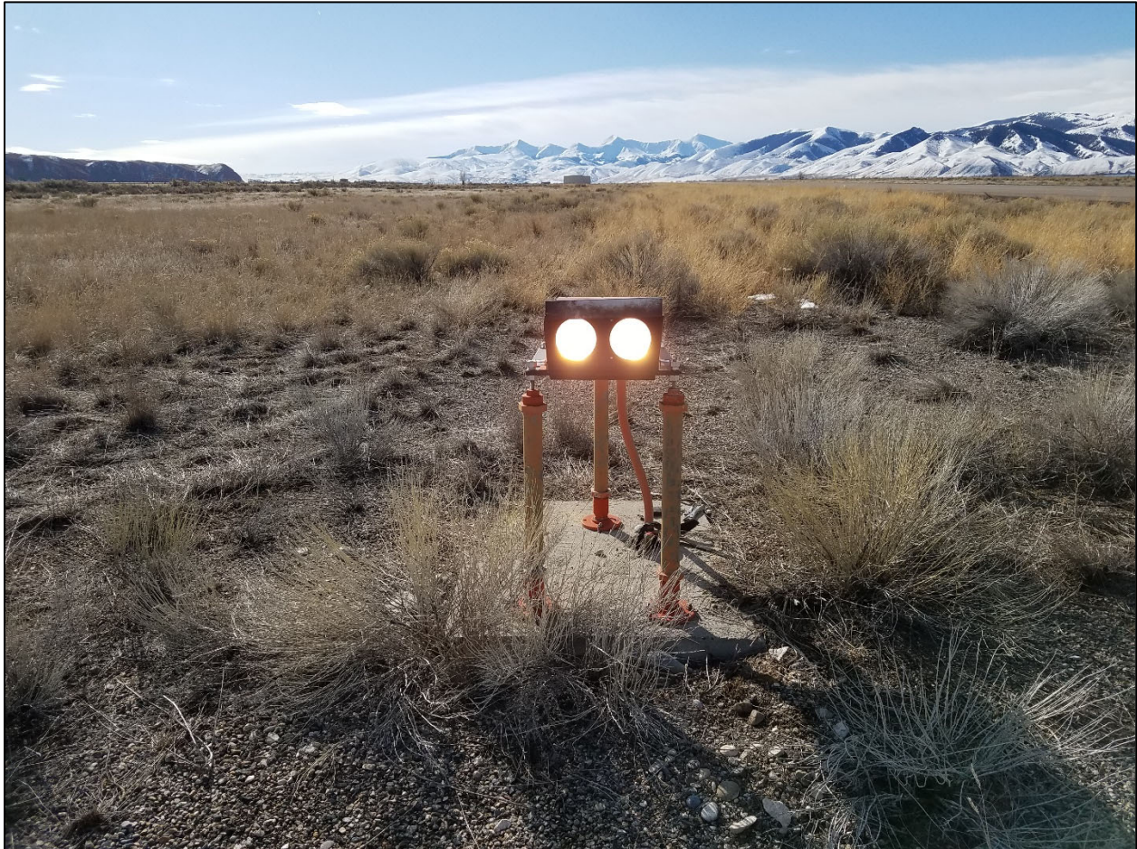
MT_BeaverheadCounty_DellFlightStrip_0019. Original Precision Approach Path Indicator (PAPI), view to south.
