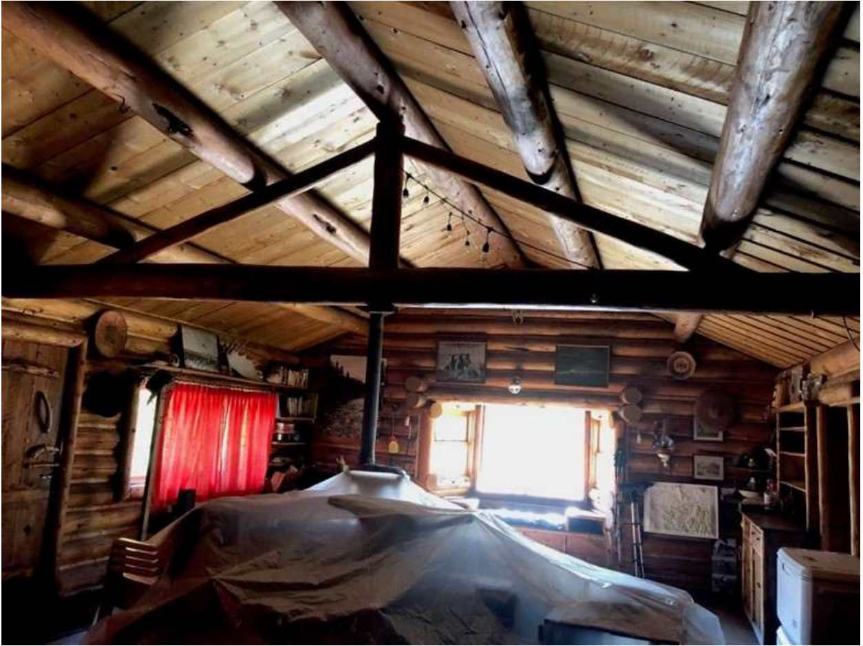
MT_ParkCounty_HerbertSummerCabin_0009. Main Cabin interior. View to south.
