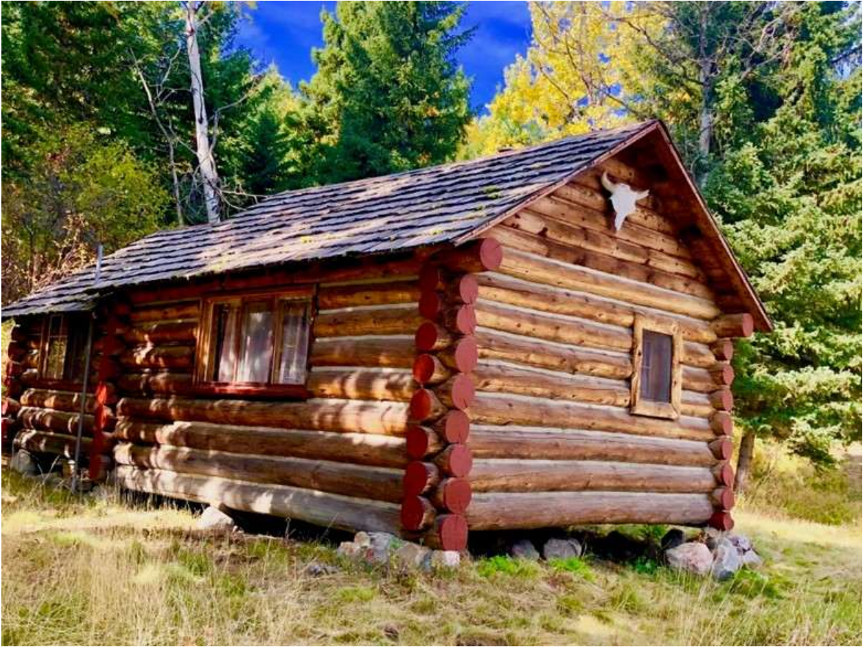
MT_ParkCounty_HerbertSummerCabin_0012. Guest Cabin, south and east walls. View to northwest.
