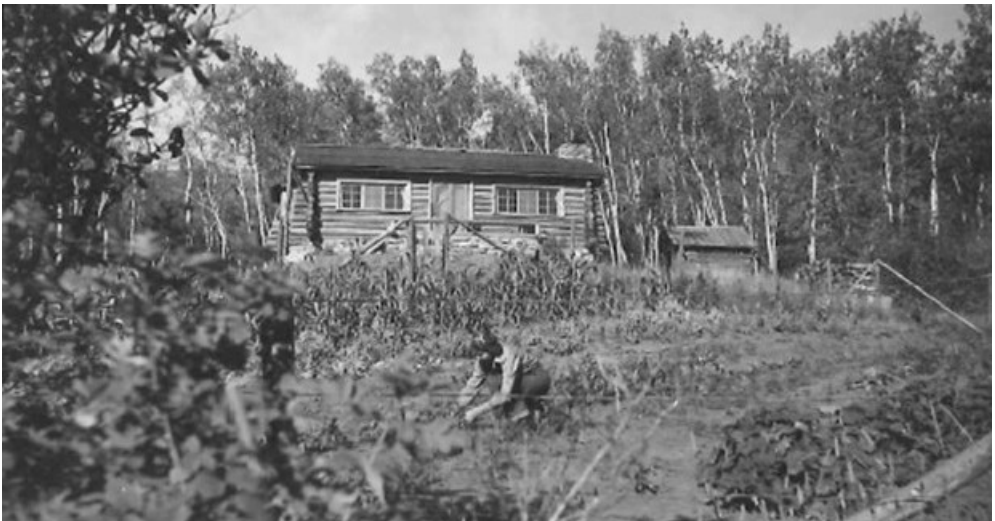
Main Cabin with garden in foreground, view to the west, circa 1935-1940.
