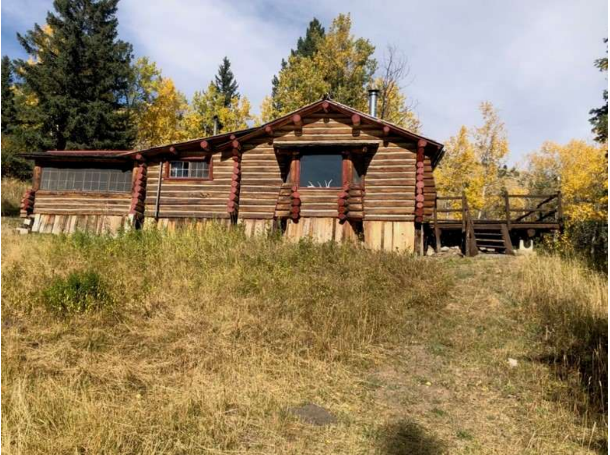
MT_ParkCounty_HerbertSummerCabin_0006. Main Cabin, south wall and deck. View to north.
