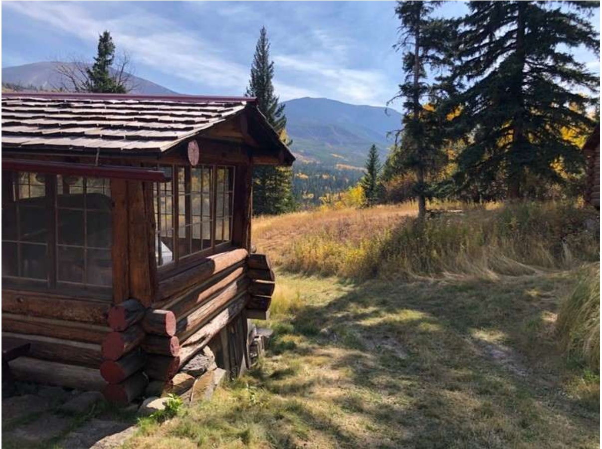
MT_ParkCounty_HerbertSummerCabin_0002. View to south.
