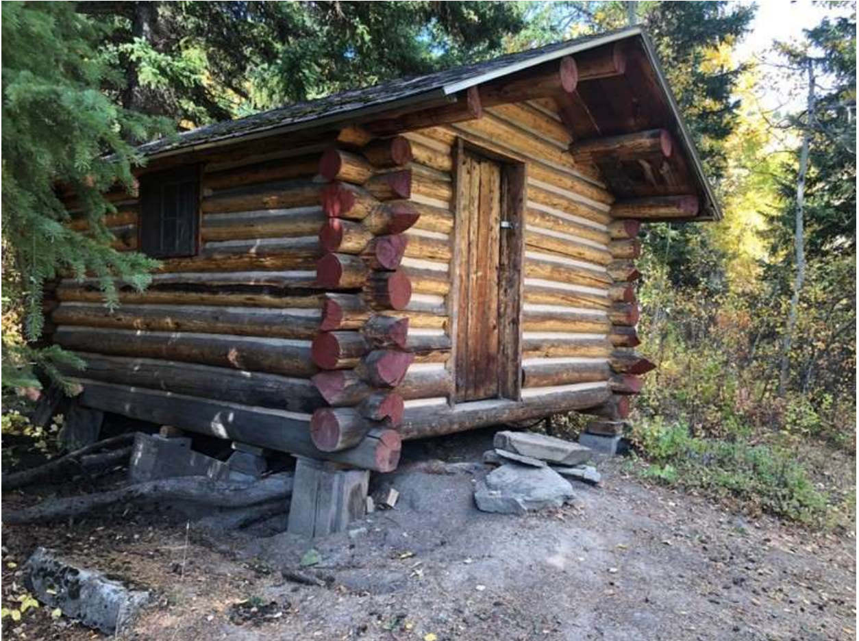
MT_ParkCounty_HerbertSummerCabin_0015. Sleeping Cabin, south and east walls. View to northwest.
