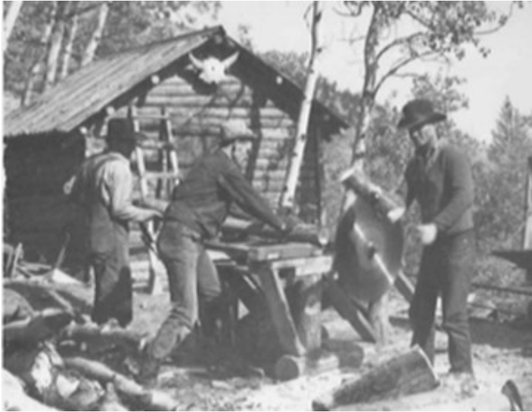
Men at work in front of Sleeping Cabin, view to the northwest, circa 1935.
