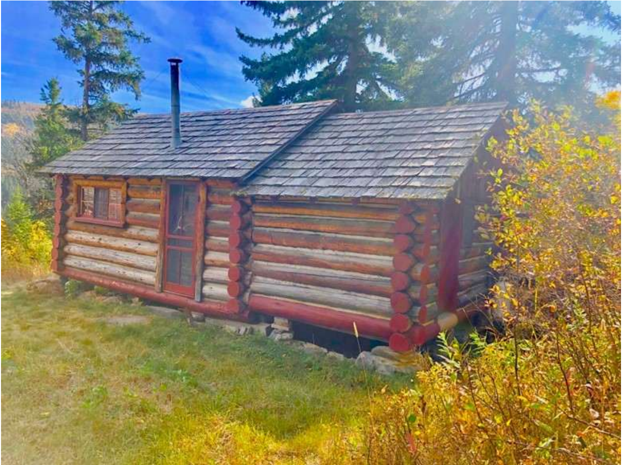
MT_ParkCounty_HerbertSummerCabin_0011. Guest Cabin, north and west walls. View to south.
