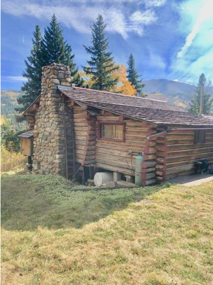
MT_ParkCounty_HerbertSummerCabin_0005. Main cabin, north wall. View to southeast.
