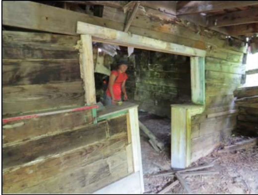
MT_CascadeCounty_AlbrightHD_0031. Feature AB-011, interior of addition to building in 2020 where the original window has been modified to create a doorway. View direction northwest. (Photographer: Preserve Montana)
