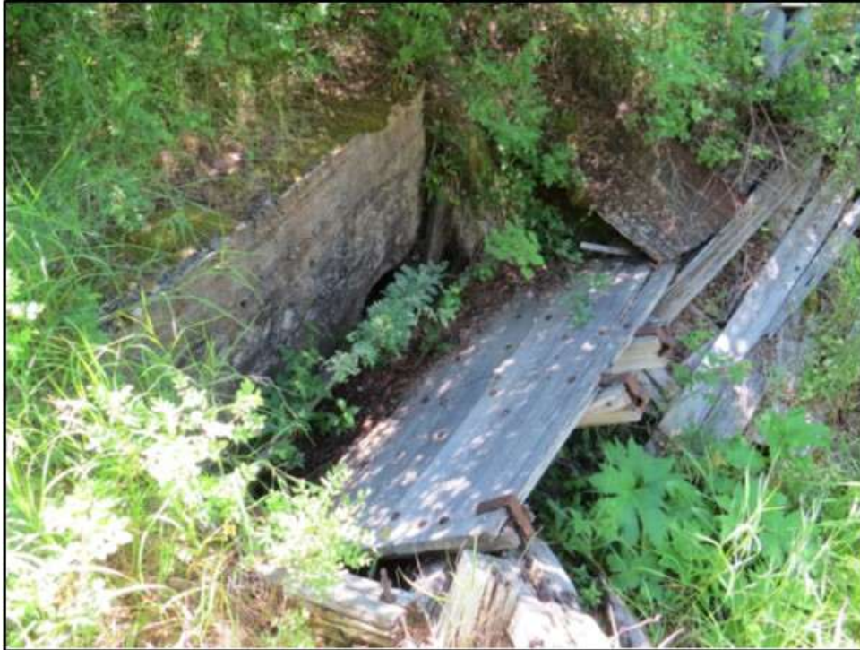
MT_CascadeCounty_AlbrightHD_0073. Feature AB-035 dam with wooden head gate leading to turbine house, in 2020. View direction southwest. (Photographer: Preserve Montana)
