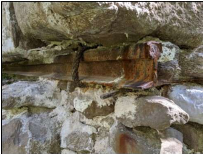
MT_CascadeCounty_AlbrightHD_0056. Feature AB-021 stone pier embedded rail with wrapped cable in 2020. View direction northeast. (Photographer: Preserve Montana)
