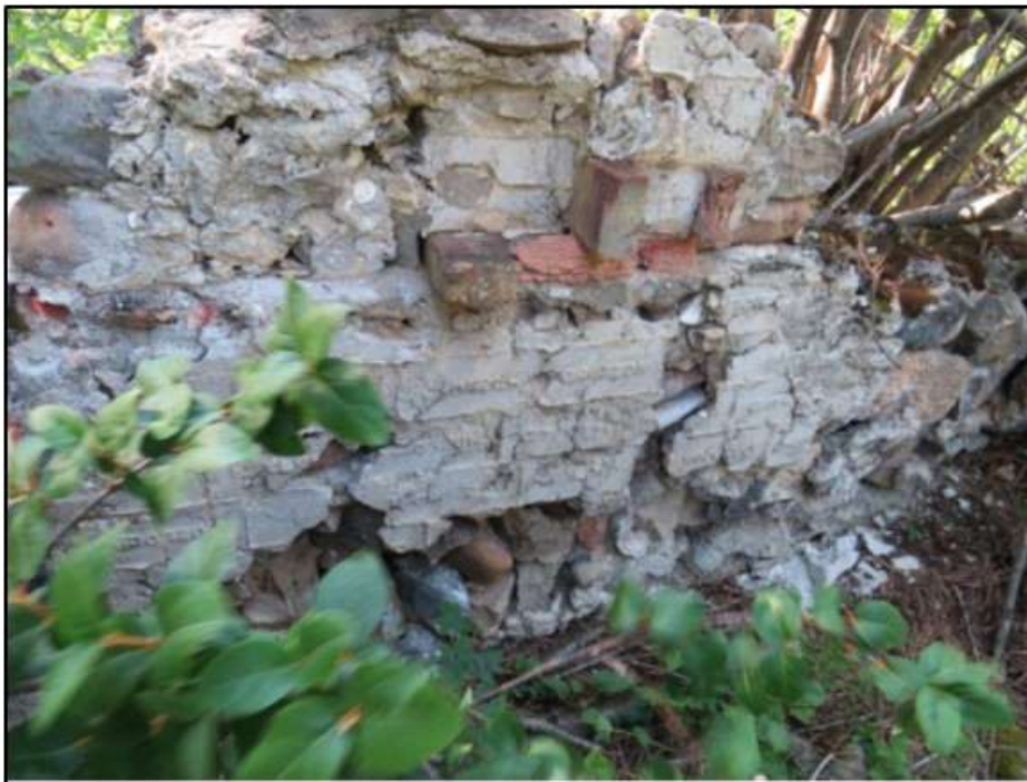
MT_CascadeCounty_AlbrightHD_0052. Feature AB-020 masonry detail showing the HOSSFORD imprints in the mortar in 2020. View direction unknown. (Photographer: Preserve Montana)
