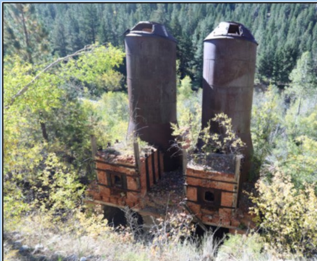
Albright Historic District, Cascade County
