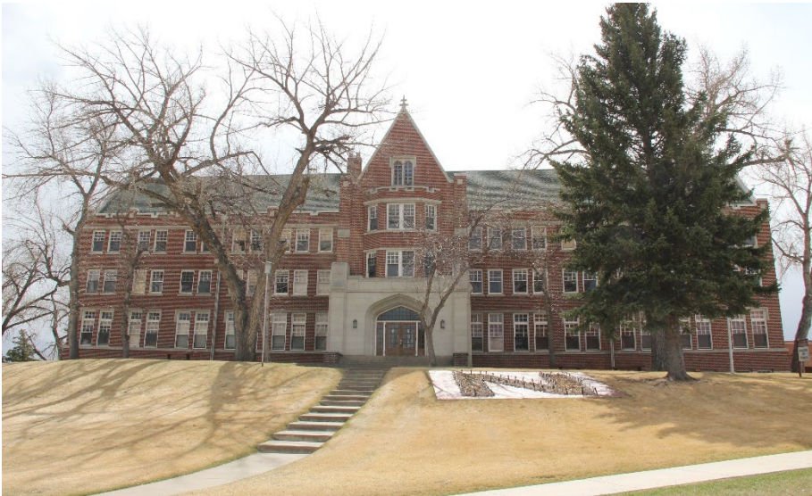
Figure 2: MSU-Northern's Donaldson Hall, north elevation. Photograph by Becki D. Miller, 07 April 2021.
