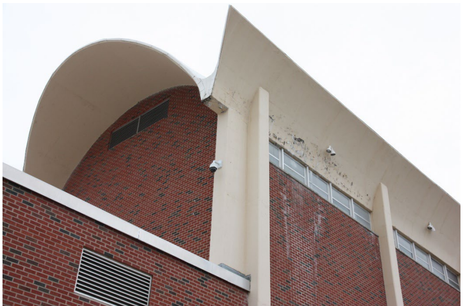
Figure 4: Physical Education Building (Alterowitz) at MSU-Billings. January 2020.
