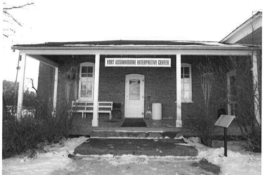
Figure 22: Fort Assiniboine, Post Library (c.1889), previously used for offices by NARC. The building is now used as an interpretive center. Photograph taken January 22, 2020.
