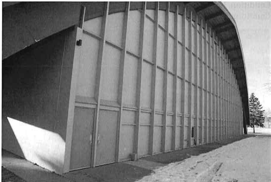
Figure 12: MSU-Northern's gymnasium - south curtain wall of wood. Photograph taken January 23, 2020.
