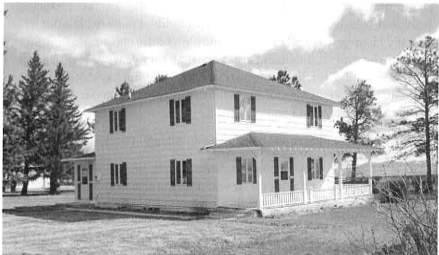
Figure 9: Farmstead House (Building #4403) at the Central AG Research Center in Moccasin. Photograph provided by MSU (powerpoint), dated 2011.
