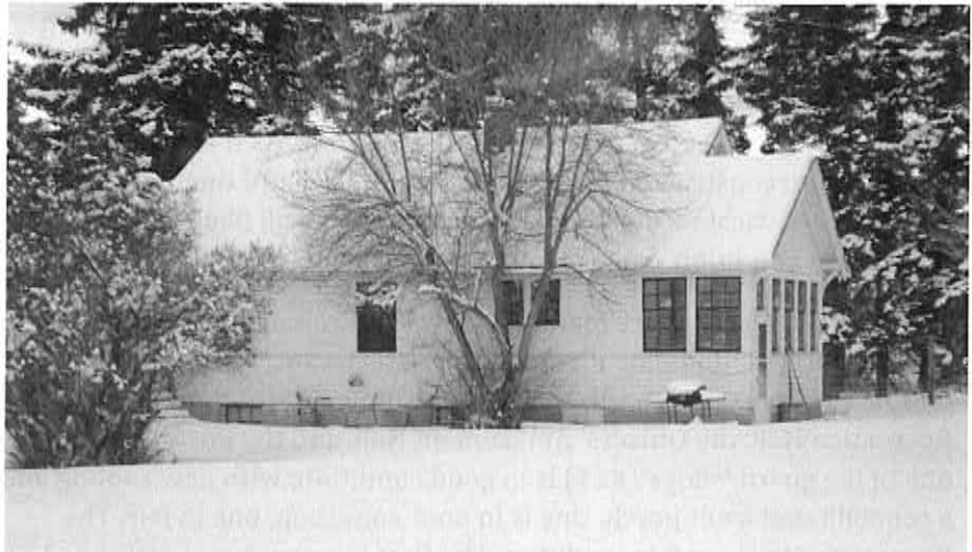
Figure 21: Fort Ellis, Ranch House No. 1 (Building# 721), as designed by Shanley, Willson & Hugenin in 1931. Photograph provided by MSU (powerpoint).
