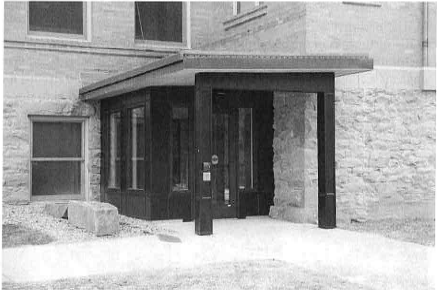
Figure 27: Montana Hall's newly constructed east exterior vestibule. Photograph taken January 26, 2020.
