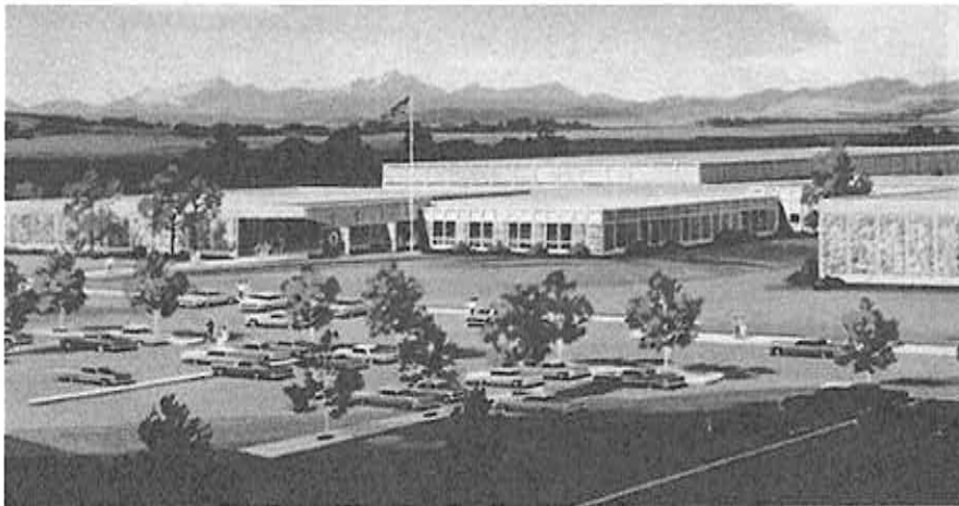
Figure 20: The sprawling building complex constructed for MSU-Great Falls in 1975. Rendering courtesy of http://gfcmsu.edu/about/history/index.html , accessed January 15, 2018.
