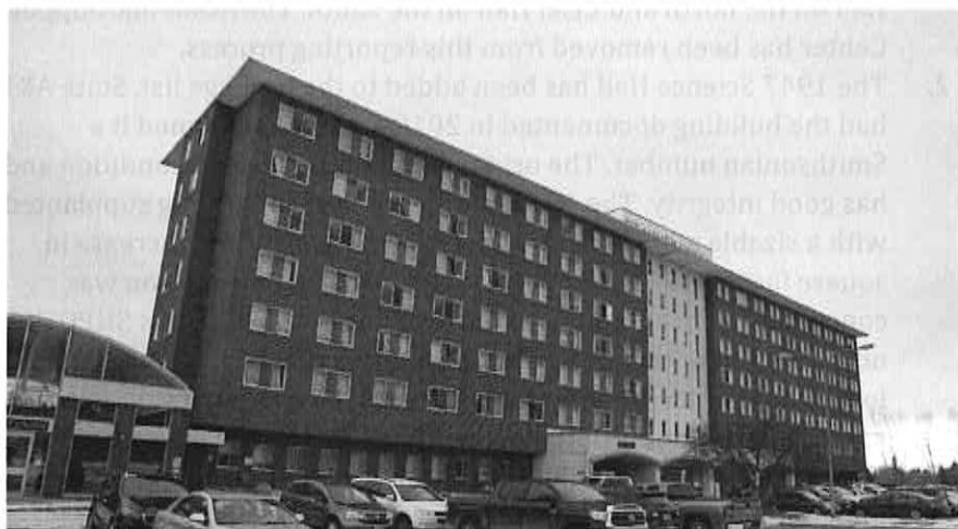
Figure 17: MSU-Billings' Petro Hall, constructed in 1966. Photograph (from the northeast) taken January 12, 2020.
