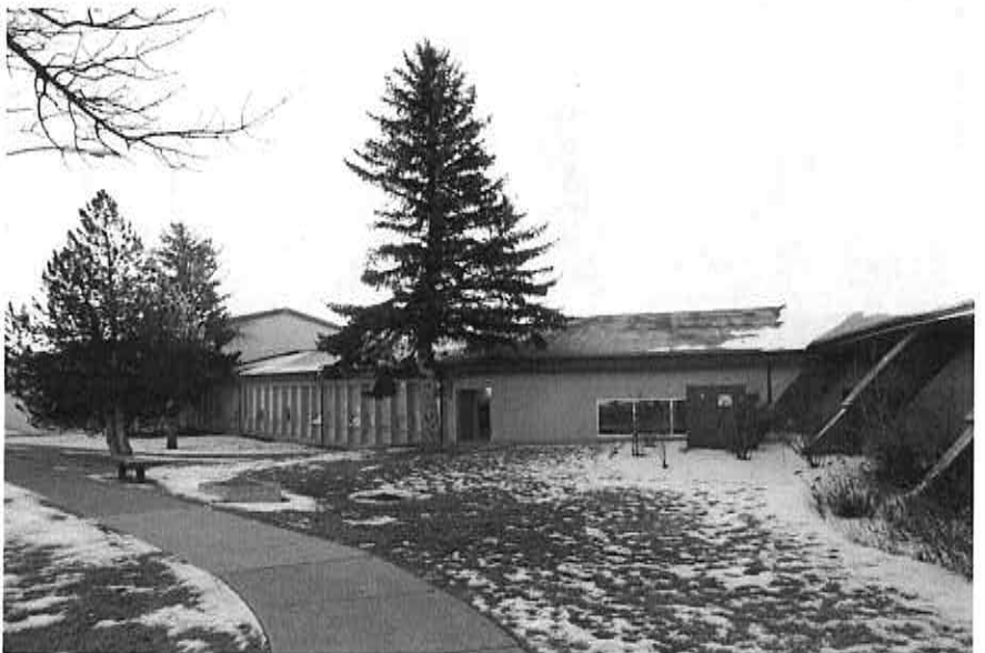
Figure 11: MSU-Northern's armory gymnasium, primarily at the right. The two left wings have been heavily modified. Photograph taken January 23, 2020.
