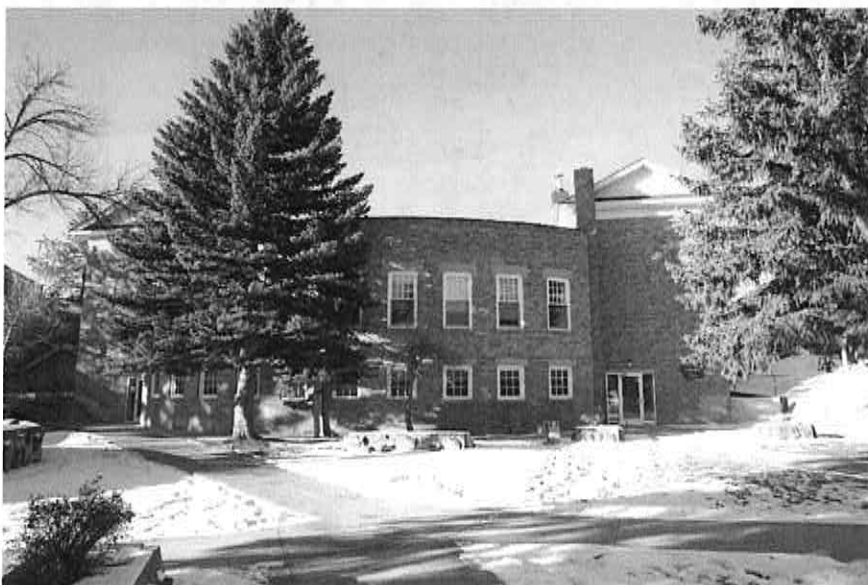
Figure 14: MSU-Northern's Pershing Hall, deemed a heritage resource in January 2020. Photograph taken January 23, 2020.
