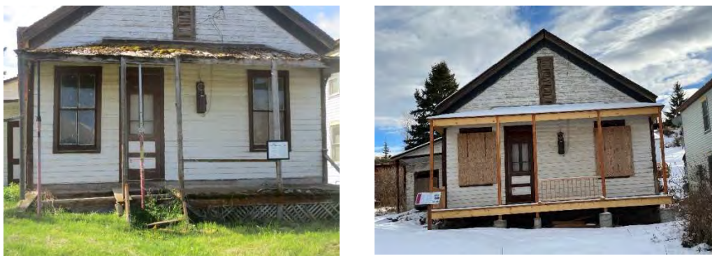
Hickman House masonry foundation and front porch stabilized – before and after (2023)
