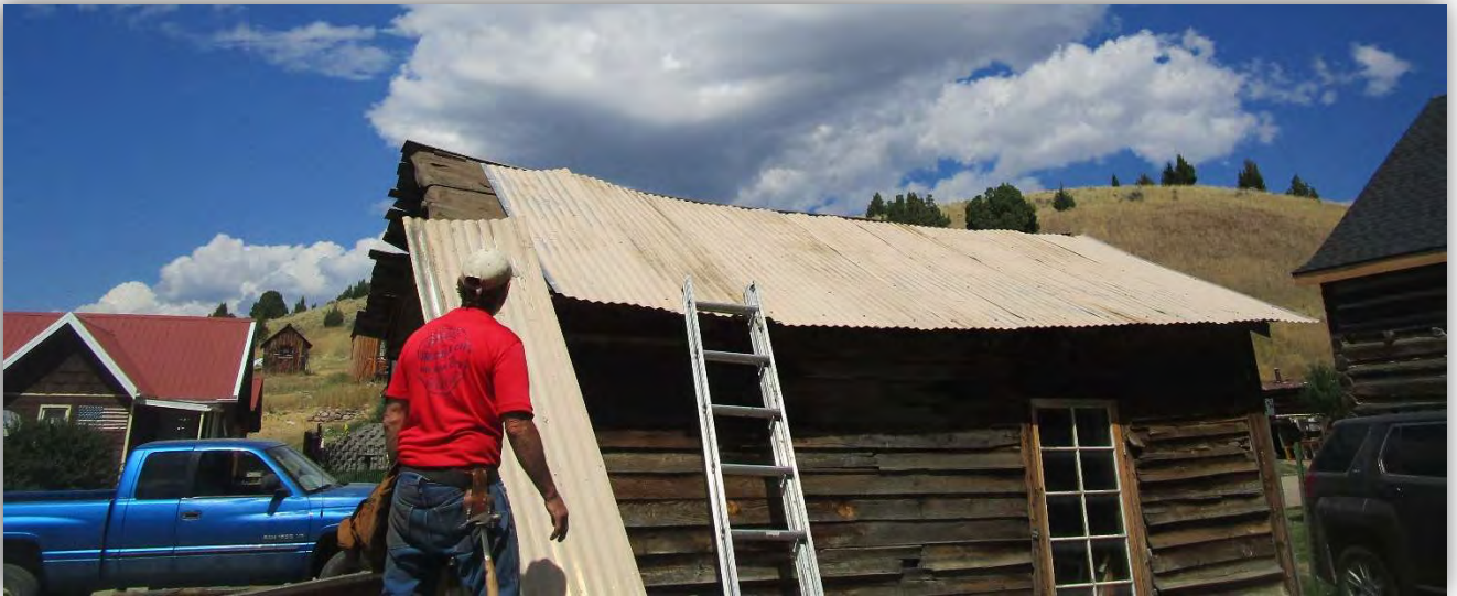
Historically sensitive roof repairs
