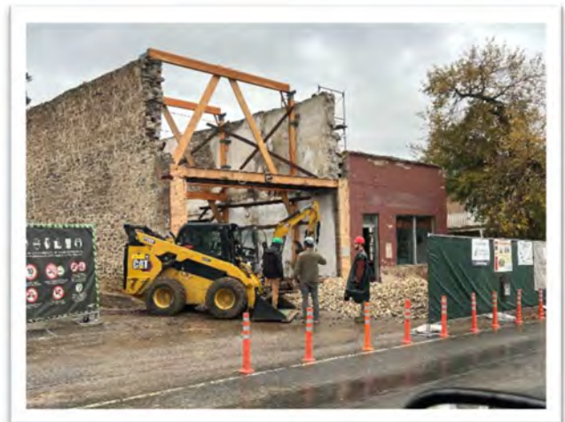
Stonewall Hall, preservation in process 1-2024
