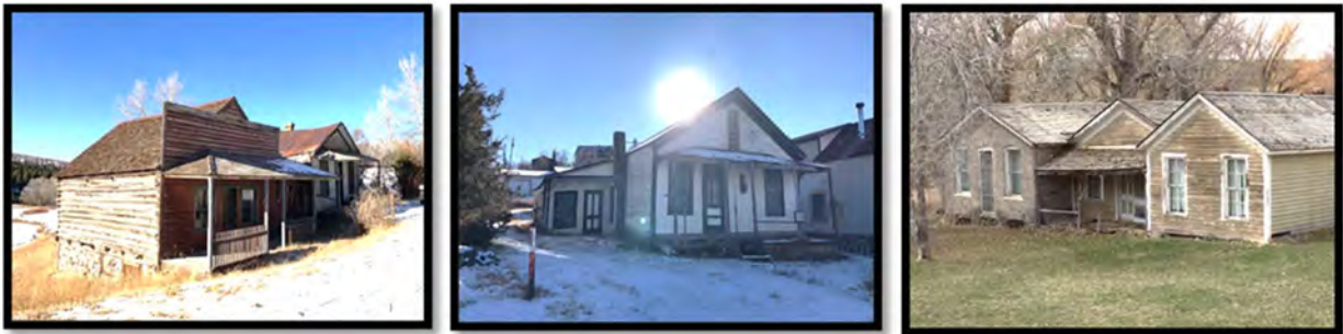
Coggswell-Taylor Cabin, Hickman House, and Gilbert House
