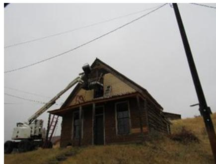
Figure 10: Harding House Exterior - siding replacement
