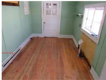
Figure 16: Smith Cabin - stabilize subfloor, install and finish new flooring; before and after
