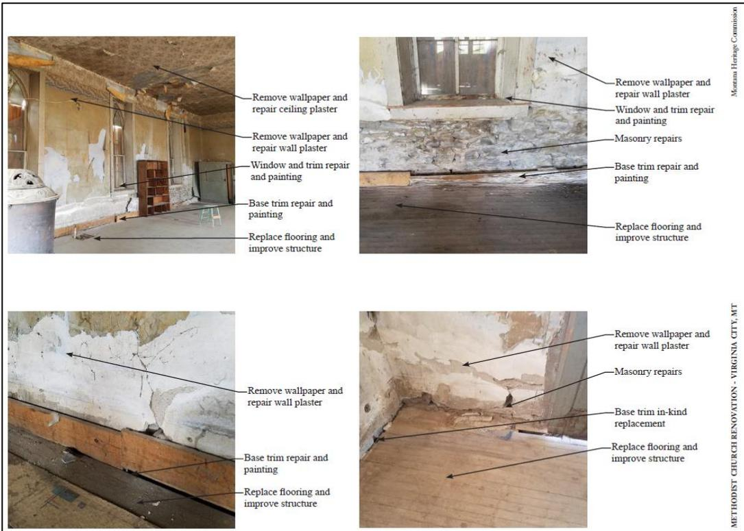
Figure 7 – Methodist Church - Scope of work (interior)
