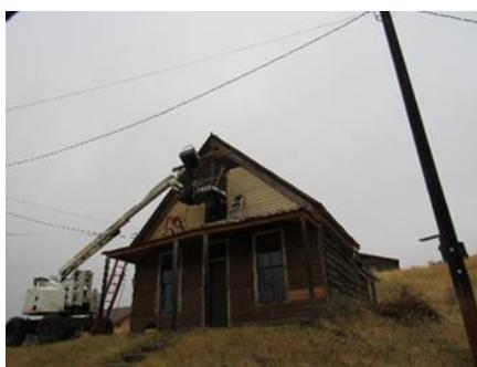
Figure 10: Harding House Exterior - siding replacement
