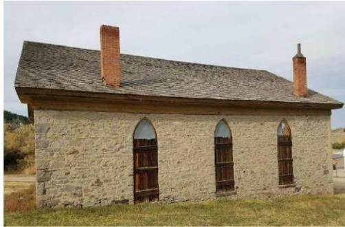
East Elevation: Stone masonry, unfinished wood windows, modified sliding wood door, decorative wood trim, and wood shingles.
