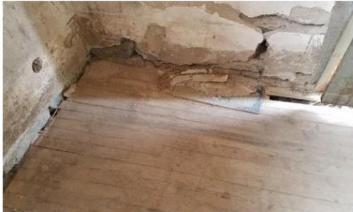
Water damage to flooring and masonry at sliding door. Gap open to exterior underneath door.
