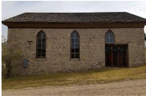
West Elevation: Stone masonry, unfinished wood windows, modified sliding wood door, decorative wood trim, and wood shingles.
