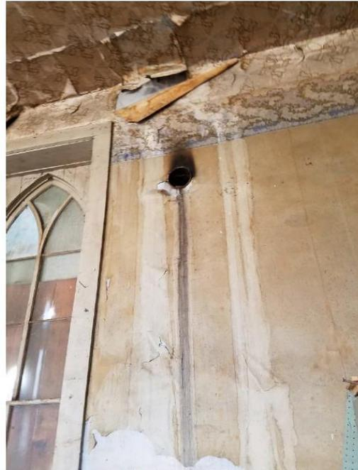
South window at east side and pipe for south chimney. Historic water damage observed beneath chimney.
