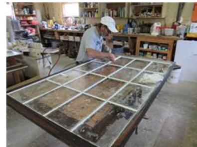
**Figure 1: Sauerbier Blacksmith Shop window – The brittle nature of old wood makes window repair a slow and delicate operation.**
