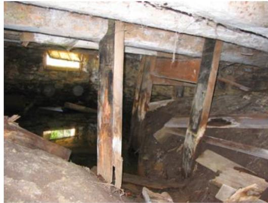
Figure 25: Gilbert House - basement subject to flooding leading to extensive interior moisture damage
