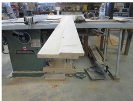
Figure 9: Harding House Exterior - siding re-fabrication
