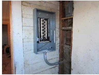
Figure 3: Harding House electrical panel – equipping old buildings with new utilities.
