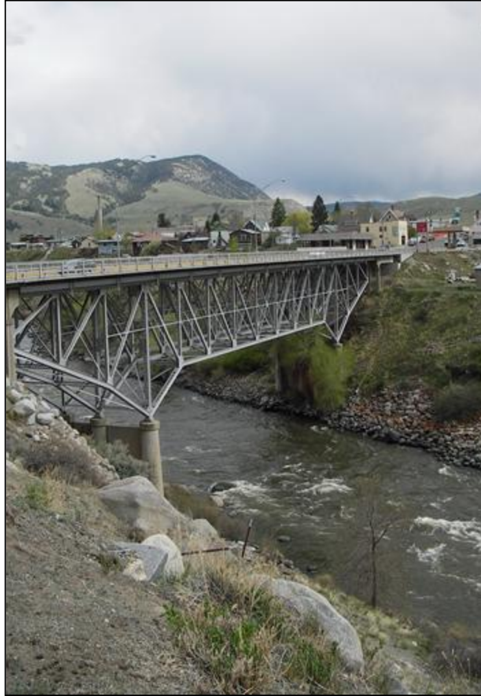
Figure 8. The Yellowstone River Bridge at Gardiner (24PA0790)
