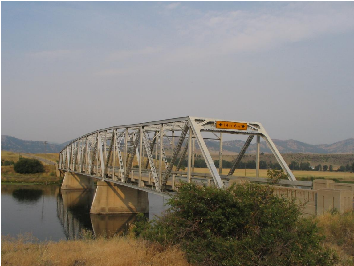
Figure 2. The National Register-listed Missouri River Bridge near Wolf Creek (24LC0131)
