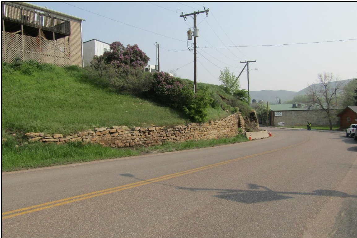
Figure 2. The Belt Retaining Wall (24CA1941) and Secondary 331/Castner Street Segment (24CA1940).
