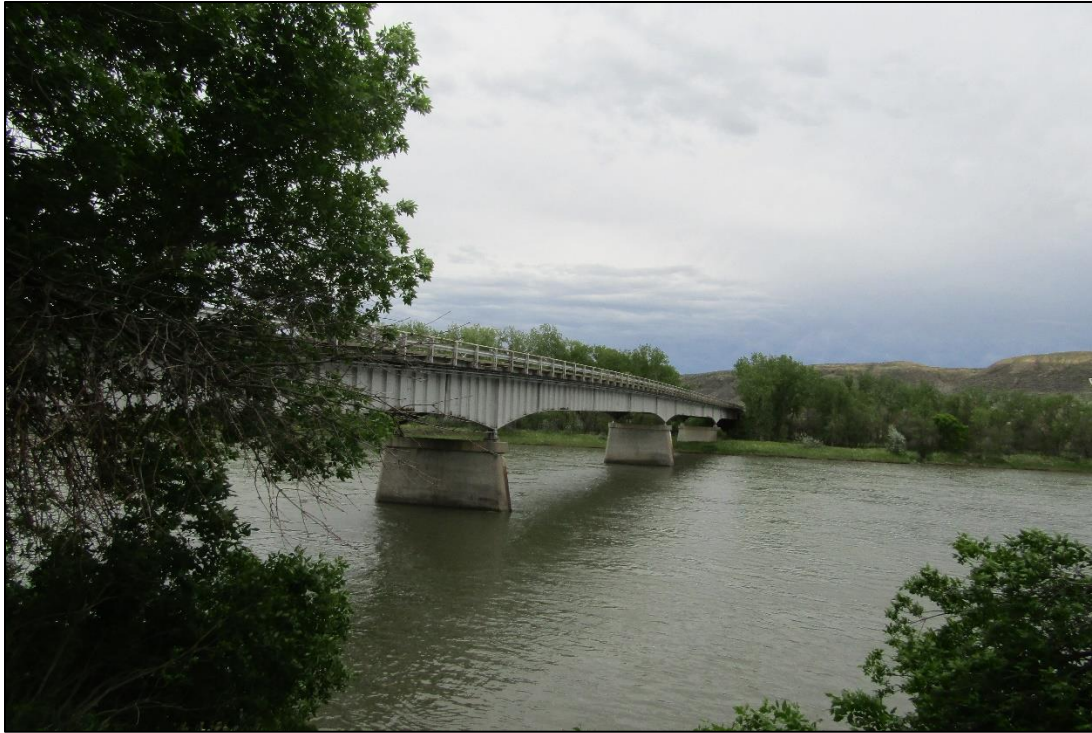
Figure 7. The Missouri River Bridge (24CG1539) at Fort Benton.
