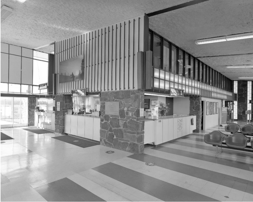
Figure 9. Interior Yellowstone Airport Terminal (24GA1958). HABS/HAER Photograph.
