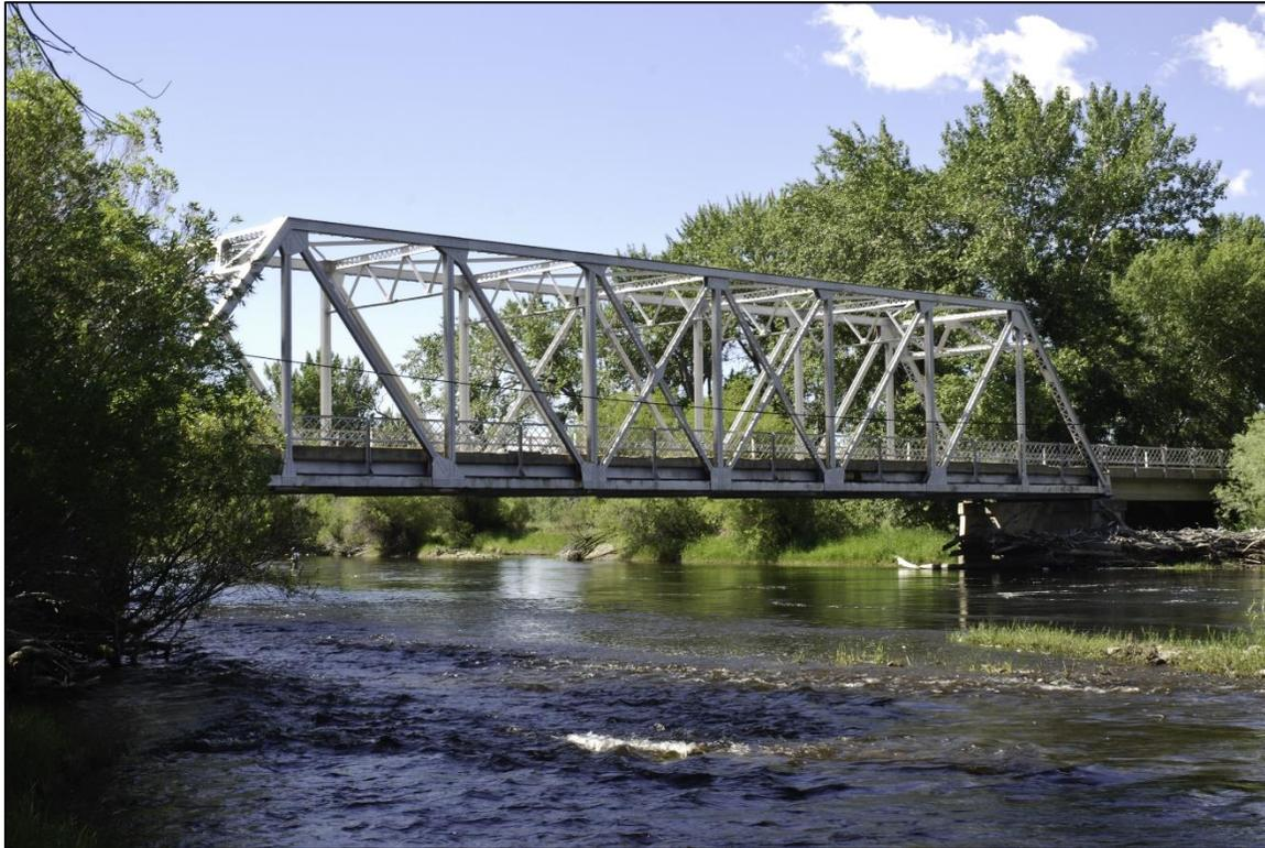
**The Big Hole River/Kalsta Bridge (24BE2061/24MA2094), 22 miles north of Dillon, is an excellent example of a late 1920s highway department-designed through truss bridge.**
