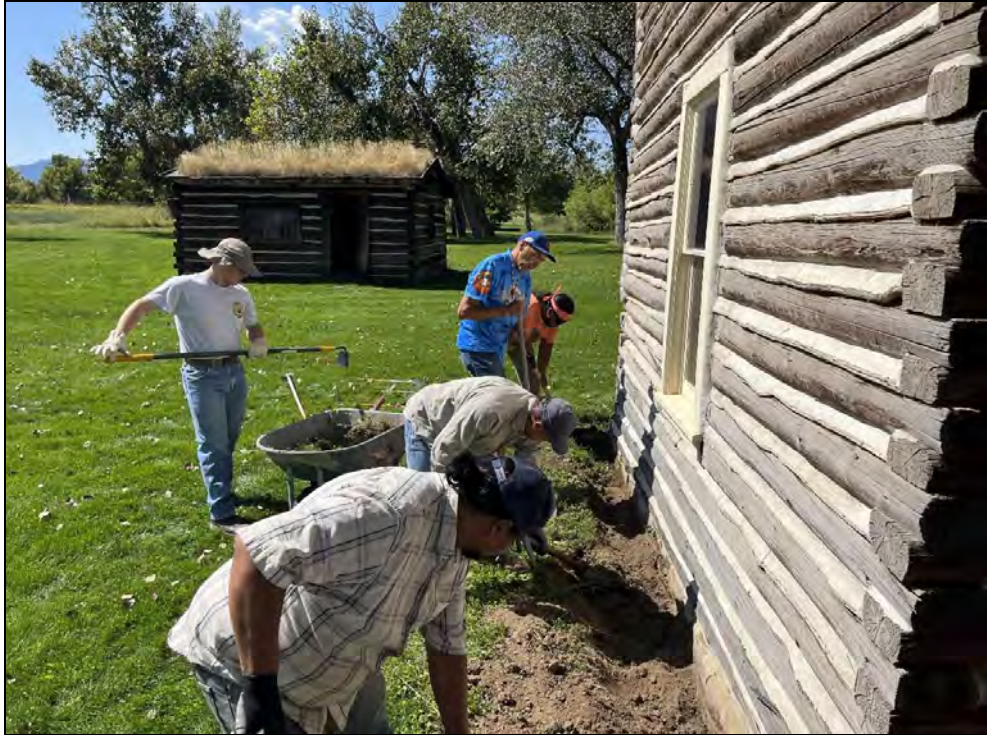
Figure 34. Grading around the Chief's House commences, August 2023.
