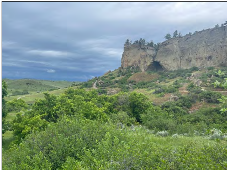
Figure 44. View of Ghost Cave and site of 2021 rockfall taken Summer 2023.
