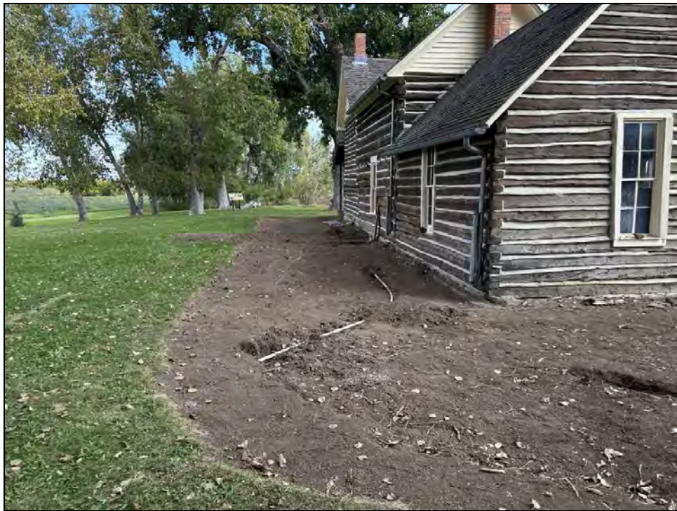
Figure 35. Overview of grading completed around Chief's Store.
