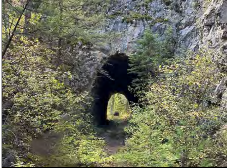
Figure 9. Remains of a wooden railroad trestle and railroad tunnel from the Belt Creek Railway, within Sluice Boxes State Park. Recorded by Preserve Montana in 2022.
