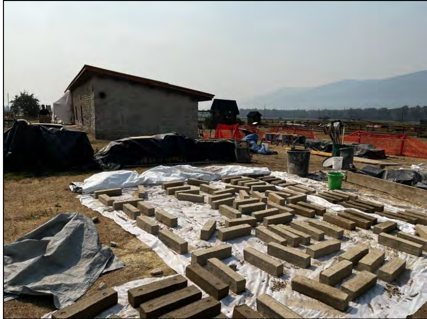
Figure 22: Adobe-making at Fort Owen for the first time in 157 years. The East Barracks (1857), Montana's third-oldest standing structure, is in the background.
