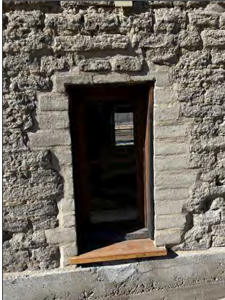
Figure 6. Adobe repairs at Fort Owen.
