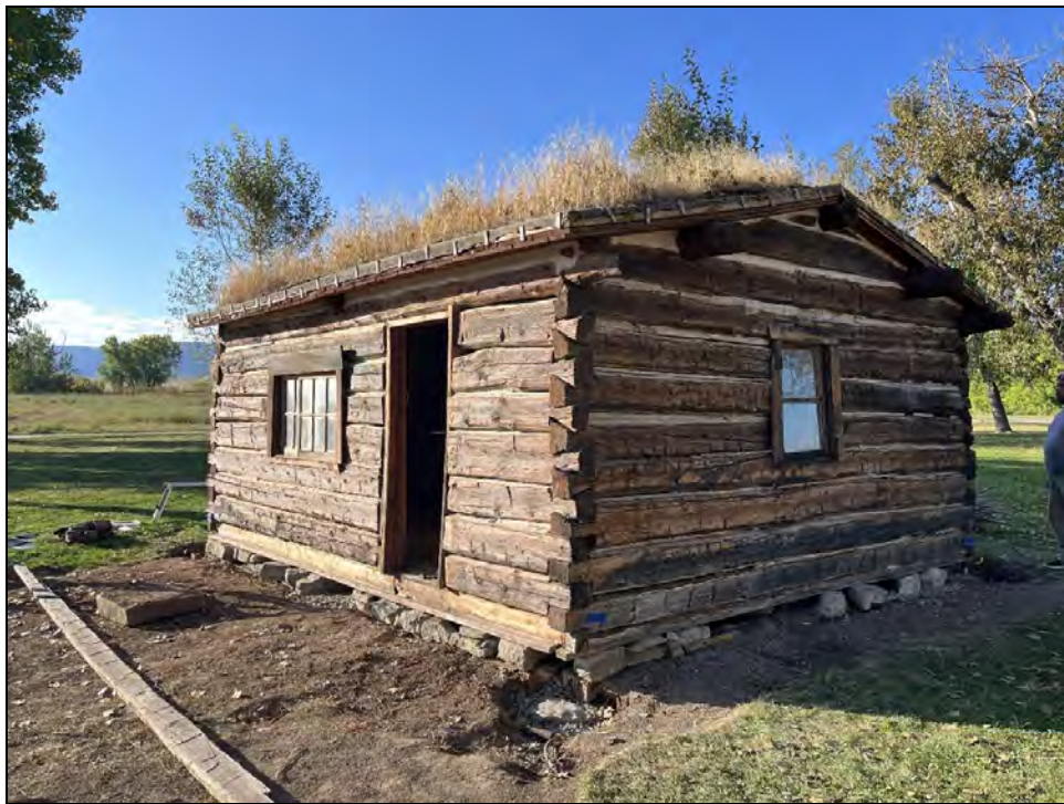
Figure 37. After grading, work begins on foundation repair at the Chief's Store.
