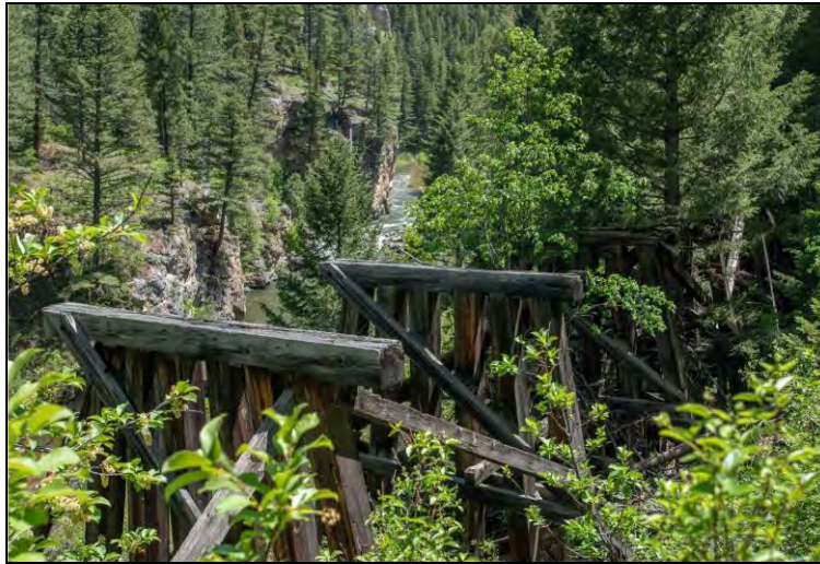
Figure 8. Remains of a wooden railroad trestle from the Belt Creek Railway, within Sluice Boxes State Park. Recorded by Preserve Montana in 2022.
