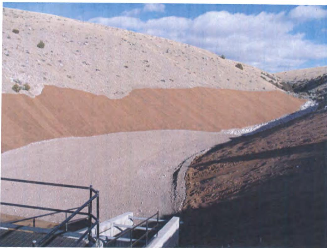
Figure 3. Recently built flood mitigation pond and spillway up Hangman's Gulch at Bannack State Park.
