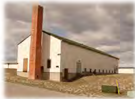
Rear of Post Theater (chimney provided mechanical exhaust venting).
