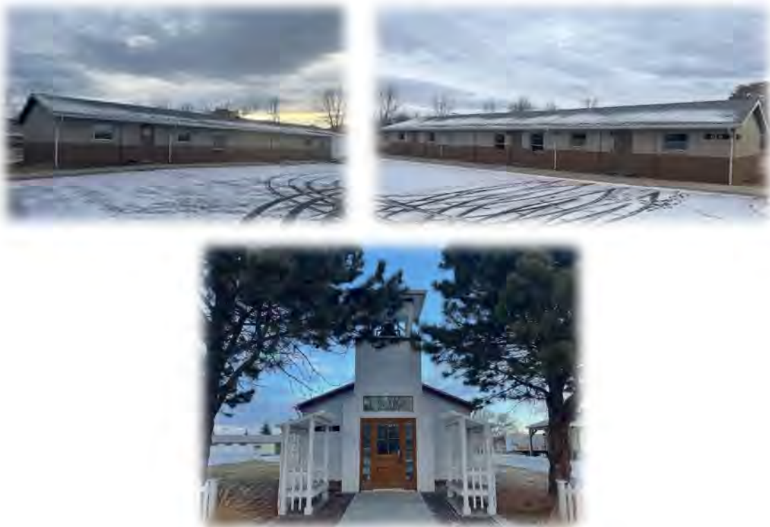
Historic buildings located within the MTARNG Cantonment District that received recent upgrades (clockwise from top left): P-220, P-230, and Chapel.
