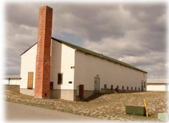
*Rear of Post Theater and chimney that provided mechanical exhaust venting.*
