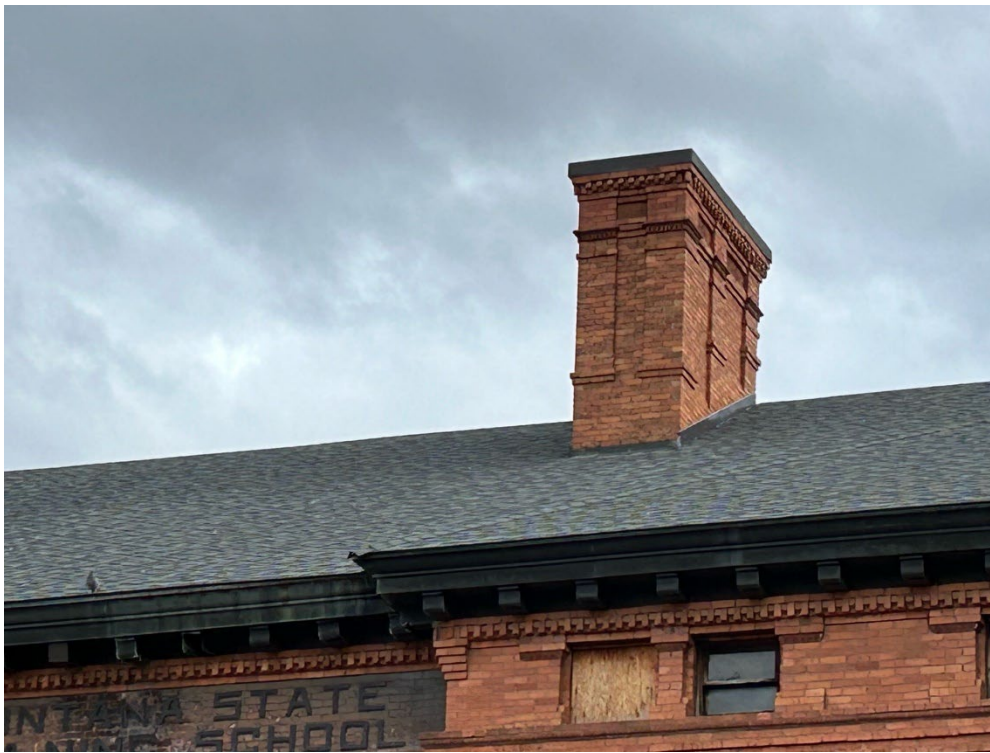
Repaired and reconstructed chimney.
