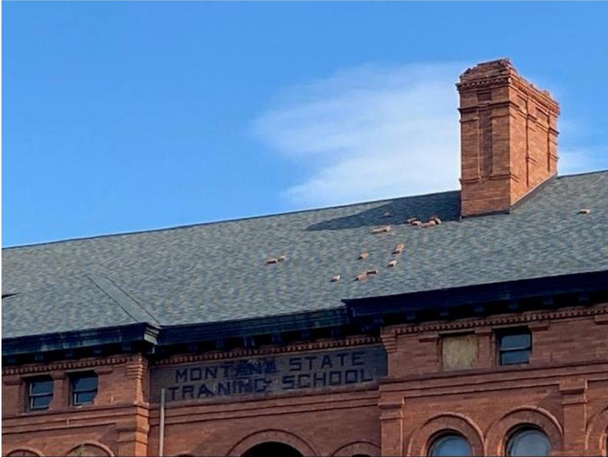
*Damage caused by a windstorm in January, 2021. The chimney cover was blown off and several bricks have been damaged.*
