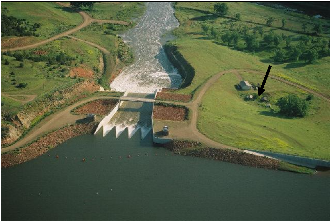
Figure 2: General view of the Lee Homestead (24BH2349: arrow) at the Tongue River Dam
