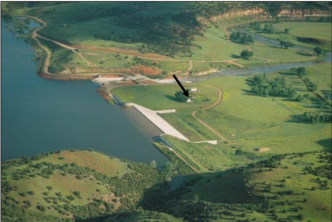
Figure 2: General view of the Lee Homestead (24BH2349: arrow) at the Tongue River Dam.
