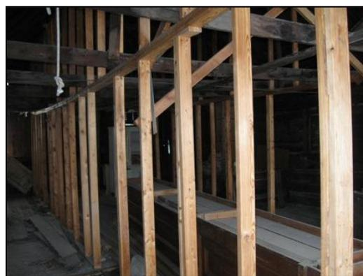
Though the clapboard false-front was preserved in 2009, the interior still retains the same temporary bracing that was placed in 2000 holding the roof up. This building was a display prior to the attempt at full stabilization, and the collections removed from the Prasch have put a strain on already overcrowded storage facilities.
