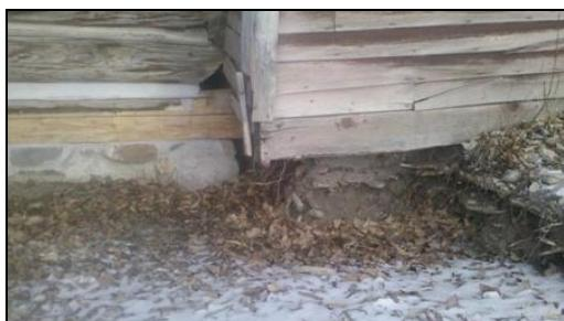
(Left photo) Rear corners of both Greenfront Buildings where they touch: the one on the left (V095) sits securely upon new sill logs and a new foundation, while the one on the right (V094) clearly needs to follow suit.
