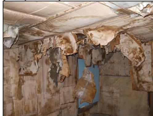
No south interior wall remains in the Cogswell Cabin to shelter it from the elements, and the protective muslin covering what walls are left is clearly beyond repair with weather and water damage. This building is close to being classified as “Failed.”
