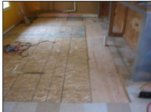
A broken hot water heater damaged the floor, causing the joists to rot. It was removed, and a new floor was put in its place.
