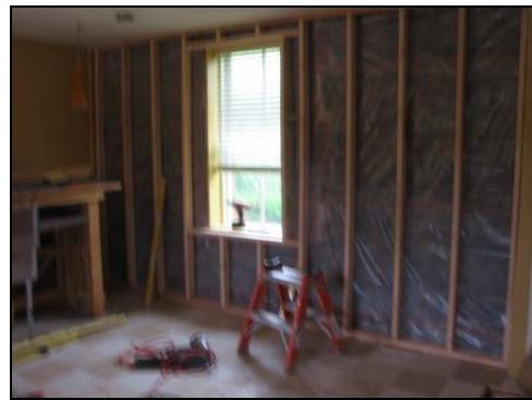
The plastic coating and stud wall before the sheetrock is placed.
