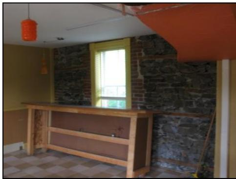
The stone and brick wall was preserved beneath a new wall.
