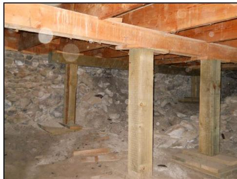
Thought the stabilizing timbers are in good shape, this is a temporary solution to an eminent problem that will eventually arise within all unreinforced stone structures in Virginia City.
