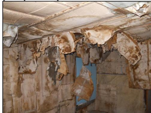
No south interior wall remains in the Coggswell Cabin to shelter it from the elements, and the protective muslin covering what walls are left is clearly beyond repair with weather and water damage. This building is close to being classified as “Failed.”
