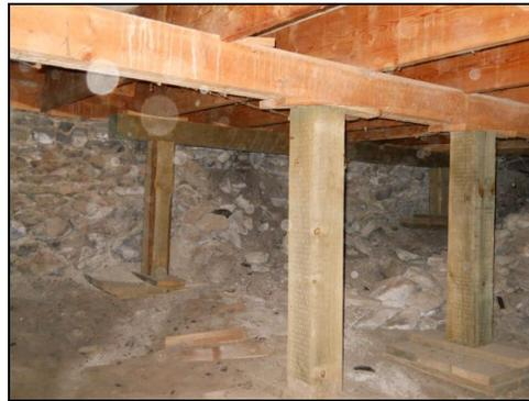
Though the stabilizing timbers are in good shape, this is a temporary solution to an eminent problem that will eventually arise within all unreinforced stone structures in Virginia City.
