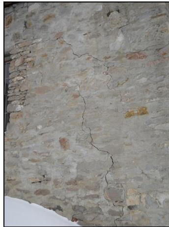
A view of the bowed out interior wall, and the exterior wall of the Montana Post building: Cracks are already appearing on the outside above where the section of stone has failed in the basement.
