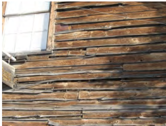
Siding needs repair or replacement
