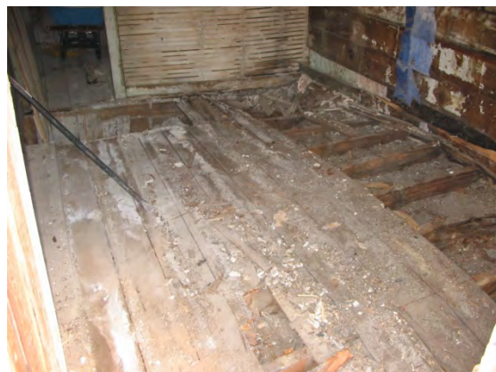
Floor joists throughout the house were critically deteriorated, requiring complete replacement
