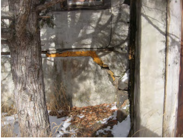
Cracks in foundation need repair
