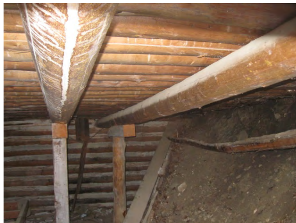
New logs and foundation will need to be constructed
