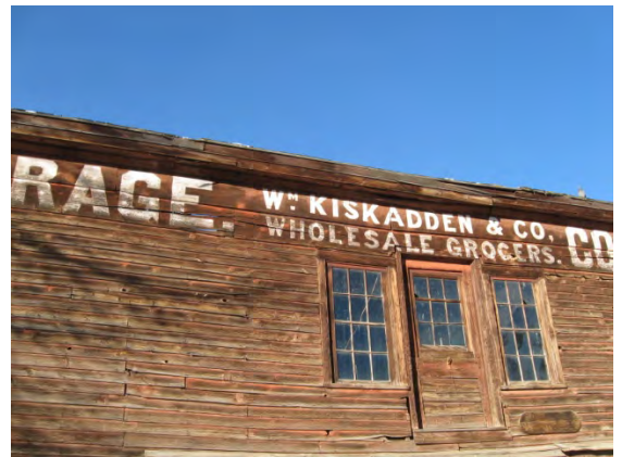
False front is starting to fail on the top. Rotten wood will need to be removed and then framing and planks installed. Siding needs to be repaired or replaced.
