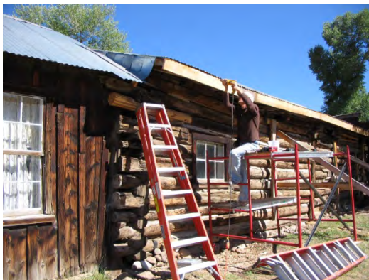
Replacement of rotten fascia boards, log splices and Dutchmen repair was completed to select areas.
