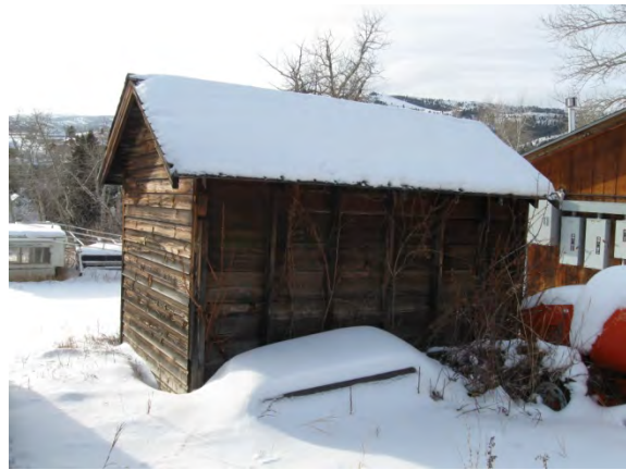
Needs siding repair and replacement
