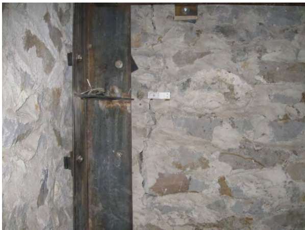
Repoint the cracks
