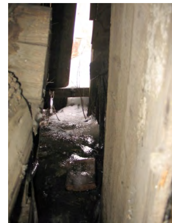
Narrow alleyway between the McGovern and Strasburger stores had long provided a pathway for water and ice to intrude into the interior spaces of both buildings
