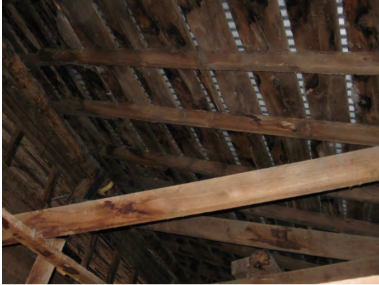
Metal roofing & sheathing will have to be removed to try and pull the deflection out
