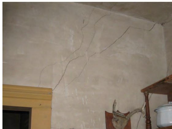
Cracked plaster
