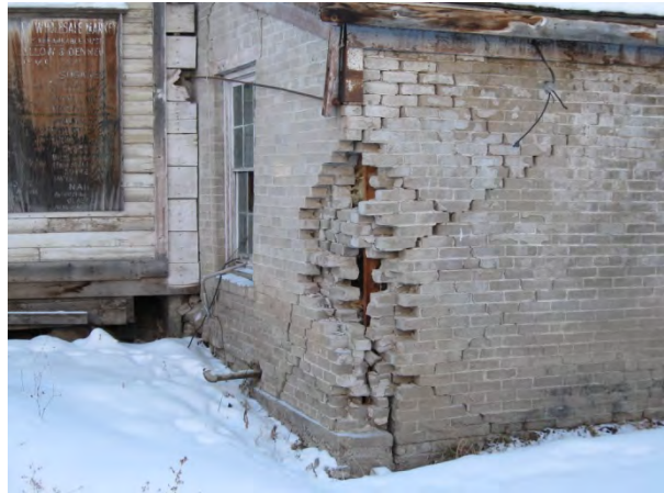
Failed brick on NE corner
