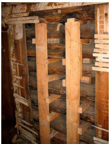
Portions of the damaged historic lath and select vertical planks are removed to provide access to the original splice point of the log members and allow for the installation of a vertical support and cleat system
