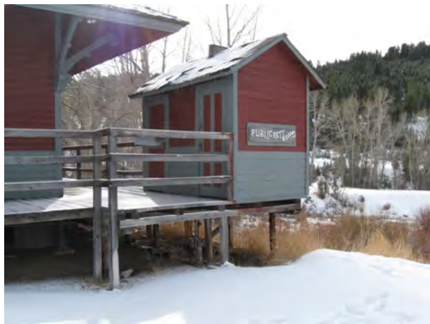
Bathrooms sit on corner of the back porch with little structural support
