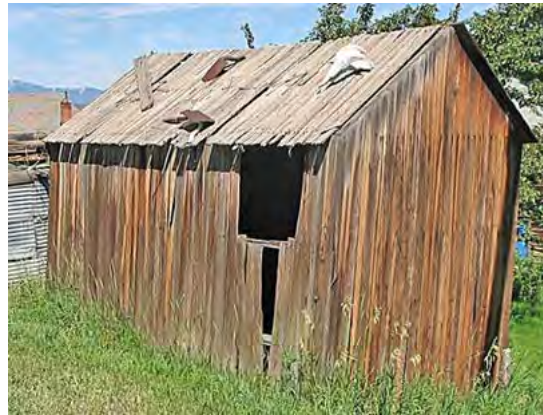
Plank boards on Hickman Shed are deteriorating and need to be replaced
