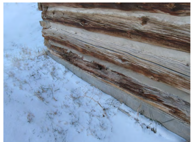
Logs showing signs of deterioration
