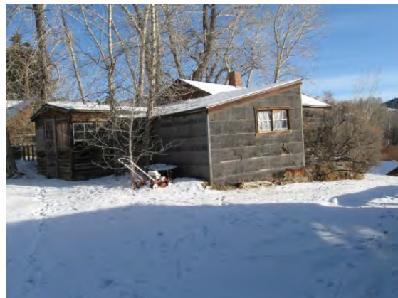
Mutt Dixon House (Costume Shack) – siding needs to be repaired or replaced. Needs door and window preservation
