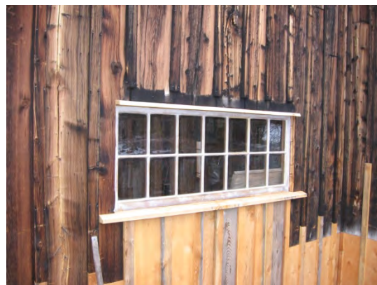
After- board and batten siding is replaced and the old broken window and frame is replaced with a fixed window
