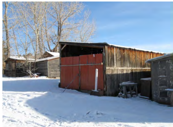
Scenery Shed – Needs foundation and siding applied to protect from further damage
