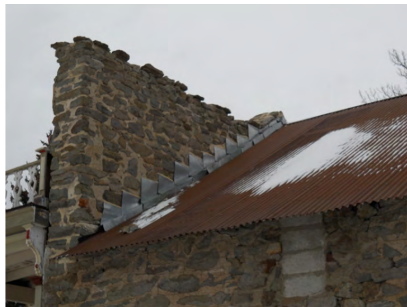
Back side of façade with failing capstones
