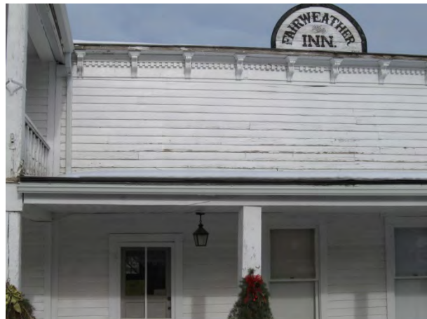
Siding needs repair and replacement along with painting
