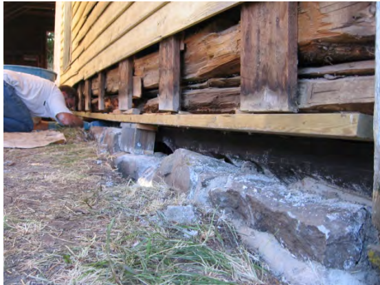
Original stone foundation was discovered on east side. The original foundation was then reset and re-pointed
