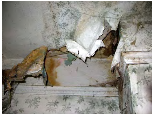
Above – Water damaged lath and plaster is assessed to provide an access point to the attic.
