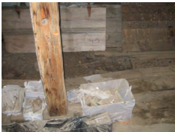
Floor boards need to be repaired or replaced
