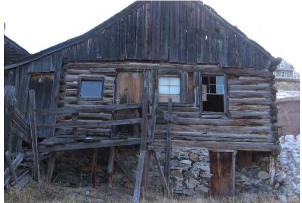
Before preservation on sill log and foundation
