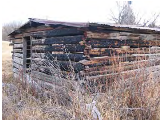
Before – Fire damage to northwest corner, weathered logs, and overgrowth
