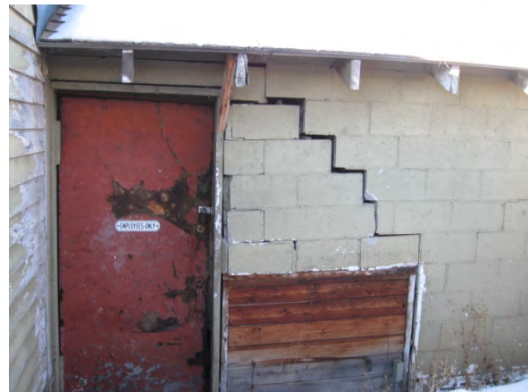
Cracked and failing cmu wall of boiler room
