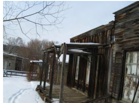
False fronts need to be stabilized and repaired throughout all the cabins
