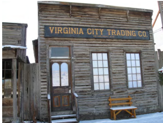
Needs some siding repair and to be oiled
