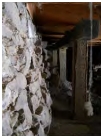
A view of the bowed out interior wall
