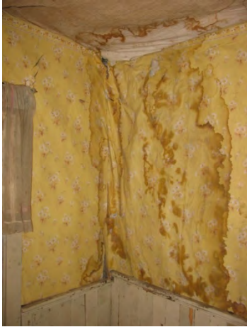
Water damage to the eastern wall and ceiling in kitchen and side room
