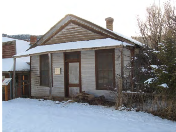
The cabin needs a new foundation, roofing and framing stabilization and a new roof
