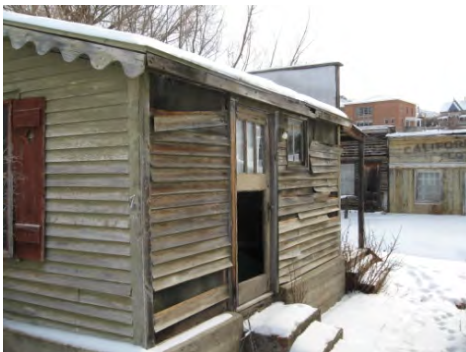
Entire row of cabins needs siding, window, and door repairs.
