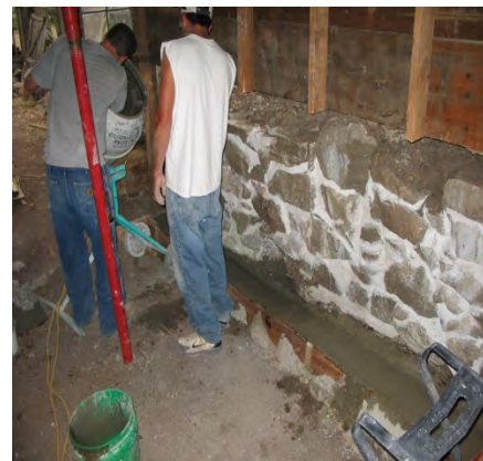
After – eastern wall re-pointed and a new footing is poured to support a new sill and wall studs in the mud room
