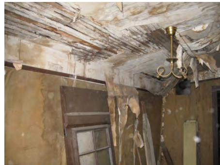
Damaged lathe and plaster work needs to be repaired on ceiling
