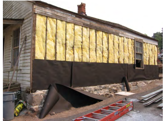
Clapboard siding removed in order to install fiberglass insulation and a felt barrier
