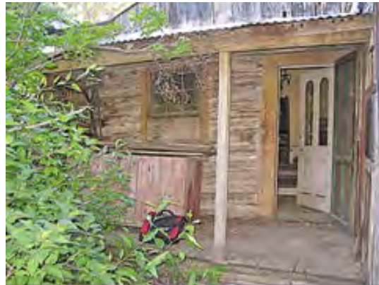
Back porch – Foundation work needed
