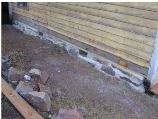
After- east wall with siding replaced and vents installed to provide proper ventilation under the floor space
