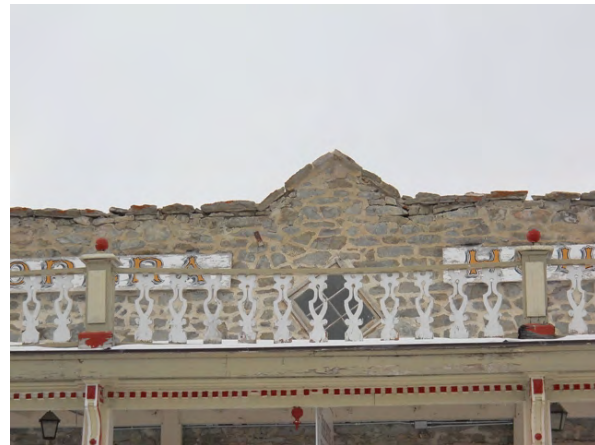
Failing capstones and crumbling mortar on façade
