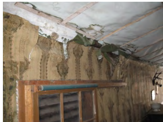
Interior damage from leaking roof
