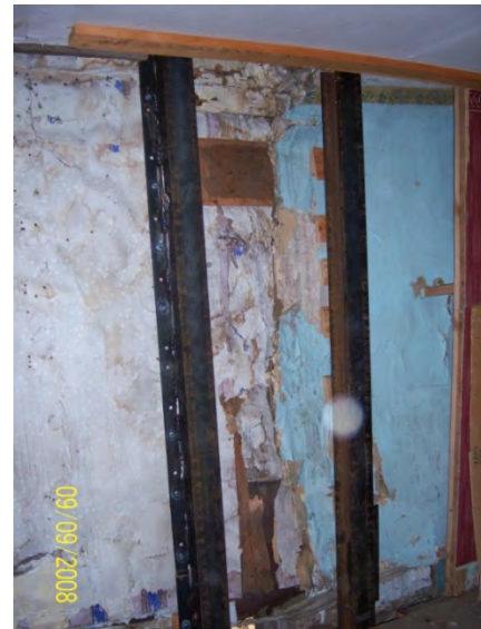
Steel bracing installed on east wall
