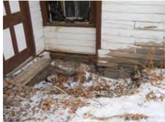
Failed foundation
