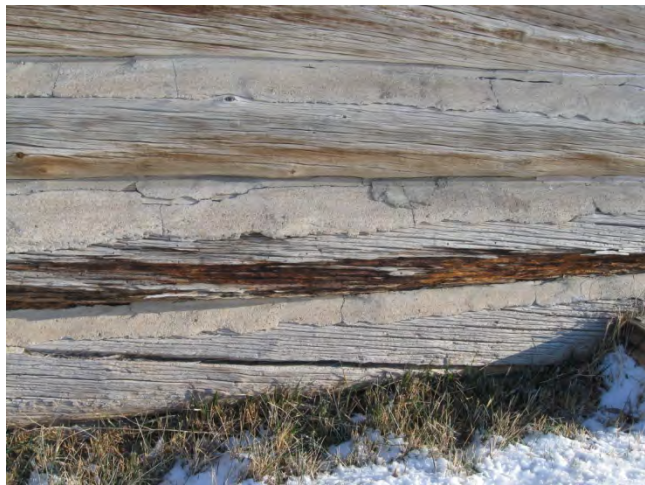
Logs showing signs of deterioration
