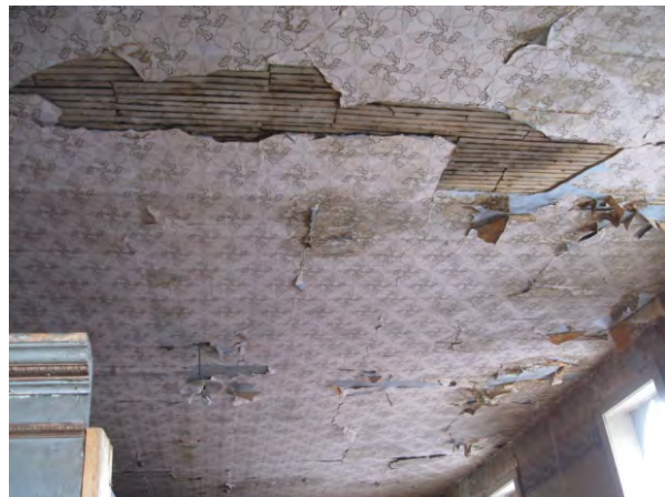
Lathe and plaster ceiling failing due to roof leaking
