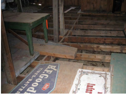
Floor is deflecting and in need of stabilization
