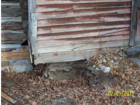
Preserved restaurant side on the left has new foundation and sill logs compared to the right side with no foundation and rotted sill logs
