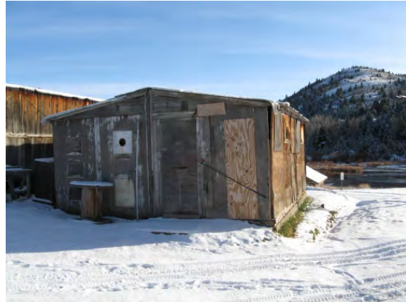
Opera House Shop – Needs to be stabilized and siding needs to be applied to protect the plywood sheeting from further damage. Needs door and window preservation.
