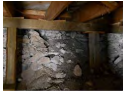
Stabilizing timbers are a temporary solution for this unreinforced wall
