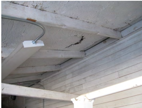
Ceiling damage from a leaking roof
