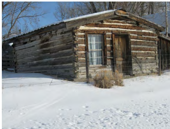
Finney Summer Kitchen has rotting logs that need to be replaced
