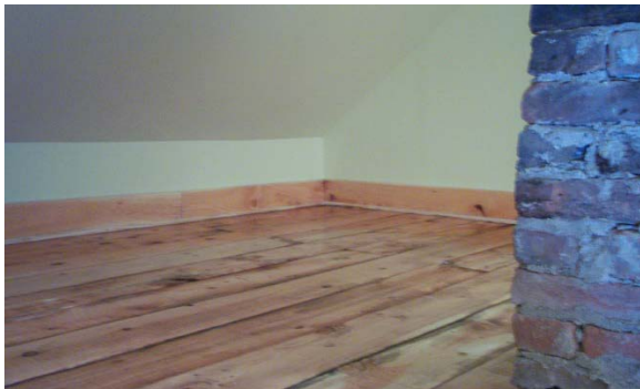
After – finished floor complete with baseboard trim in the loft area
