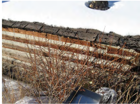
Rotten sill logs need to be replaced
