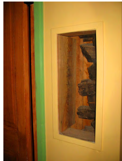
An exposure window was installed in the created door way to the residences reveals the original, southwest log corner of the Corbett wing
