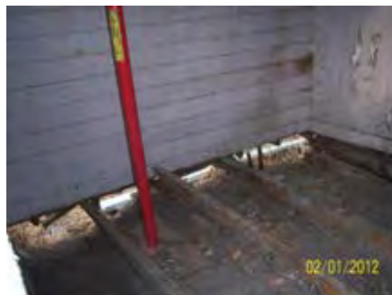
The interior of an addition to the Hickman House sitting on floor joists exposed to the element
