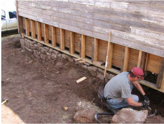
Rotten ends were sistered with new studs around the west and southwest walls of the Daemes House for added strength and support of the original material.
