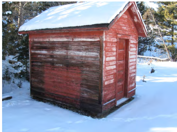
Needs to be jacked up and timbers placed underneath
