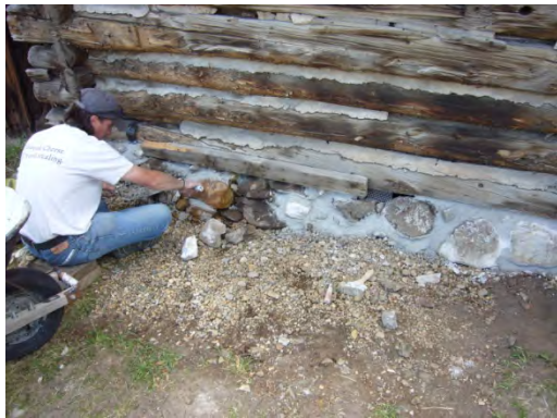
An improved foundation system and a drainage system was installed for the west wall.
