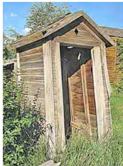
Outhouse located behind the store needs to be jacked up stabilized with timber placed underneath it
