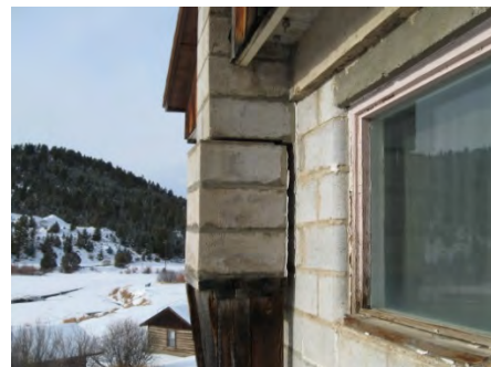
Chimney on the south side of building needs to be stabilized
