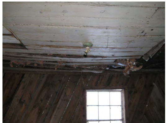
Daylight shows through a wall, along with missing ceiling boards
