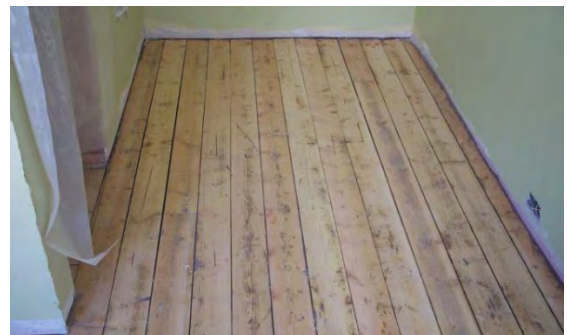
After - Original flooring put back in sanded about to get a finish coat
