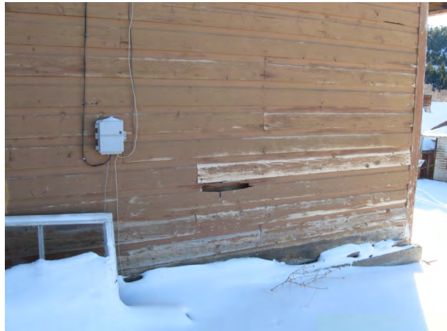
Siding needs to be repaired or replaced
