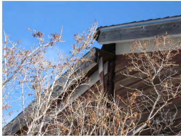
Roof line has separated
