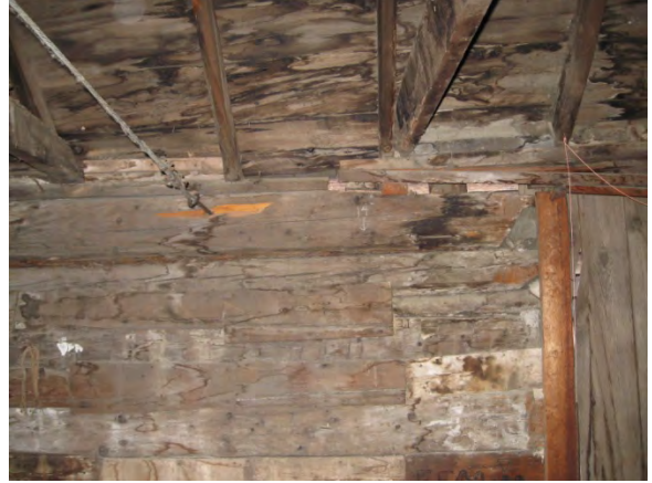
Water damaged to ceiling and walls left deteriorating wall boards.
