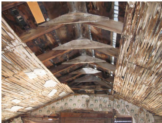
Entire roof framing needs to have new framing sistered to it
