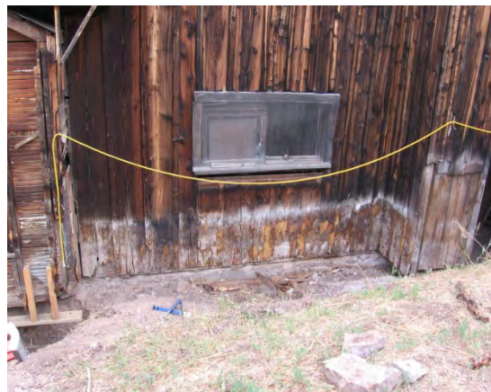
Before - False concrete foundation is removed from the south side of Corbett house which then reveals rotten boards.
