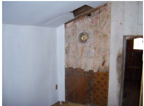
After- 3 rd room walls complete and plexiglass over northern wall to protect historic wall coverings
