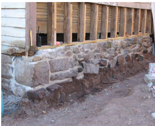
After – northwest corner after re-pointing and new concrete grade beam
