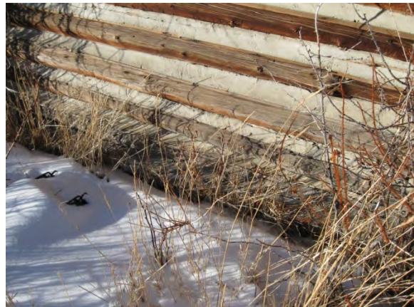
Needs to be excavated for foundation
