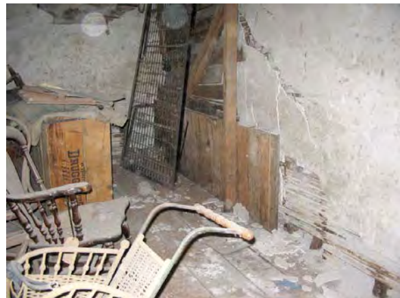
Interior damage to historic lathe and plaster
