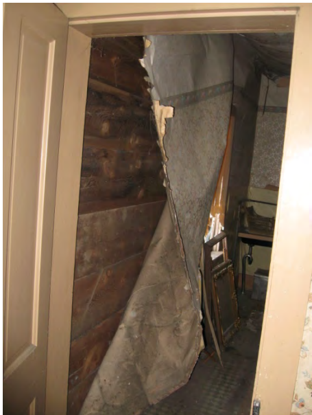
Failing wall coverings
