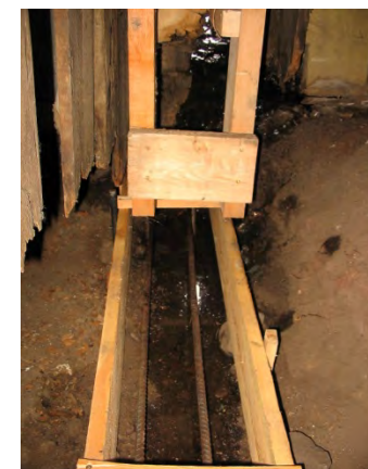
A new footing system was created to stabilize the eastern log wall and to assist in diverting moisture from entering the alleyway
