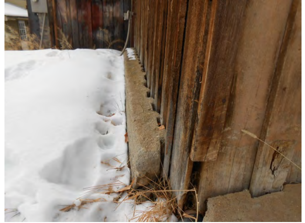
Foundation and sill work needed
