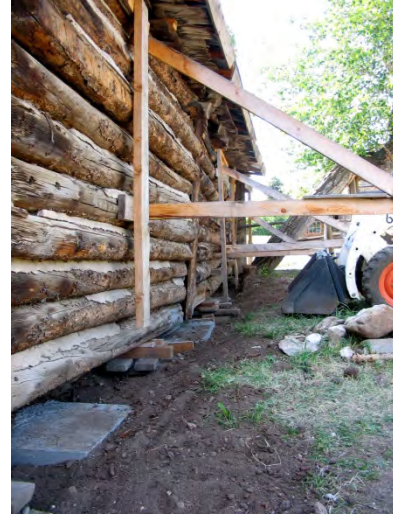
Stabilization treatments were done to the building including digging five footings
