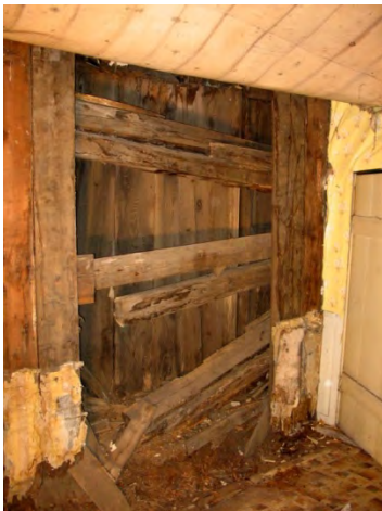
Planks from the eastern wall were removed to reveal extent of damage
