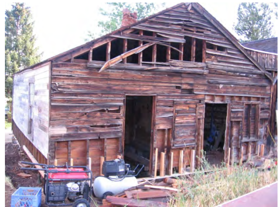
Before- critically deteriorated siding along the south façade was removed for insulation to be installed and replacement of siding
