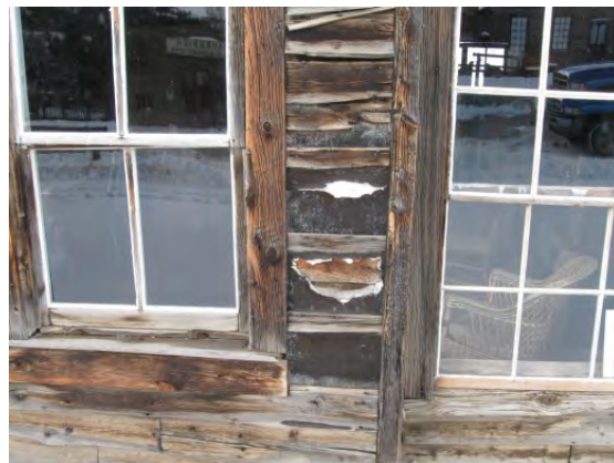
Deteriorated lap siding needs to be replaced
