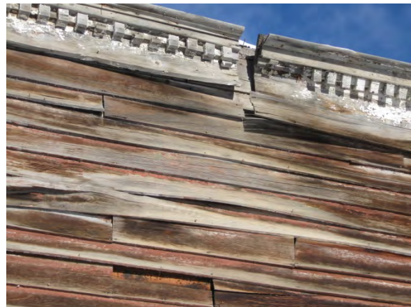
Decorative cornice pieces failing and separating from building
