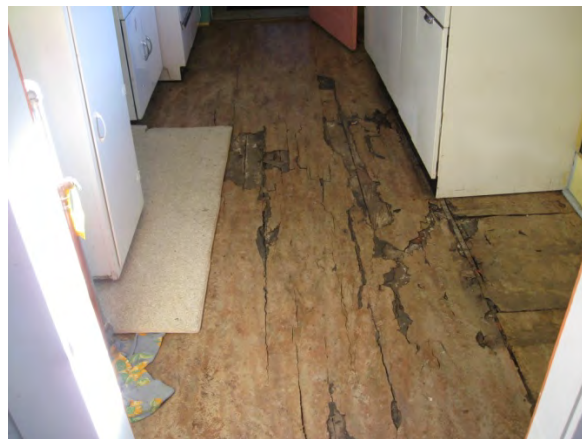
Floors need to be removed and replaced throughout the house
