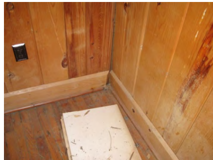
SW corner of one unit is sinking causing walls to separate
