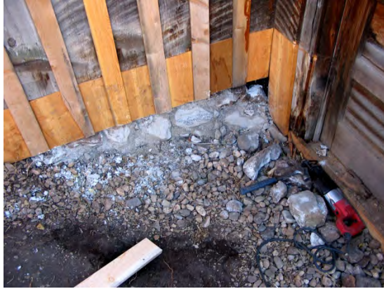
Deteriorated building material which was damaged from ground water issues and an elevated grade was replaced. A short French drain is employed to direct water away from an inside corner.
