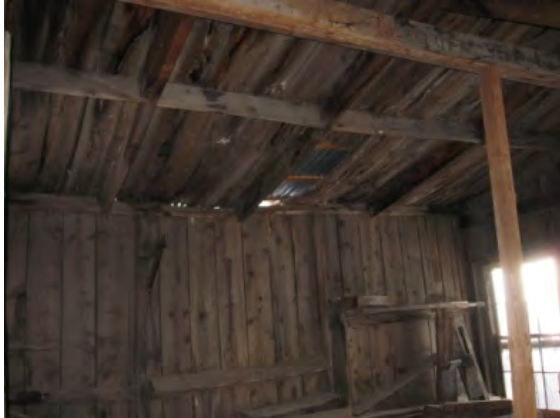
Roof boards need to be repaired or replaced
