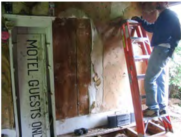
Before- Wall paper falling off, planks exposed
