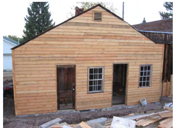
After- siding was replaced and attic vent and new windows have been constructed and installed
