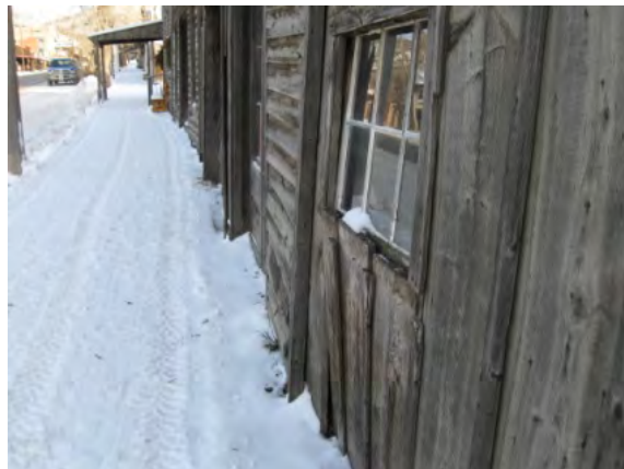
Front wall is starting to buckle out which needs to be stabilized and repaired
