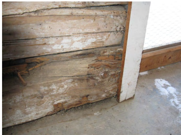
Logs showing sign of deterioration
