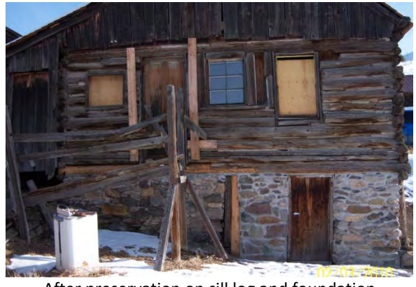
After preservation on sill log and foundation
