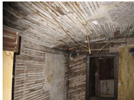
Damaged lathe and plaster work needs to be repaired on walls
