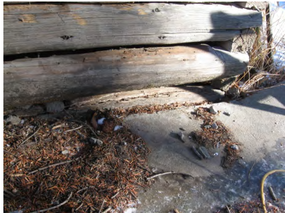
Sill logs are rotting around entire cabin. New foundation is needed
