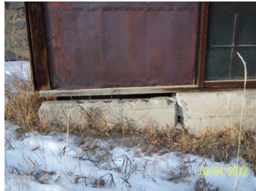
Structural issues with the foundation
