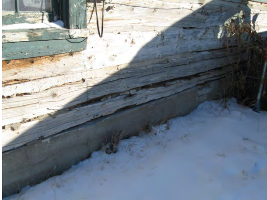
Rotten sill logs on the West side of house needs to be replaced
