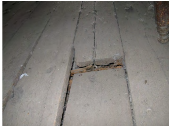
Floor joists are rotting making the floor boards loose and unsafe to walk on
