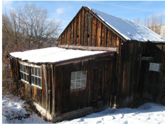
Cabbage Patch Barn. Entire Cabbage Patch complex needs to be jacked up, stabilized and sill logs and plates replaced.
