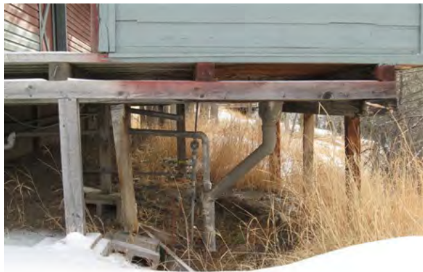
Bathrooms sit on corner of the back porch with little structural support
