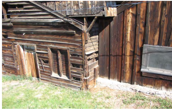
Before – South side of houses – Note the grade level and the “Bovey Backfill” false foundation. Major excavation was needed to expose the foundation around the entire structure
