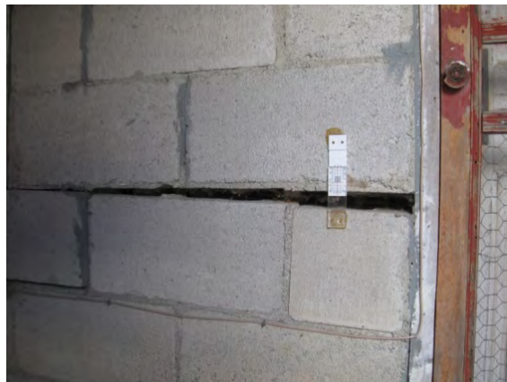
Crack monitor placed on rear façade shows growing displacement at an alarming rate
