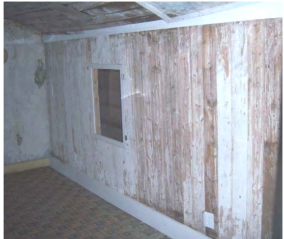
After- Finished look of western wall. Plexiglass window installed to see logs
