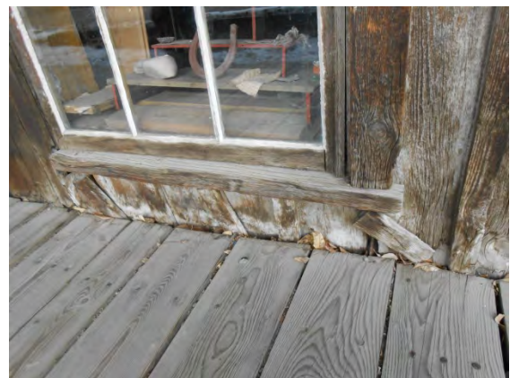
Foundation work needed on front of building
