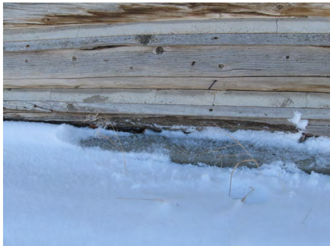
Sill logs are rotting and need to be replaced along with the foundation
