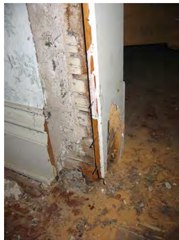
The facing section of wood trim is removed from the opening in the stone portion to gauge the extent of Carpenter ant activity. Damage is visible on the remaining portion of trim where it meets the floor.
