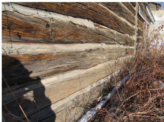
South side logs starting to show signs of deterioration
