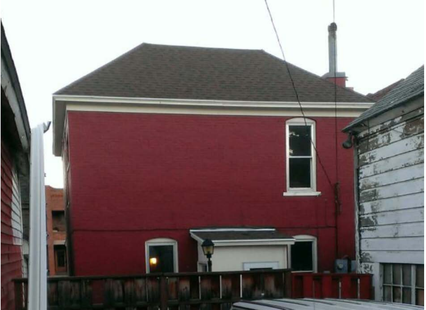
John and Armeta Duncan Residence Rear Elevation, Facing: S Anthony Wood, June 26, 2015
