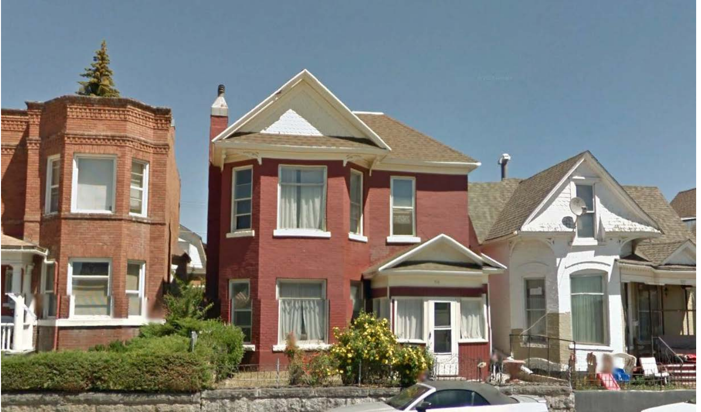
John and Armeta Duncan Residence South Façade, Facing: N Google Earth, 2014
